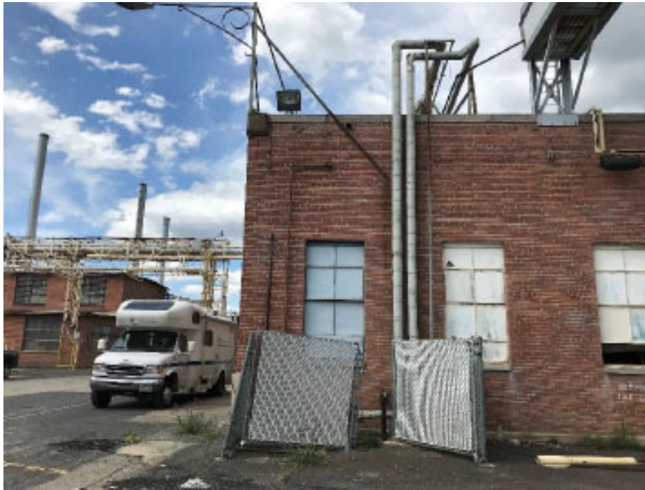
Figure 5: Asbestos containing pipe wrap found in a deteriorated condition and falling to the ground in several locations.
