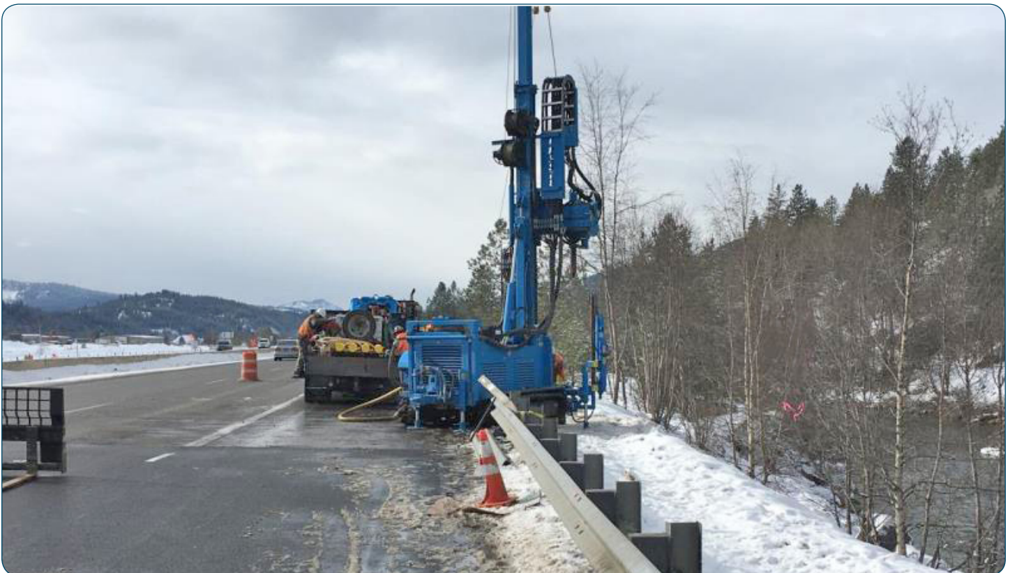
Installing monitoring wells north of I-90.
