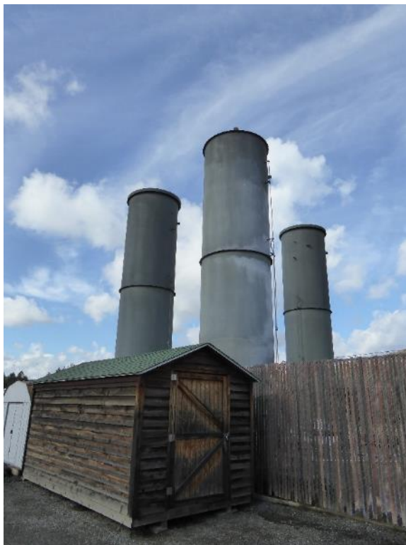
Three landfill gas flares on site; only one operates due to low gas volumes.
