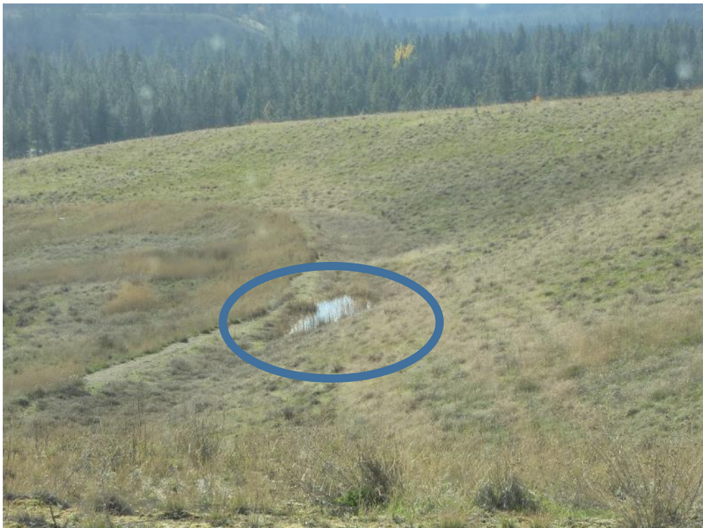
Ponding on the capped landfill.
