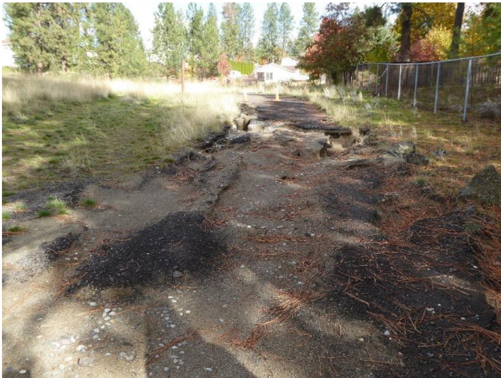
Damage to the access road at the top of the washout area.
