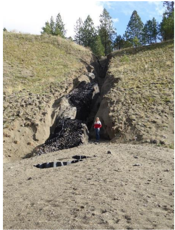
Two views of the washout area in the outer edge of the landfill buffer zone. Left image shows material and geowebbing carried to the bottom by the water flow. Right image shows site RPM standing in washout for scale.
