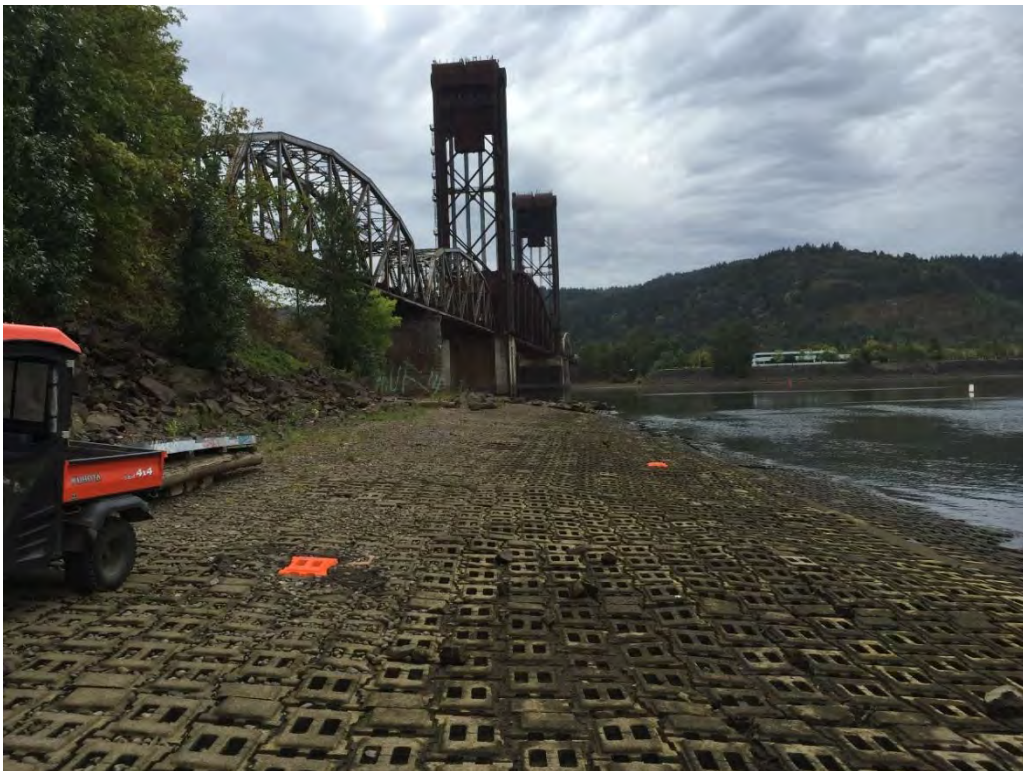
Photograph 5 – Willamette Cove sediment cap ACB blocks (bright orange) replaced following September 2015 organoclay sampling.
