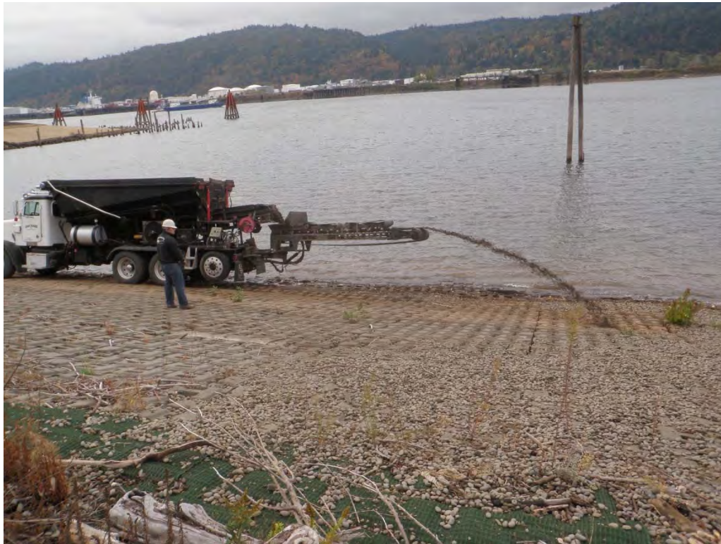
Photograph 10 – ACB gravel replacement in 2012.
