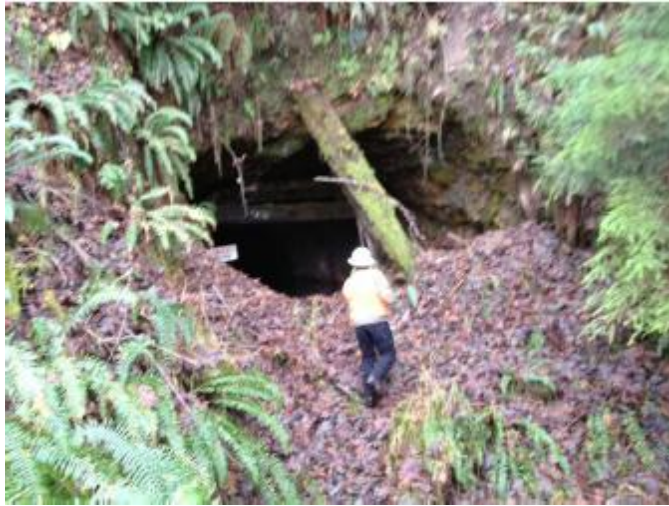
Photo 1. One of the adits found during the site walk of the mine. An adit is a passage that leads into a mine or provides a passage for water to drain from the mine.
