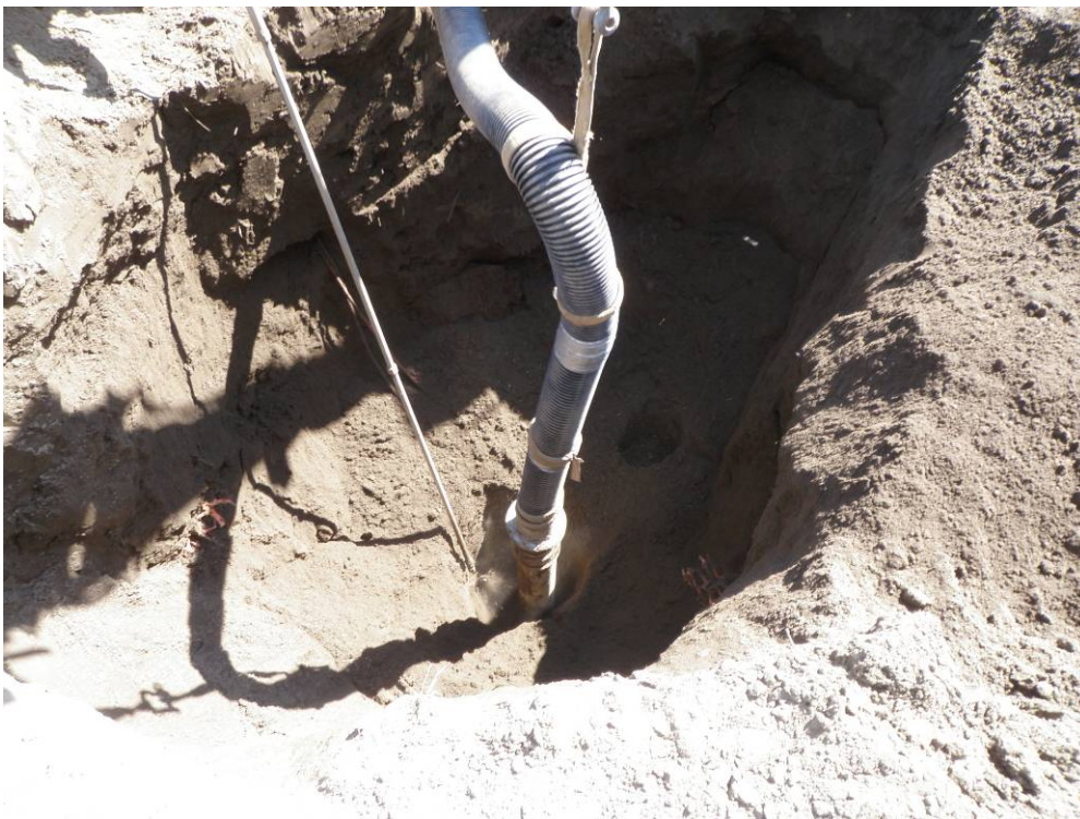
Photograph 8 – Pot holing to 25 feet depth.
