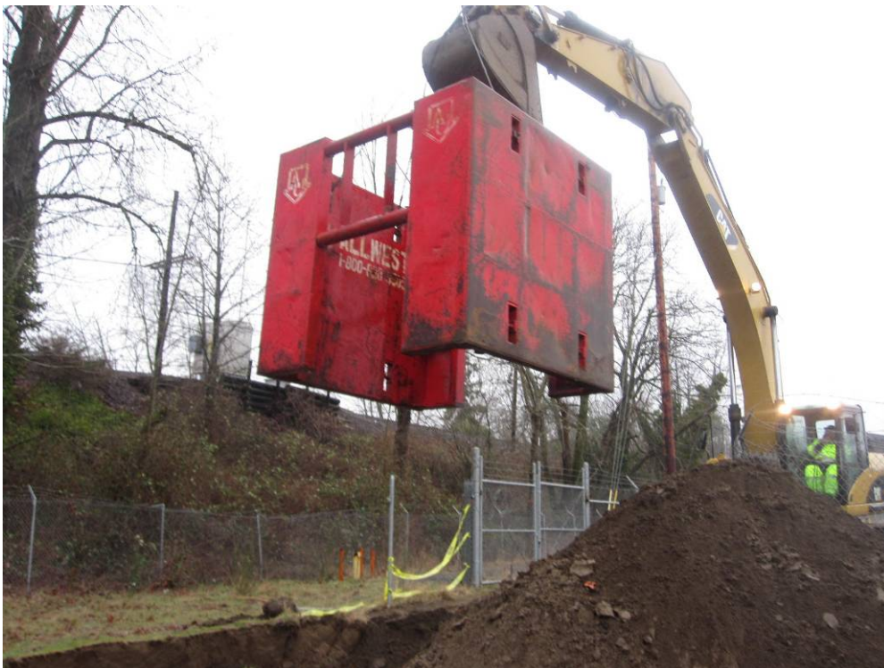
Photograph 4 – Shoring used to stabilize loose sands. Photograph is facing north.
