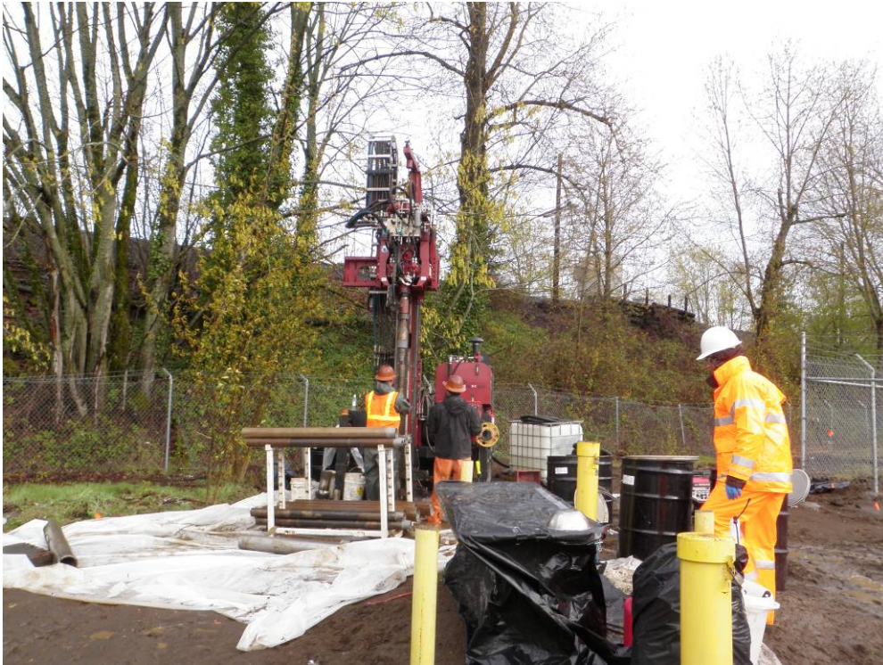
Photograph 11 – Sonic soil boring SC0111. Photograph facing north.
