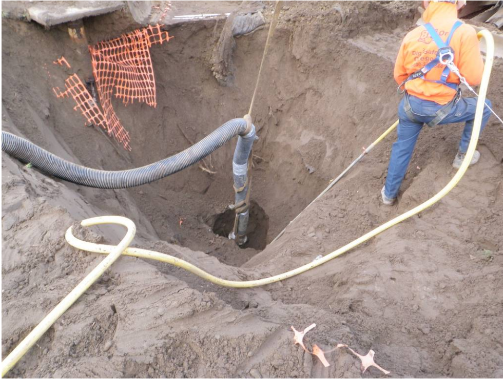
Photograph 9 – Pot holing for sewer lines near MW-20i. Photograph facing northwest.
