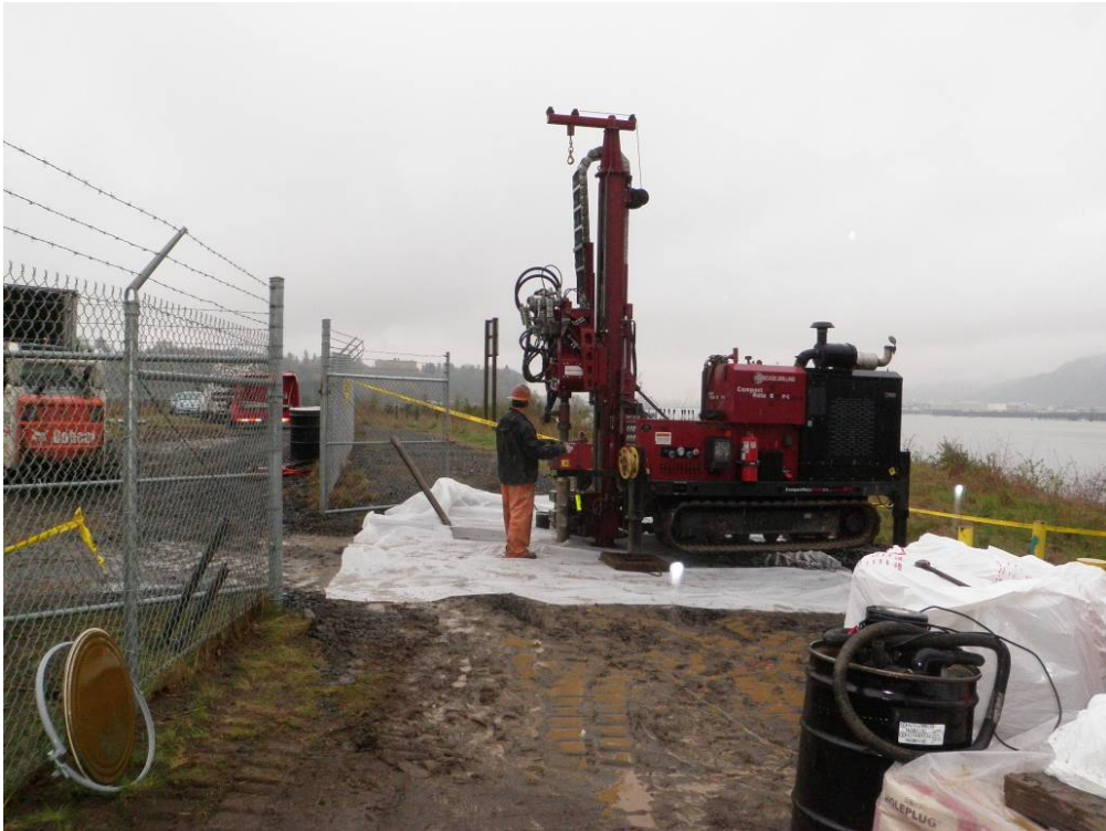
Photograph 13 – Sonic soil boring SC0411. Photograph facing north.
