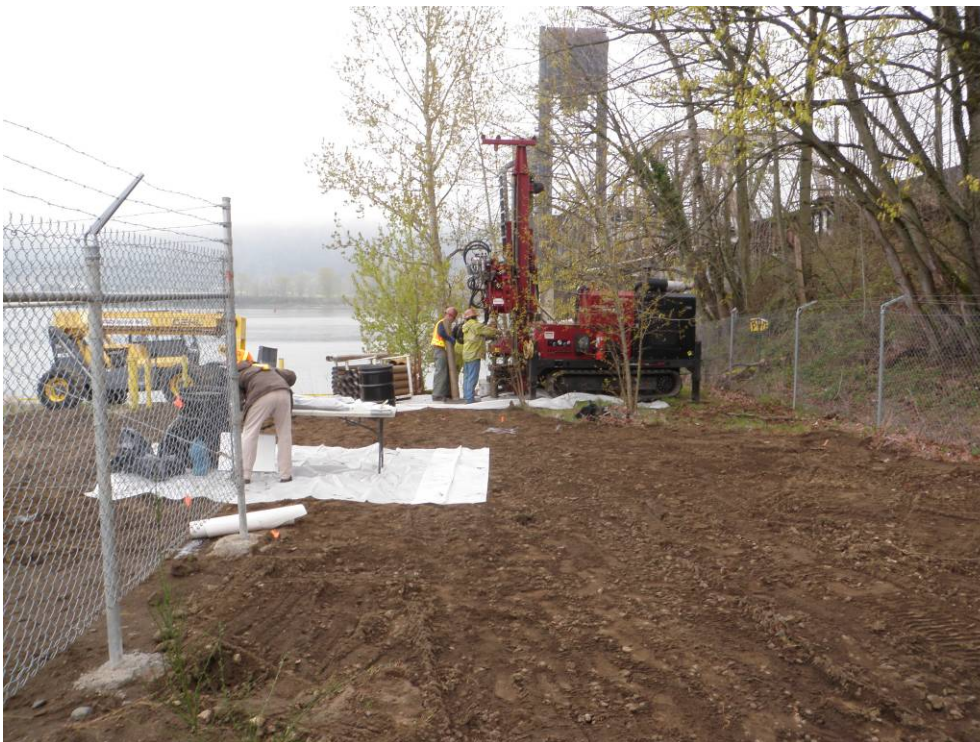
Photograph 10 – Sonic soil boring SC0211. Photograph facing west.
