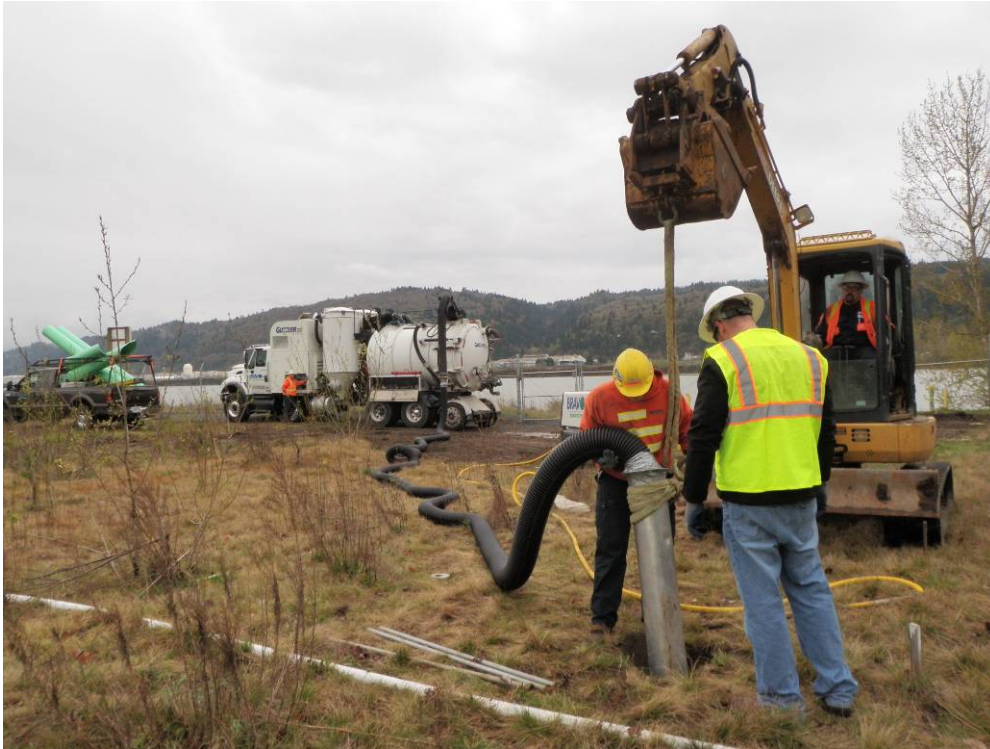
Photograph 5 – Pot holing 100 feet upland from MW-20i. Photograph facing southwest.
