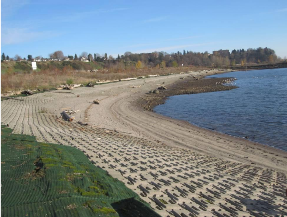
Photograph 3 – Erosion matting intact after high water. Vegetation growing back on matting (December 2011). Photograph taken looking southeast.
