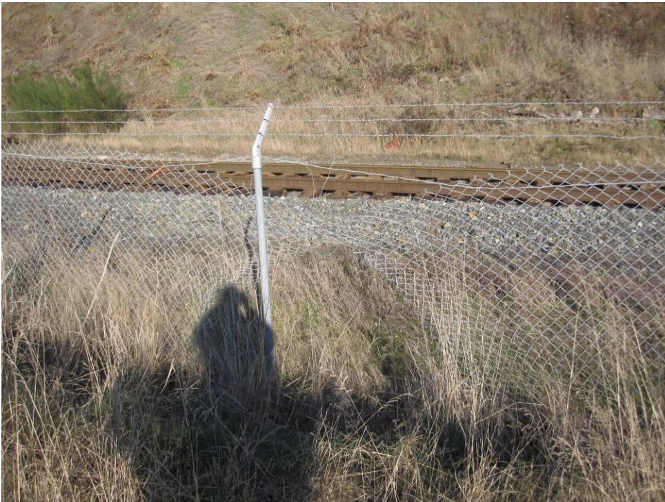
Photograph 14 – Fence damage by trespassers. Photograph taken looking northeast (December 2011).
