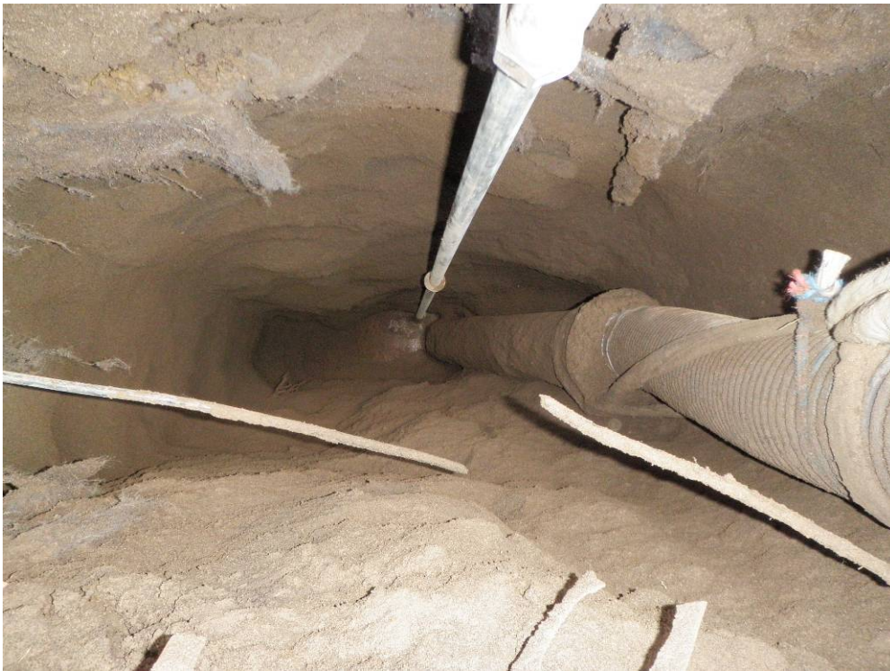
Photograph 6 – Sewer line at 12 feet depth.
