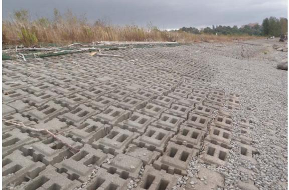
Photograph 2 – Comparison of ACB with and without habitat gravel to fill voids. Photograph taken facing east.
