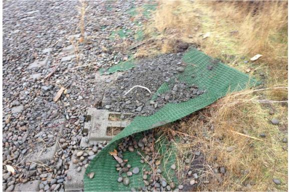
Photograph 6 – Void space under TRM filled in with crushed rock before TRM was re-secured to ACB. Photograph taken facing north.
