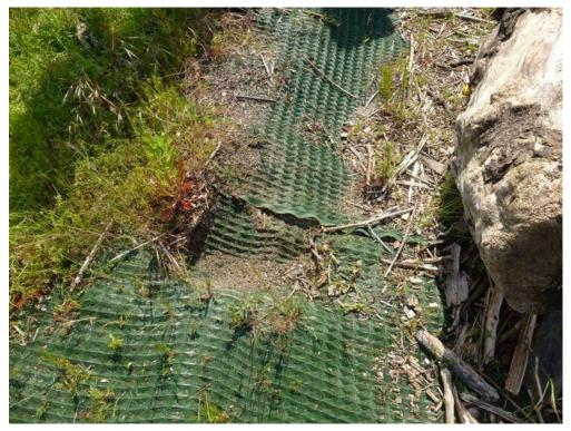
Photograph 2 - Soil erosion and damage to the TRM.
