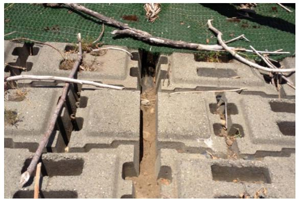
Photograph 4 – Soil can be observed eroding from under the TRM into ACB. Photograph taken facing northwest.
