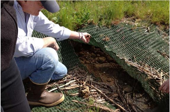
Photograph 5 – Void space under the TRM where soil has eroded away. Photograph taken facing east.
