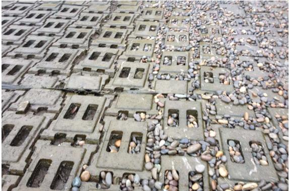
Photograph 1 – Comparison of ACB with and without habitat gravel to fill voids. Photograph taken facing northeast in Willamette Cove.
