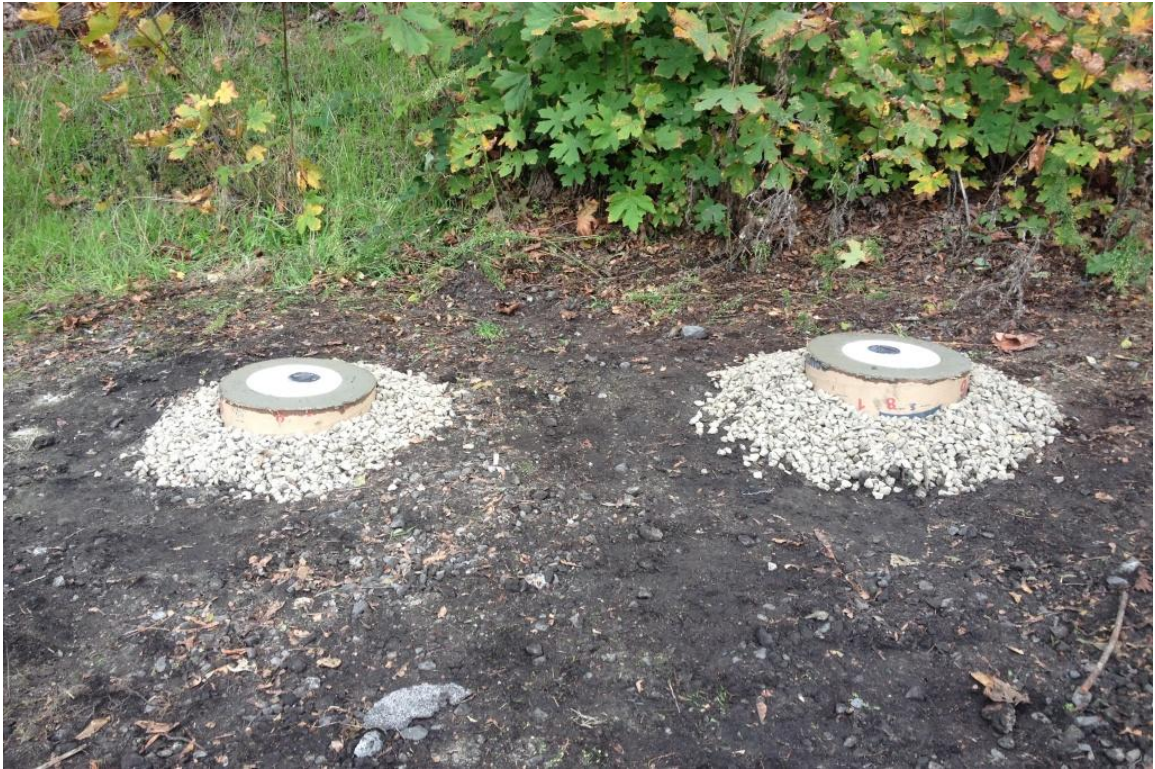
Photograph 7 – Two of the three MW-58 wells in the well cluster completed.
