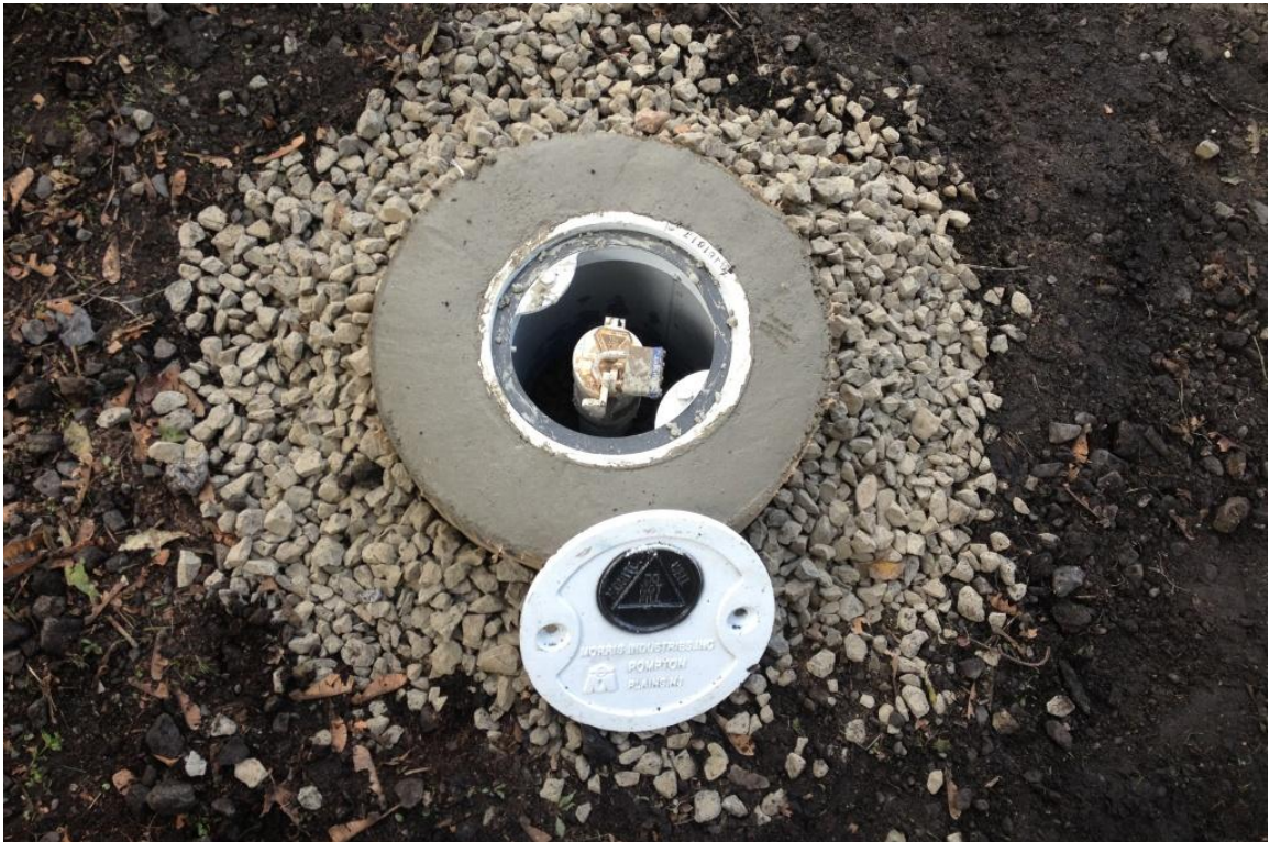
Photograph 6 – MW-58 well cluster repairs completed without making modifications to the existing well casing heights.
