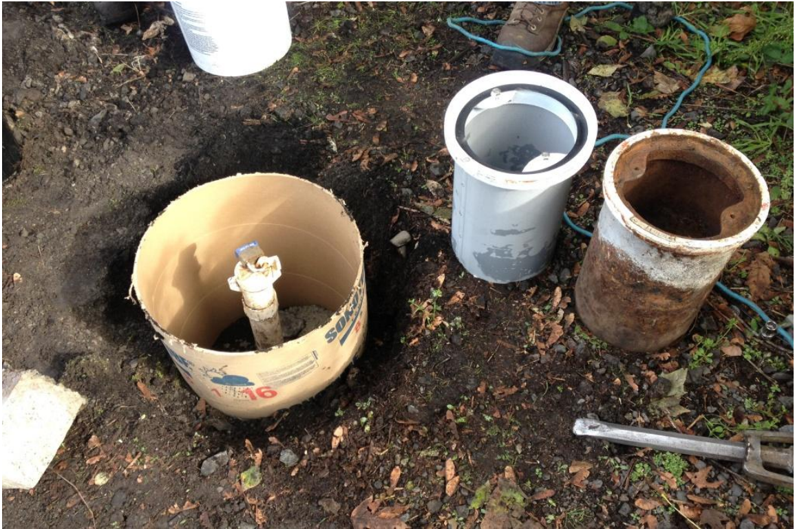
Photograph 5 – MW-58 well under repair. Old surface seal and monument removed. New concrete surface seal is approximately 2-feet deep.
