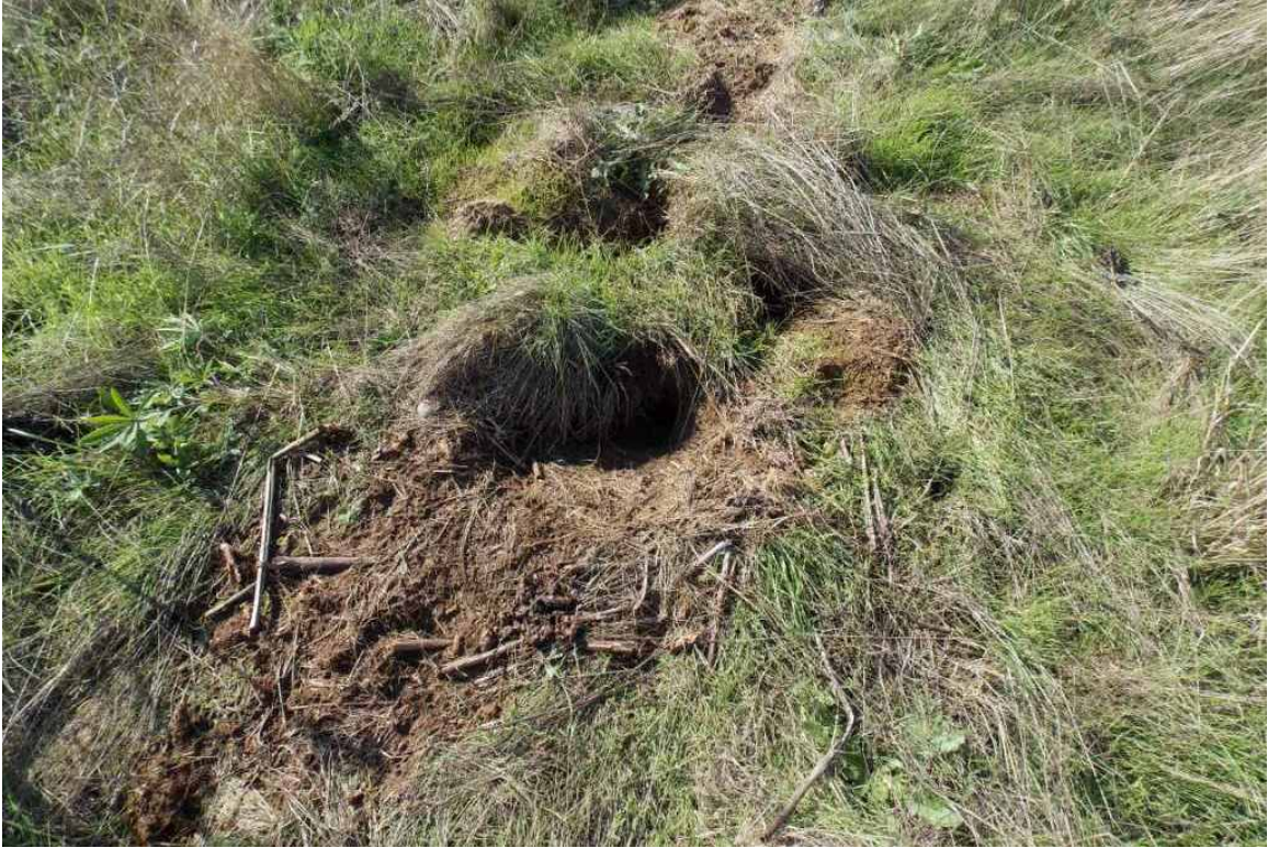
Photograph 1 – Typical rodent holes, these were observed in the stormwater swale area. (October 2013)
