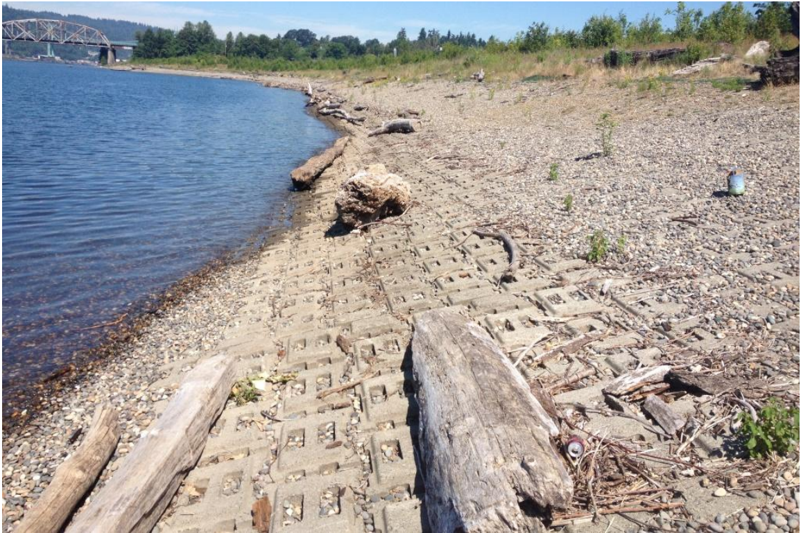
Photograph 9 – Willamette River shoreline showing distribution of woody debris and habitat gravel on ACB armoring. Photograph taken facing northwest.
