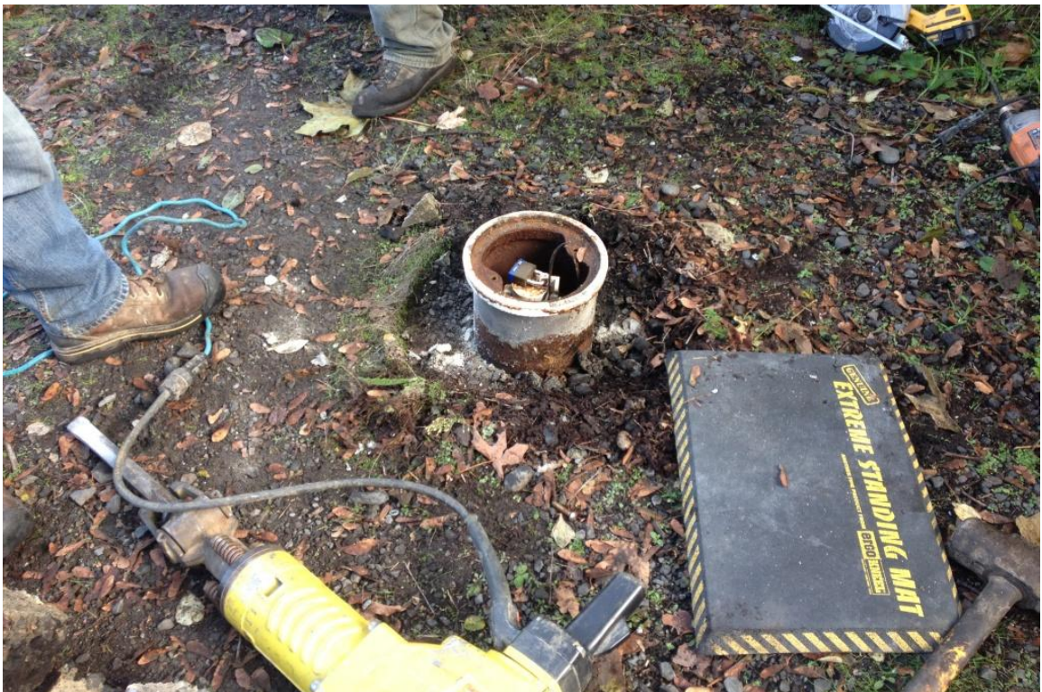
Photograph 4 – MW-58 well under repair. Old concrete surface seal and well monument removed prior to replacement.
