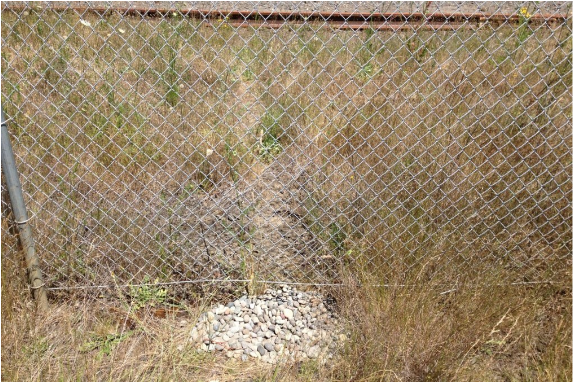
Photograph 1 – Typical animal burrow underneath perimeter fence. Photograph taken facing east with Union Pacific Railroad in the background.
