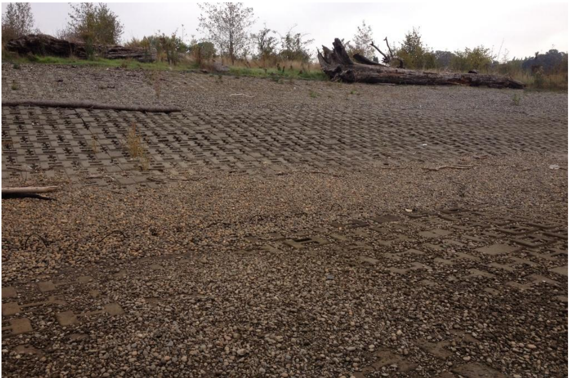
Photograph 10 – Habitat gravel distribution on ACB armoring. Photograph taken facing west.
