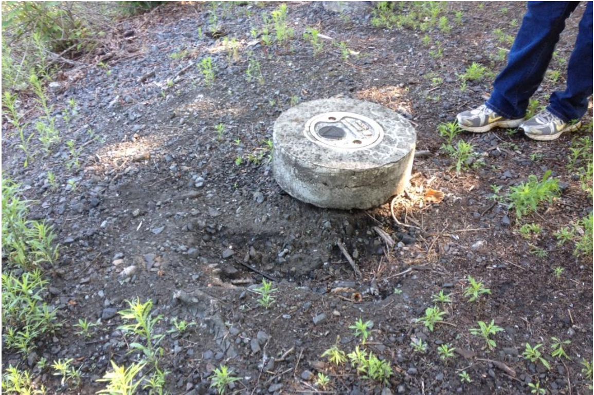
Photograph 3 – One of the MW-58 monitoring wells showing localized erosion and concrete surface seal completely undermined prior to repairs.
