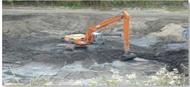
Figure 5. The site during cleanup in the mid-2000s.
