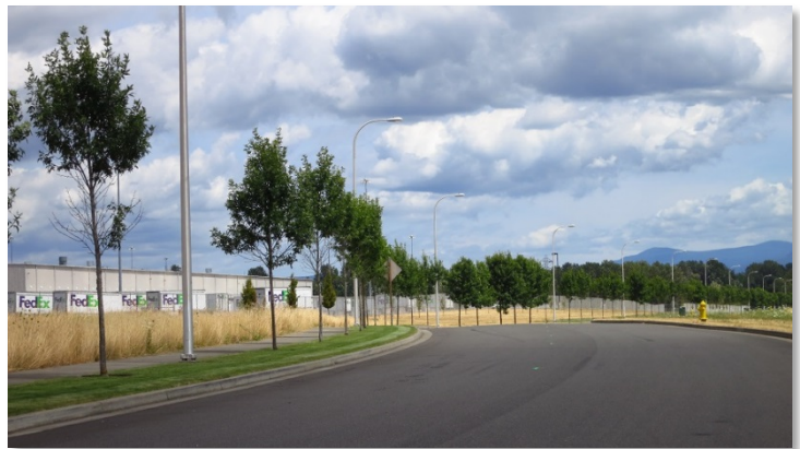
Figure 6. New infrastructure built as part of the Port's Phase I site preparation efforts included roads and storm sewers.
