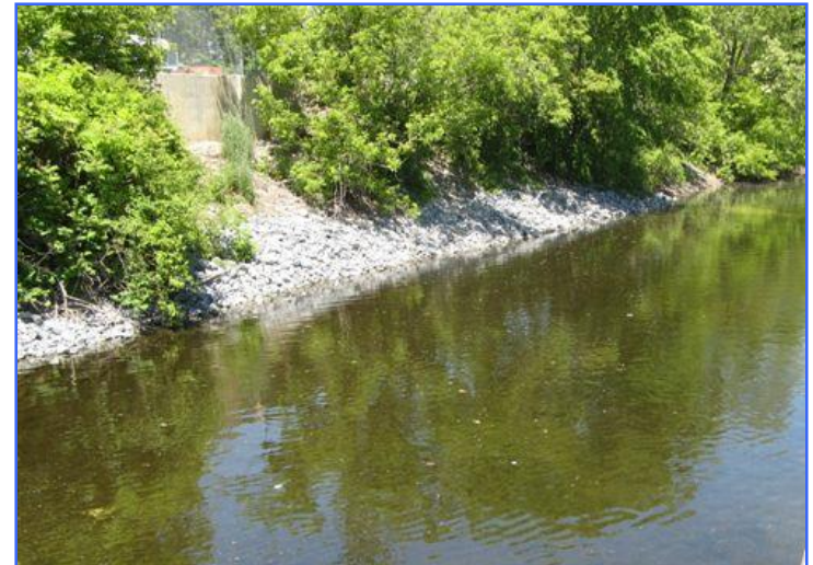
Completed Cap with Armor and rip rap on slope
