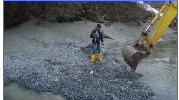
Placement of stone armor over AquaBlok low permeability capping material
