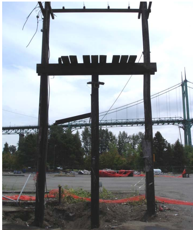
Photo 2: Transformer area following transformer removal and soil removal
