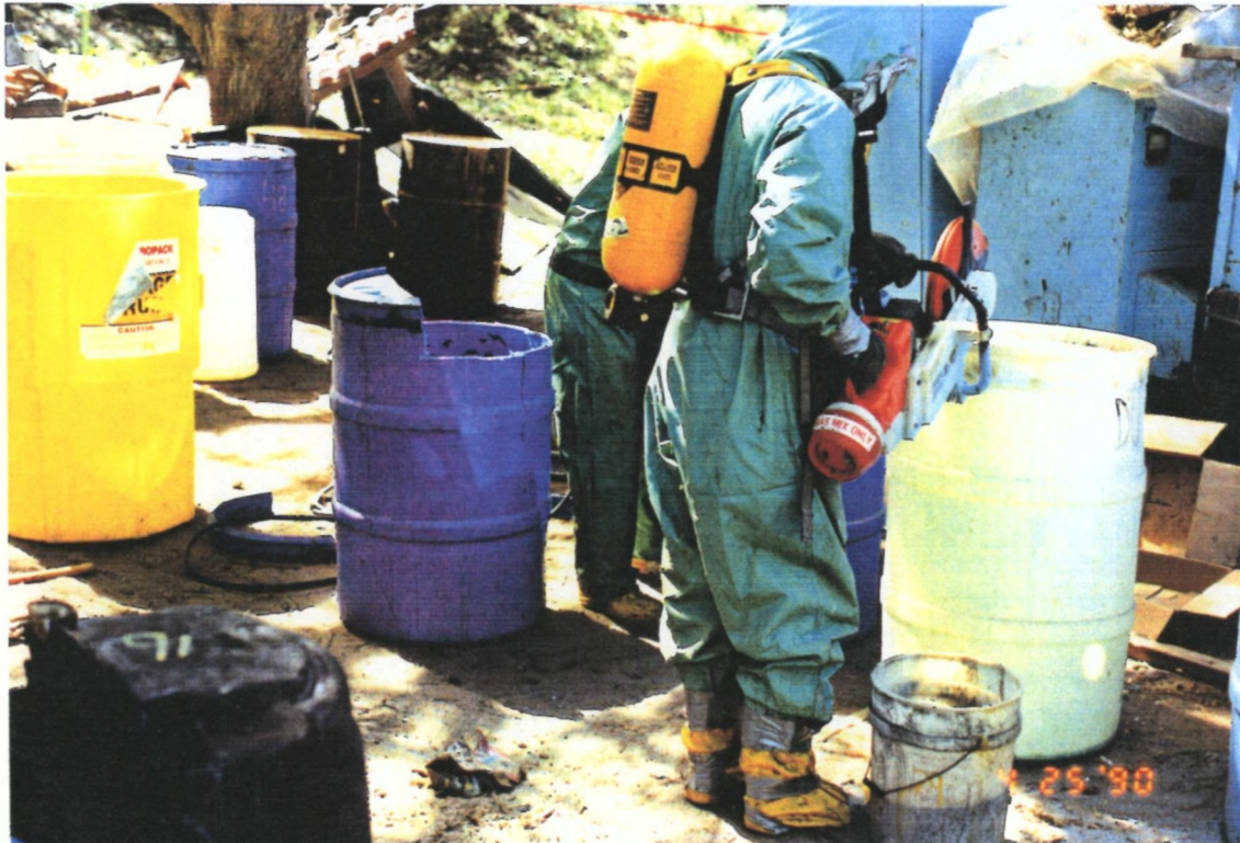
Cutting open drums to facilitate sludge removal.
