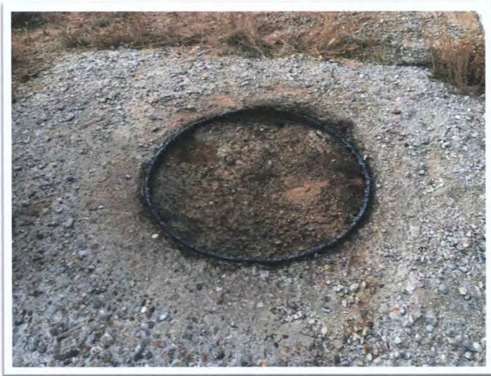
Photograph 24: View of typical cutting of sharp metal surface flush with concrete slab (S3) at MAC No. 1.
