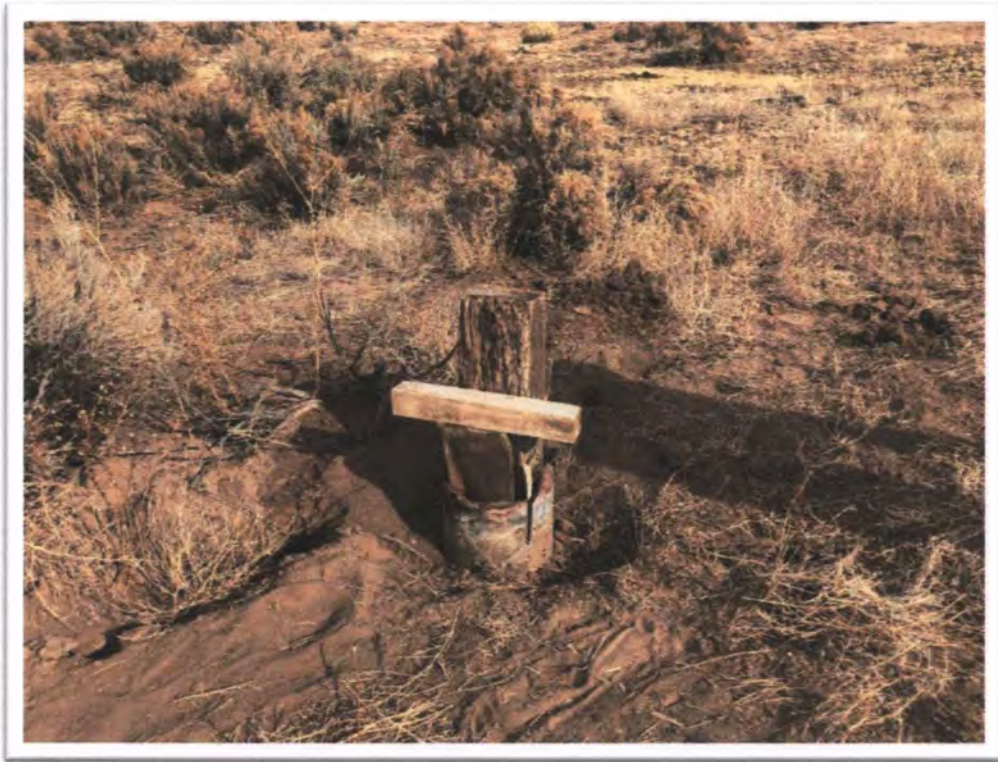
Photograph 17: View of typical plugging and sealing Utility Raise U2 at Black Jack No. 2.
