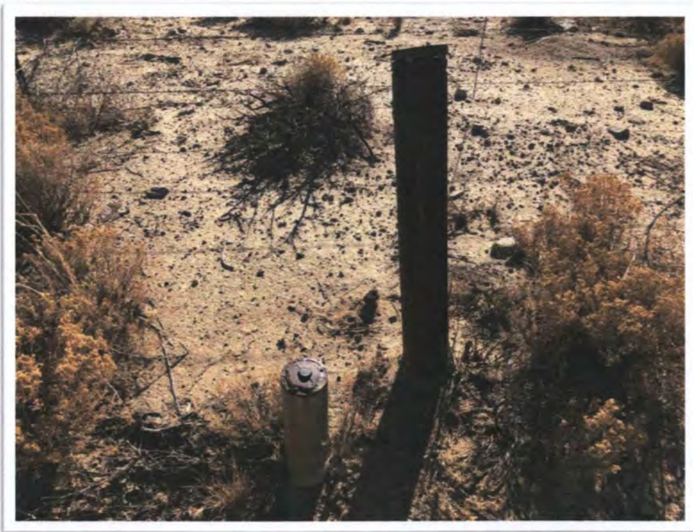
Photograph 10: View of typical cutting of "T"-handle at Utility Raise (U2) at Black Jack No. 1.
