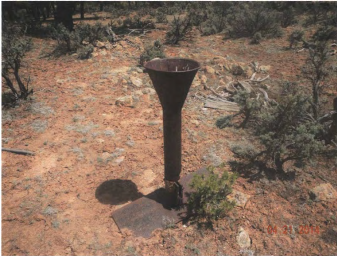
BJ2-9 Utility raise near north vent shaft
