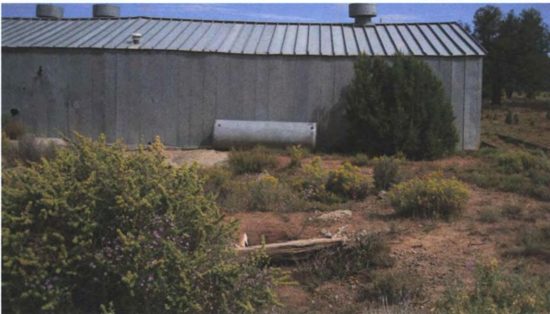
Mac1-5 Collapsed shaft tunnel (foreground, with timbers)
