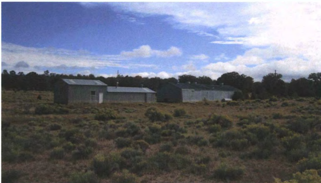
Mac1-1 Mine office building (left) and hoist/ change house (right)
