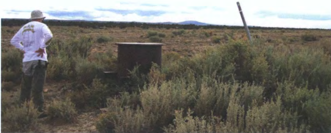
BJ1-7 South vent shaft
