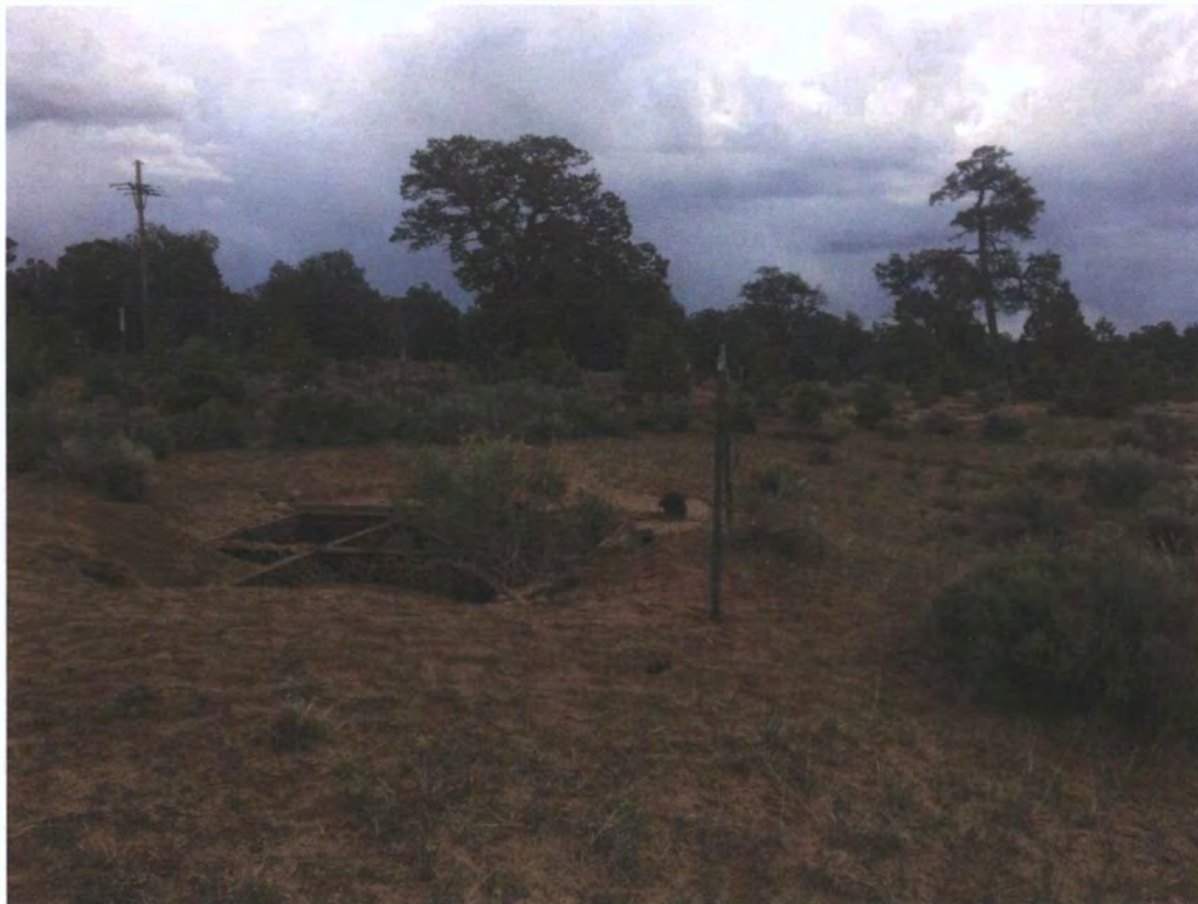
Mac1-3 Mine shaft collar with fencing installed in 2017
