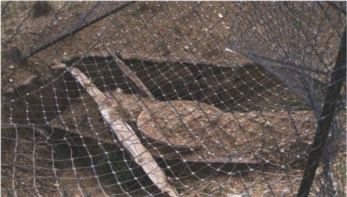
BJ1-4 Close-up view of north vent shaft
