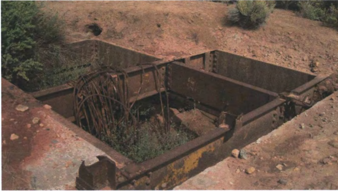
Mac1-2 Mine shaft collar
