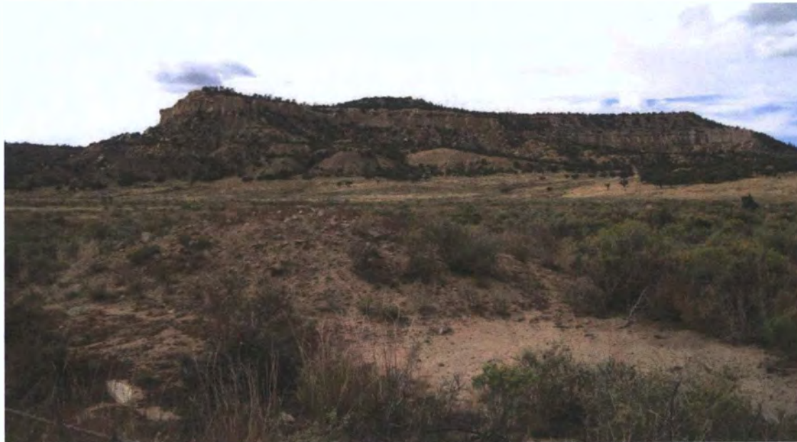
BJ1-2 Main shaft backfill (mound in foreground) looking WNW
