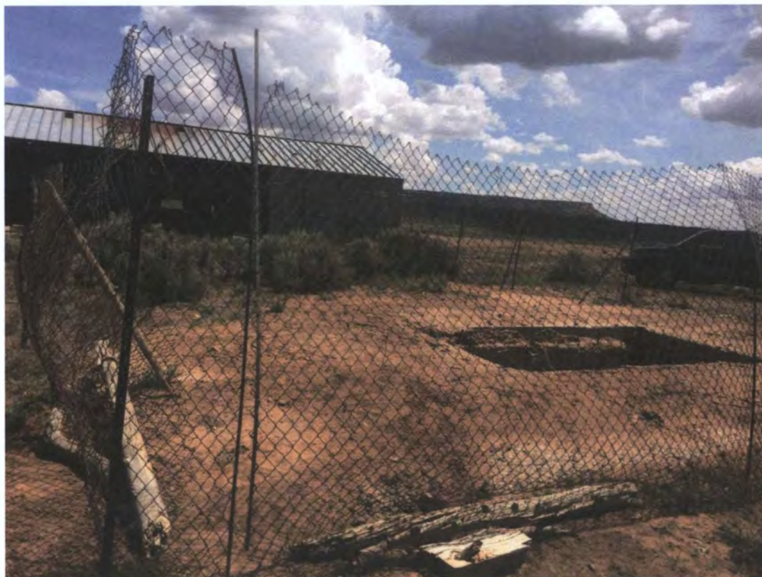
BJ2-4 Fencing around mine shaft improved in 2017, looking northeast
