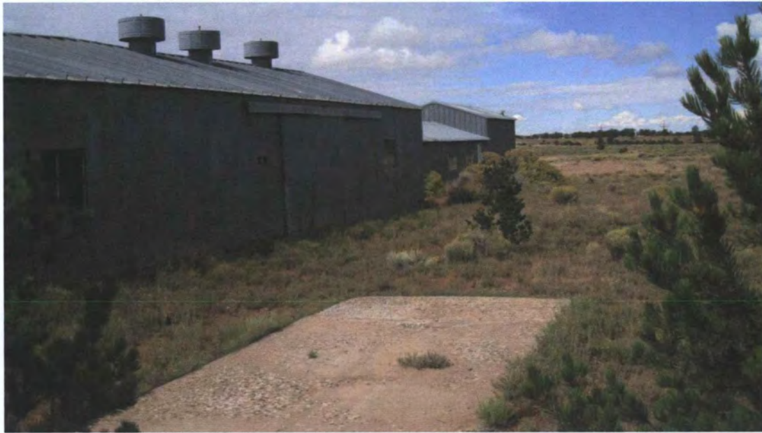
Mac1-6 Concrete slab north of hoist house
