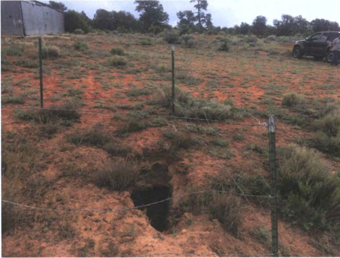
Mac 1-10 Uncovered vent raise south of office building, looking east
