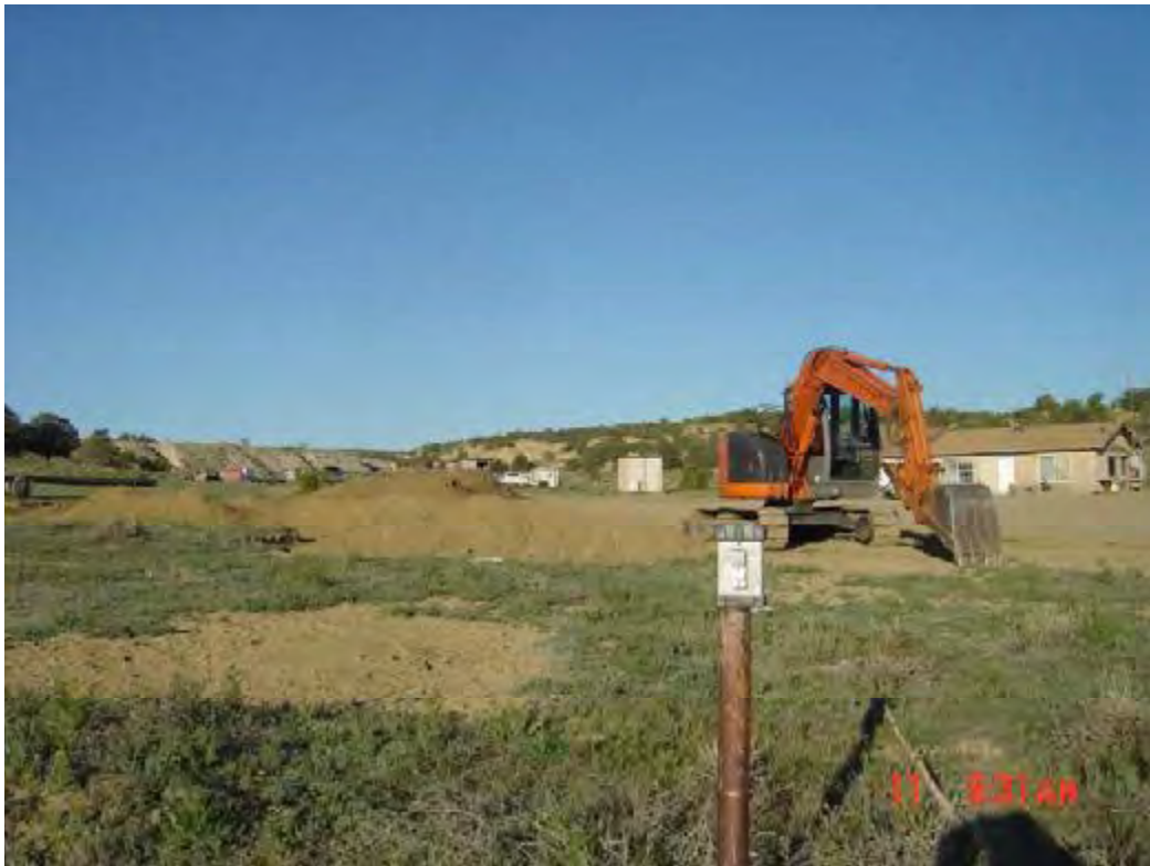
Photo 2: Personal Dust Meter staged downwind during the excavation of Property B.
