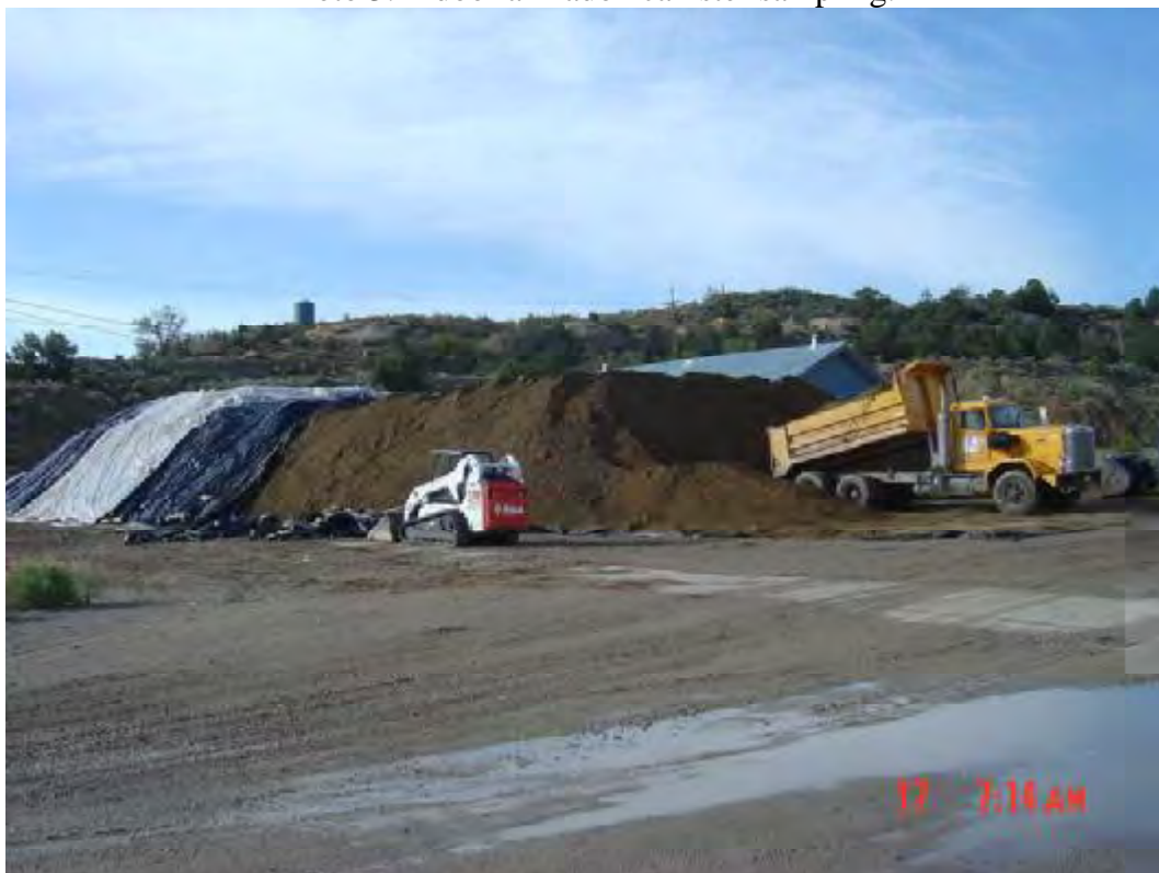
Photo 4: NECR area where soil removed from the homes sites was stockpiled.
