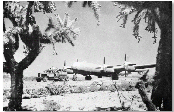
Figure 4. Historical U.S. military operations at site.
