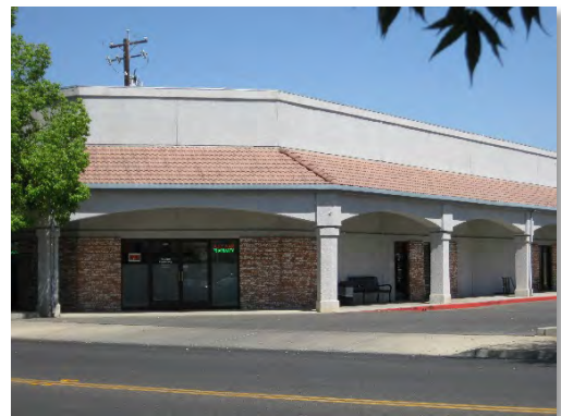
Figure 8. Medical office complex at 155 South 5th Street.
