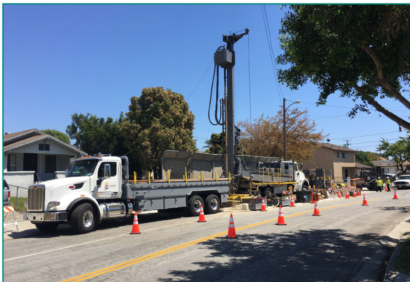
Figure 4: May installation of LW-12. This monitoring well was installed to check contaminants in the deeper aquifer (225 to 245 feet below ground surface).
