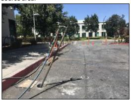
**Photo 4:** Injection hoses connected to angled injection points.
