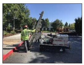
**Photo 3:** Geoprobe making angled direct push injection point in Barriers.
