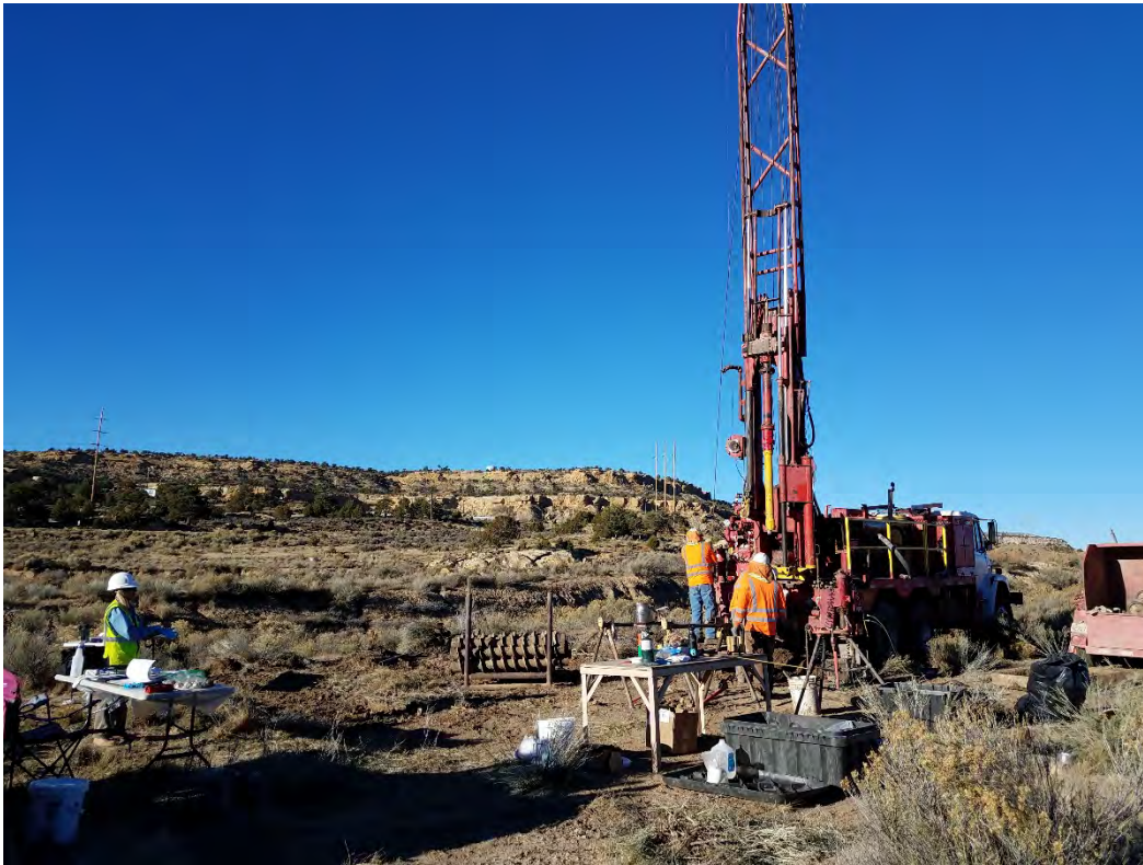
8. GENERAL AREA OF DRILL SITE, LOCATION B6
