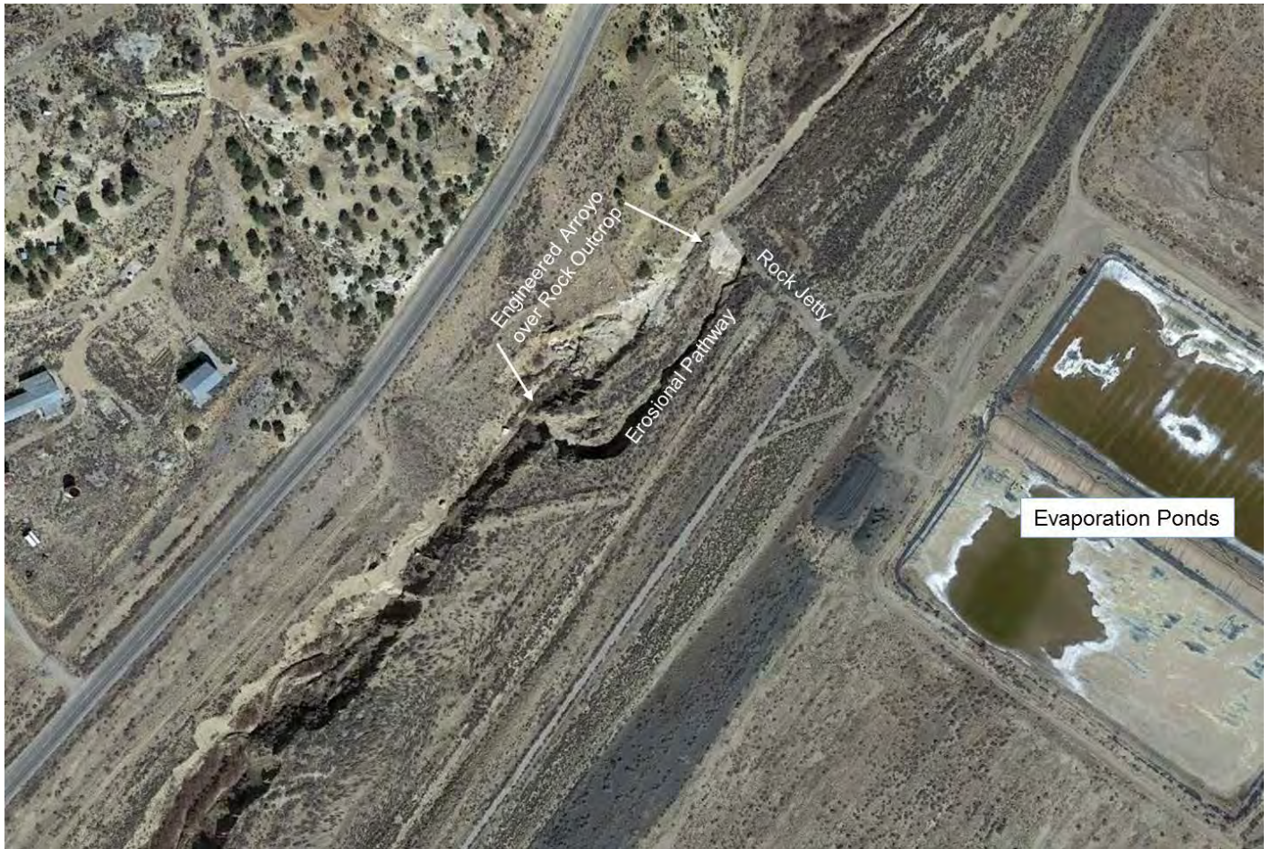
Figure I.7-11: Pipeline Arroyo in the Vicinity of the Rock Jetty
