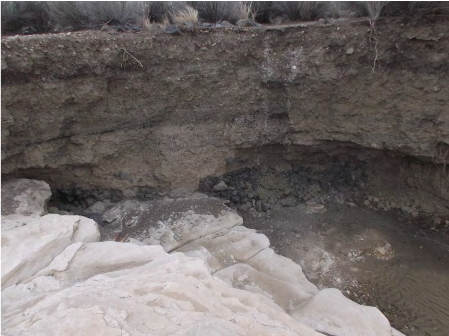
Photo I.7-1: Downstream Side of Rock Jetty (February 18, 2016)
