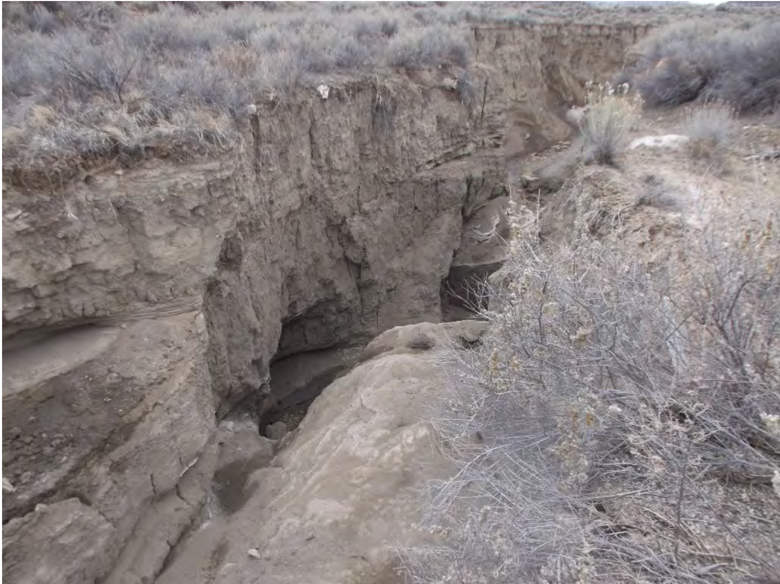
Photo I.7-4: Drainage Cut Approximately 300 Feet Downstream of the Rock Jetty
