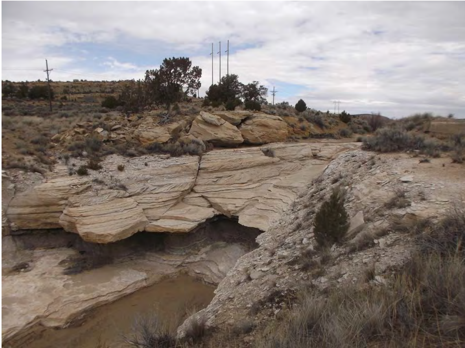
Photo I.7-5: Existing Pipeline Arroyo Channel at the Location of the Rock Outcrop
