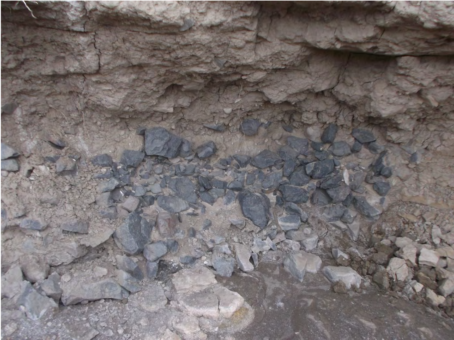
Photo I.7-2: Undercutting of Downstream Side of Rock Jetty
