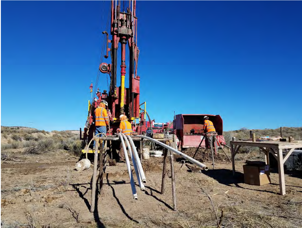
7. DRILLING OPERATIONS, GROUTING BOREHOLE B6
