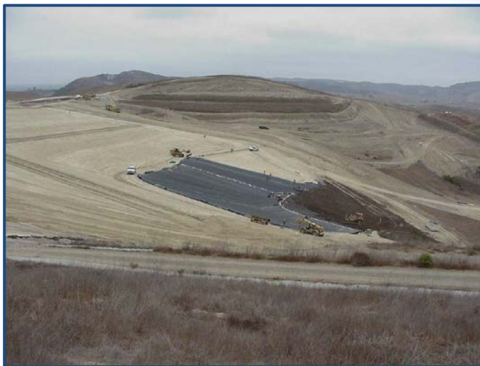
Heavy Metals Landfill (Installation of Geosynthetic Liner)
