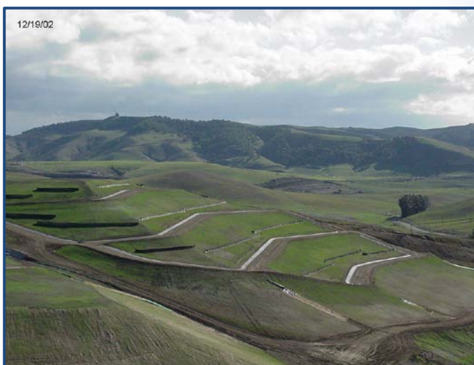
Acids Landfill (following Installation of RCRA Cap including Geosynthetic Liner and Vegetative Cap)
