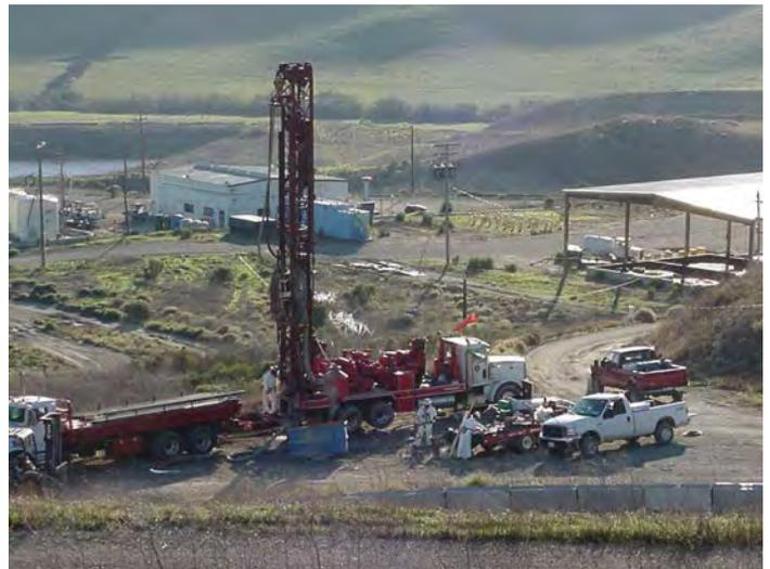
**Figure 3:** Installation of groundwater monitoring well
