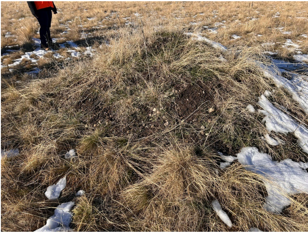
Soil pile observed south of Cedar Street
