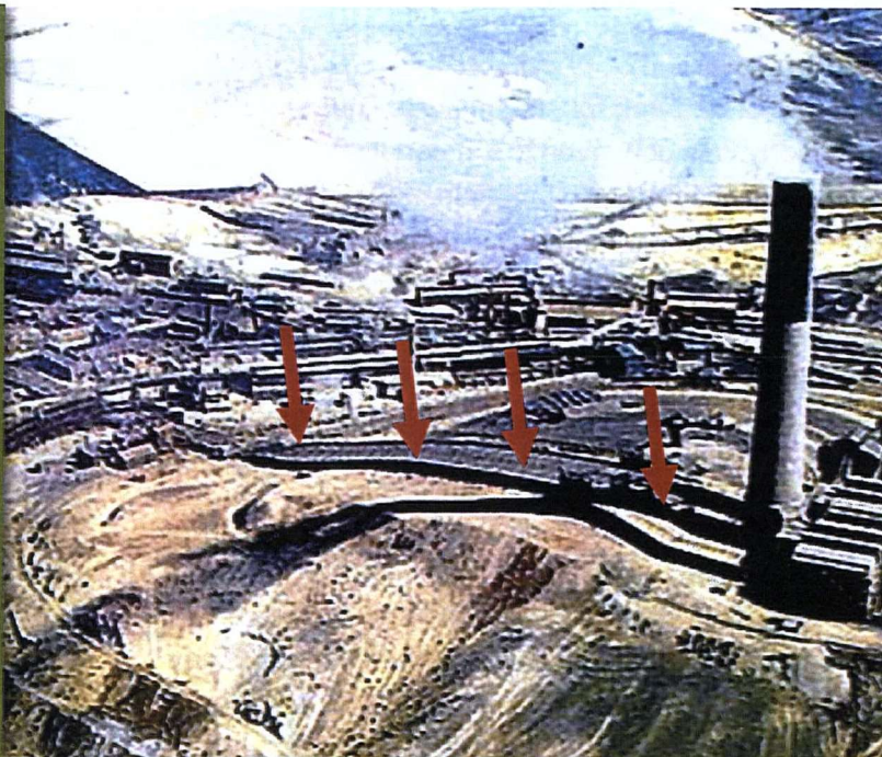
Masonry Flue Leading to Smelter Stack
