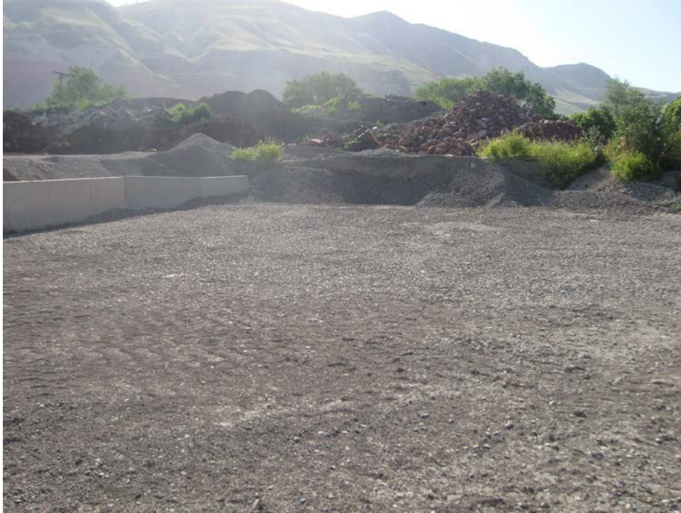
Photo No. 3 – Gravel piles located on the northwest side of the Site; note the piles are above grade.
