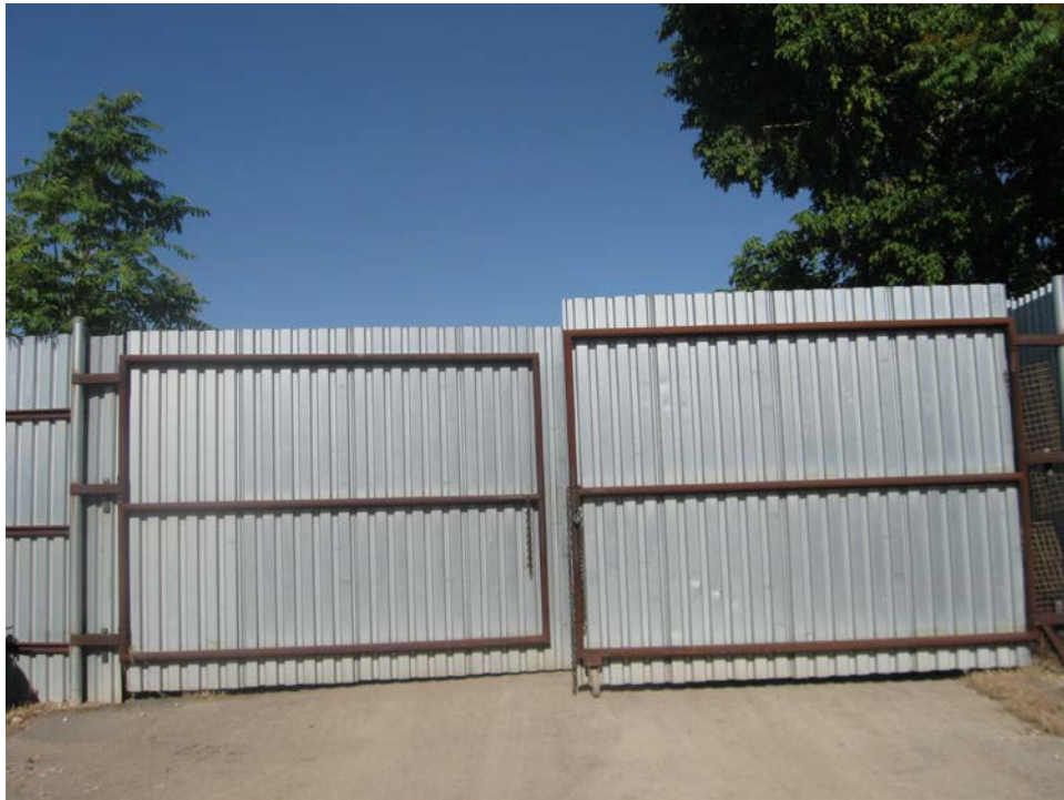
Photo No. 6 – Locked gate to the Site.
