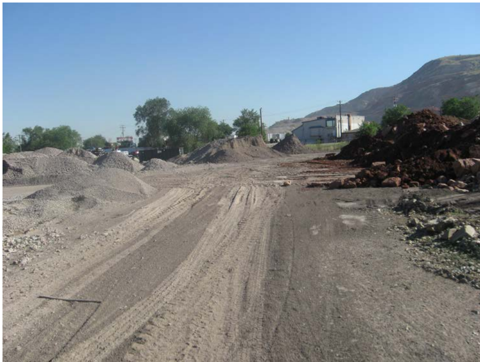
Photo No. 2 – Gravel piles located on the northeast side of the Site; photo looking north.
