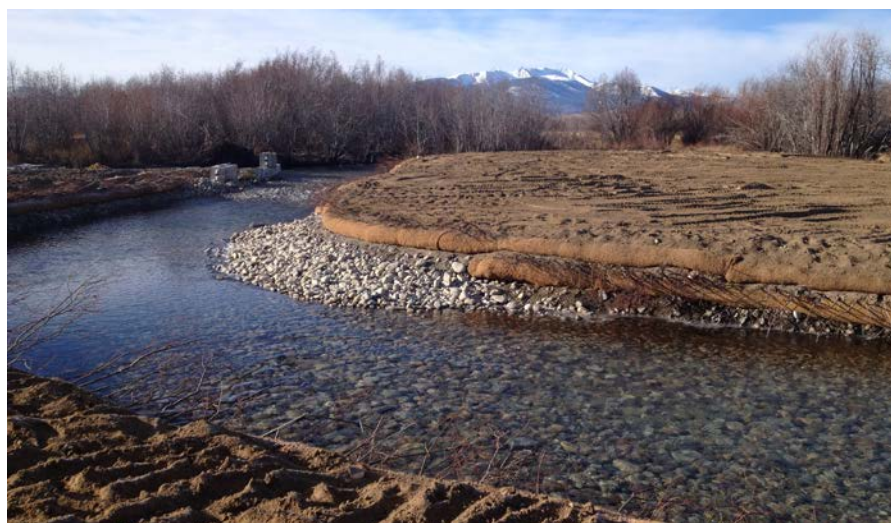
Ongoing remedial action construction at Warm Springs Creek has been designed to both improve water quality and fish habitat by removing mining wastes from inactive meander bends and reconstructing them as new, clean stream channels.
