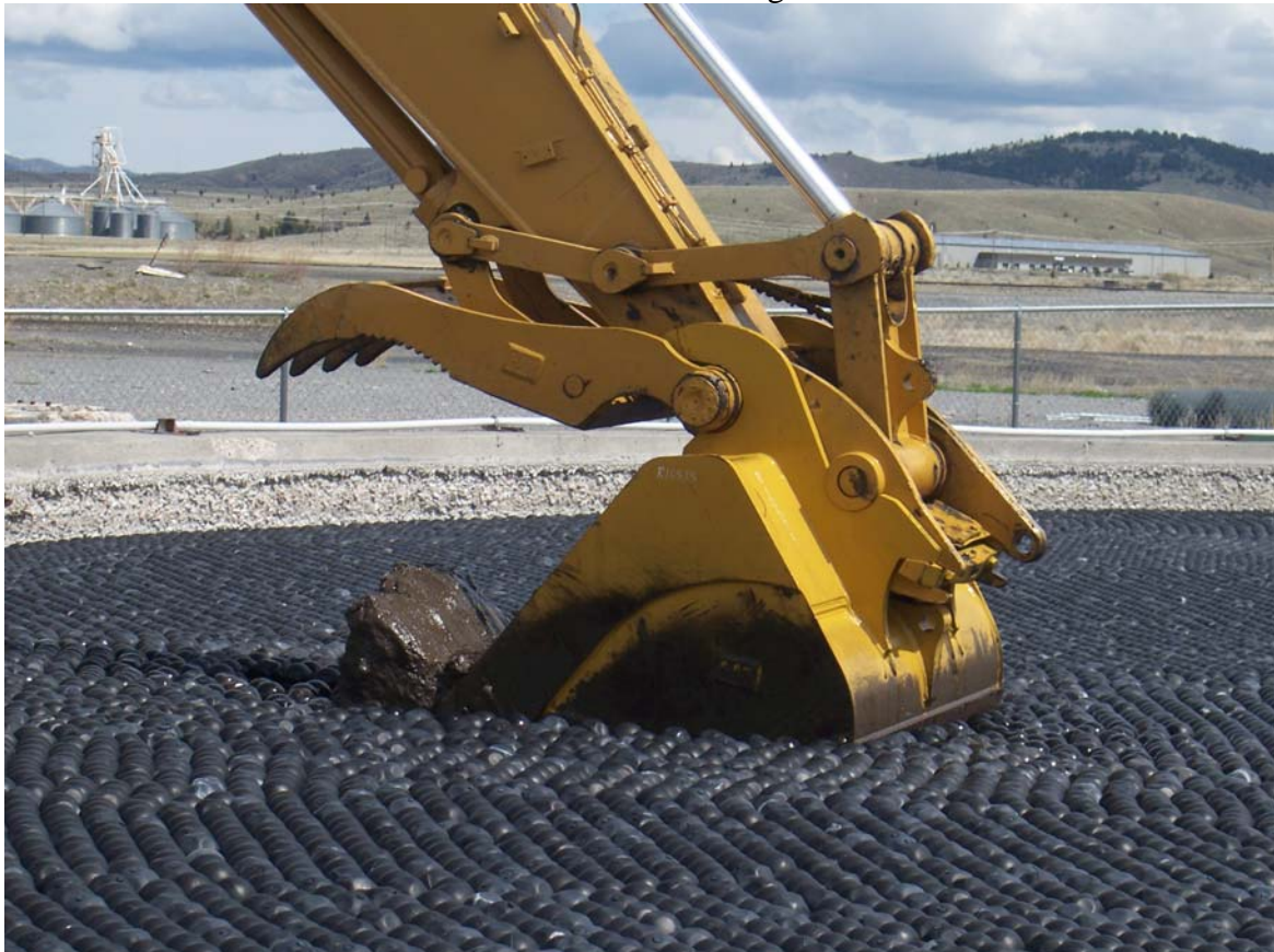
Trackhoe Sampling the Clarifier
