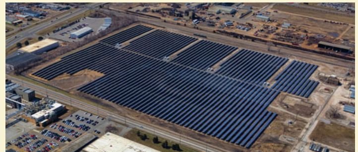
At the Riley Tar Superfund site, the 43-acre Maywood Solar Farm integrates an 11,000 kW solar PV system with the site's capping remedy (Indianapolis, IN).
