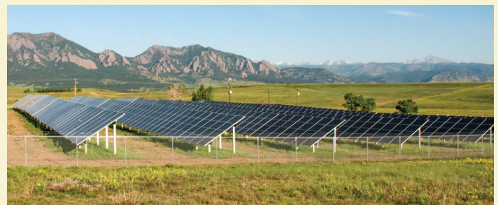
A 500 kW community solar garden at Cowdery Meadows is located on 4 acres at a former landfill (Boulder County, CO).
