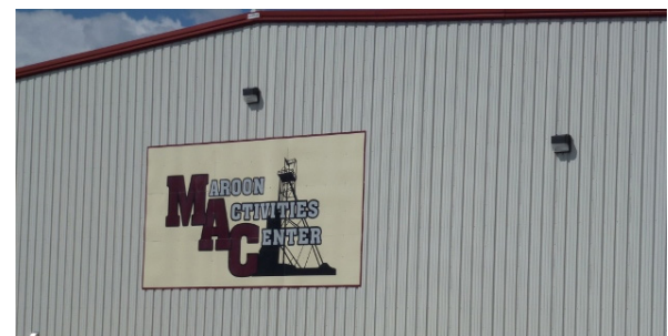
This high school activity center next to the Belmont Mine Yard was built after geophysical studies determined subsidence was not an issue.
