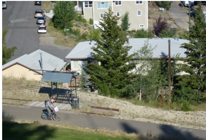
Reclaimed railroad corridor that is now part of the BA&P walk-and-bike trail.
