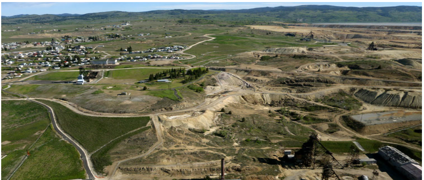
Once heavily impacted by mining waste, large parts of Butte and Walkerville have been reclaimed under the Superfund program.
