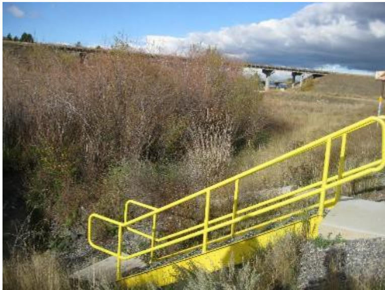
BPSOU: discharge point with view of highway (Butte Silver Bow Wastewater Treatment Plant discharge point is under the highway)
