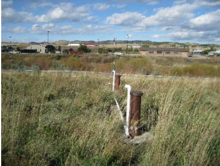
Looking toward Town Pump from Rocker fenced area
