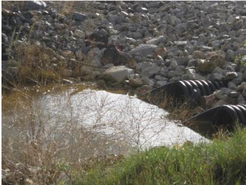
BPSOU: Butte Treatment Lagoons HCC (hydraulic control channel)
