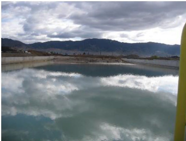
BPSOU: drying bed
