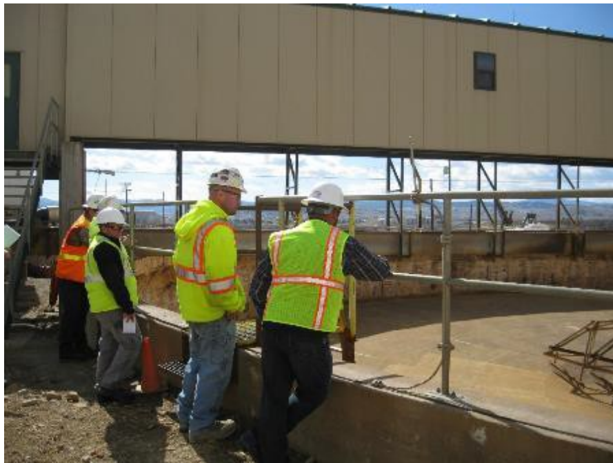
BMFOU: Clarifier – Recently emptied to clean
