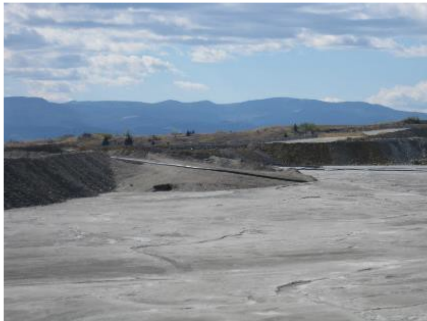
BMFOU: Outfall of Tailing system – 24 million gallons/day recycled back to concentrator
