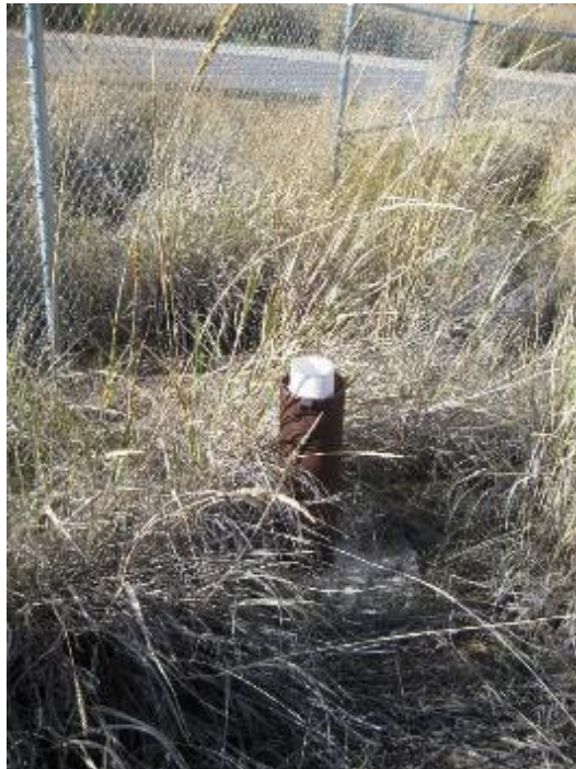
Rocker well with frost heave
