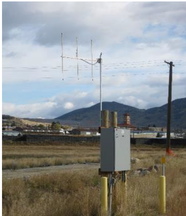
BPSOU: telemetry station at MSD discharge
