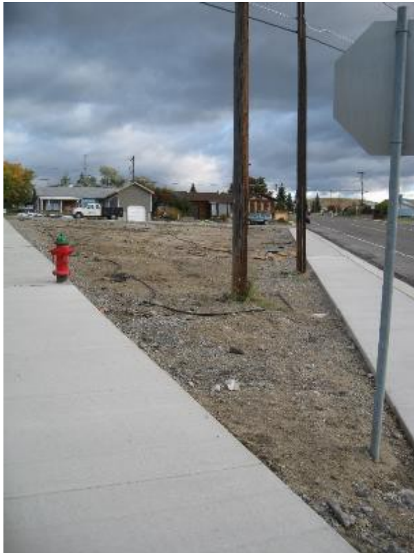
BPSOU: 11 th and Excelsior beginning of a curb and gutter project
