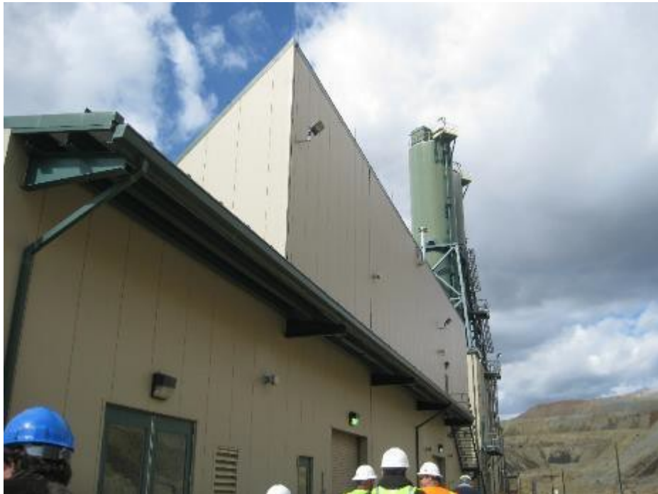
BMFOU: Horseshoe Bend Water Treatment Plant
