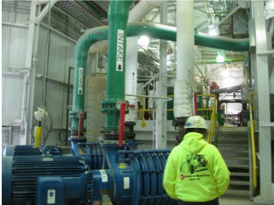
BMFOU: Blowers-reinstalled. They run one at a time.
