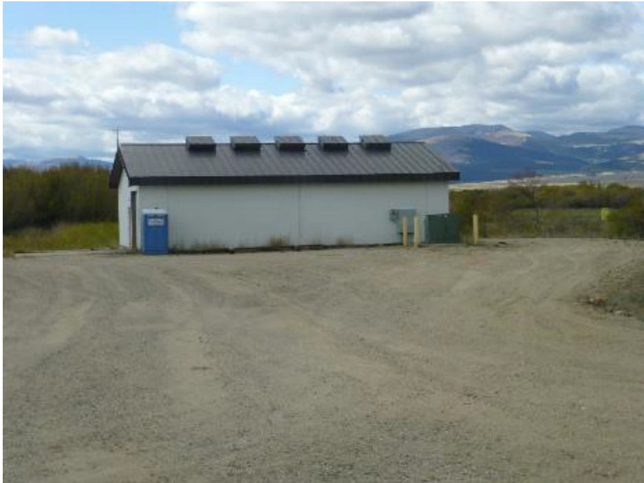
Warm Springs Ponds: Pump station
