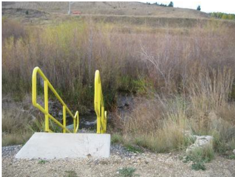
BPSOU: discharge point to creek
