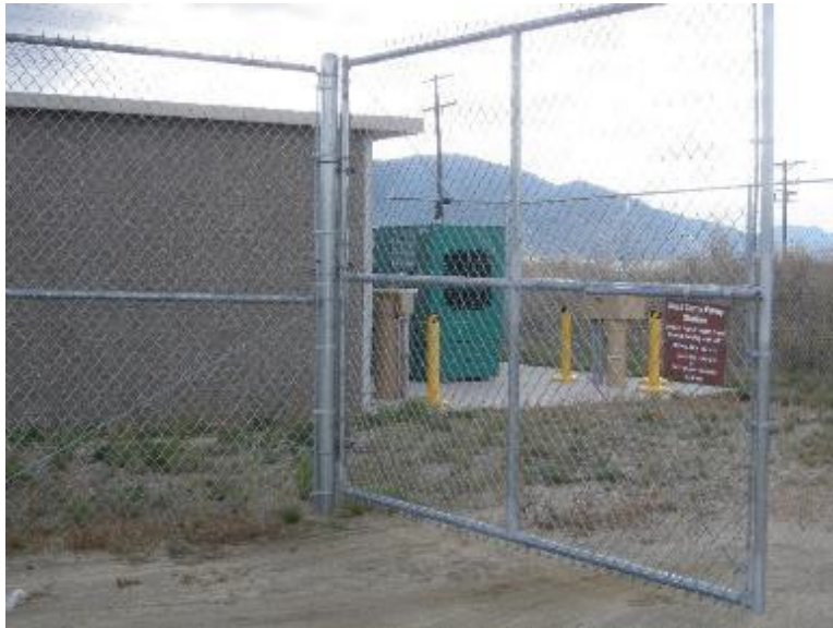
BPSOU: West Camp pump station
