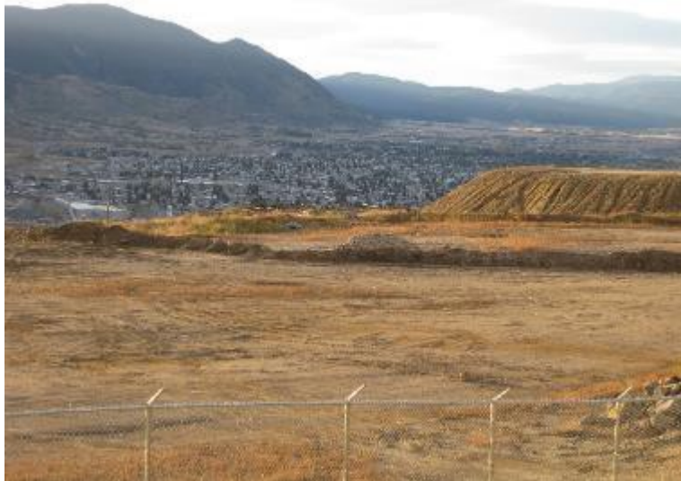
BPSOU: Mine waste repository with cap
