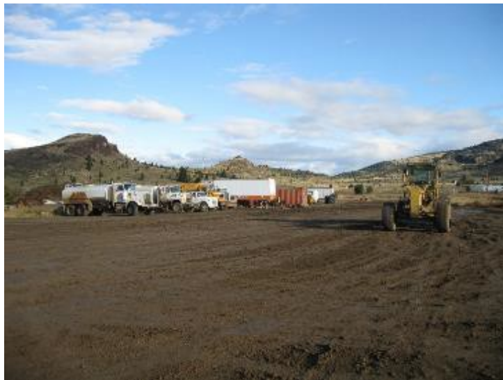
SSTOU: Staging area for construction
