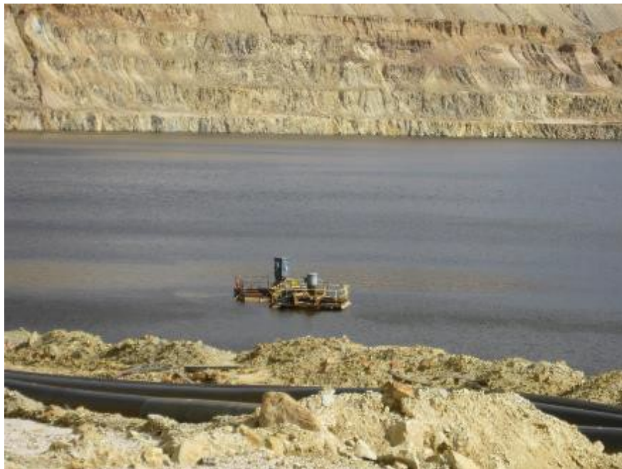
BMFOU: At the water surface of Berkeley Pit – two pumps had gotten disconnected
