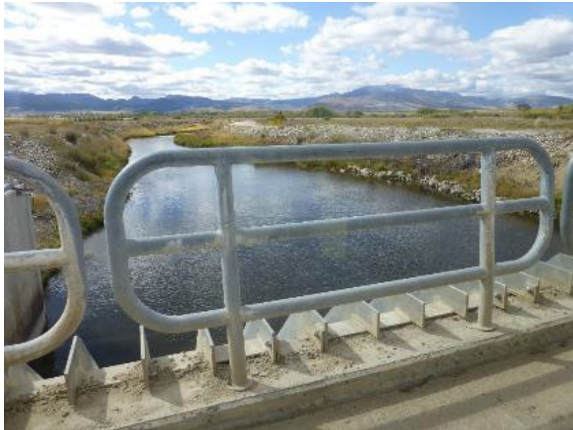
Warm Springs Ponds: Level sensor with an alarm
