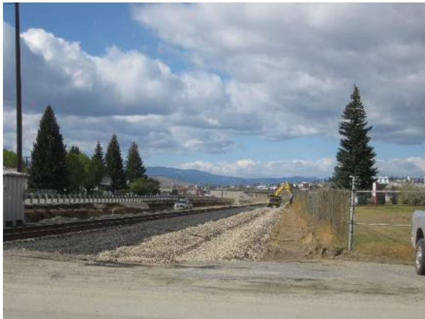
BMFOU: Continental Ditch roadside project
