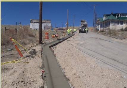
Wyoming Street Steep Challenges for Curb and Gutter Storm Water Control
