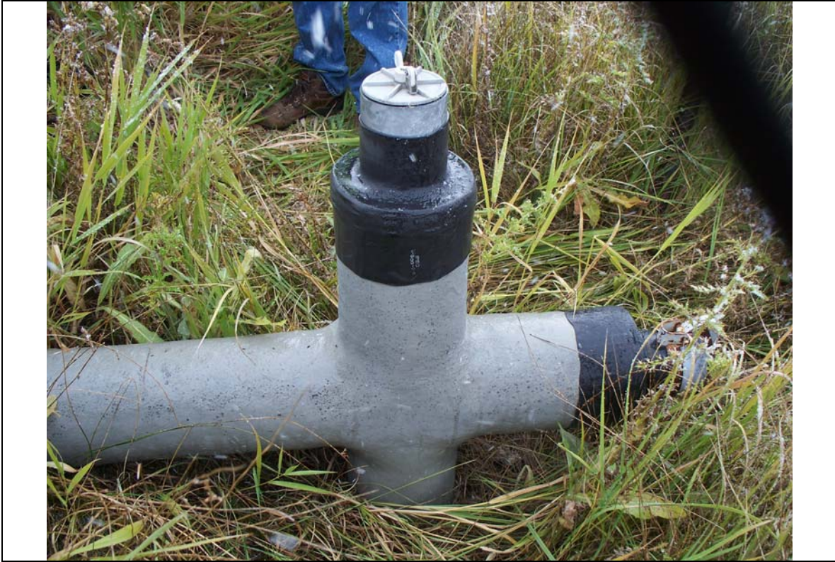
Photo 9. Manifolded Toe Drain.
