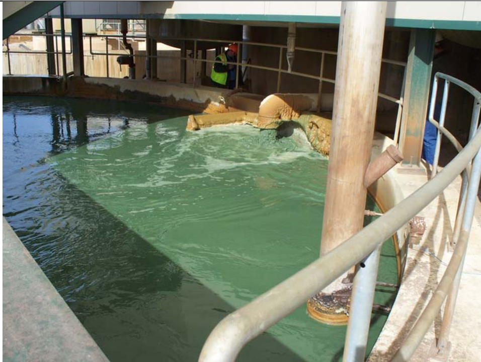
Photo 8. Flow into first stage reactor tank.
