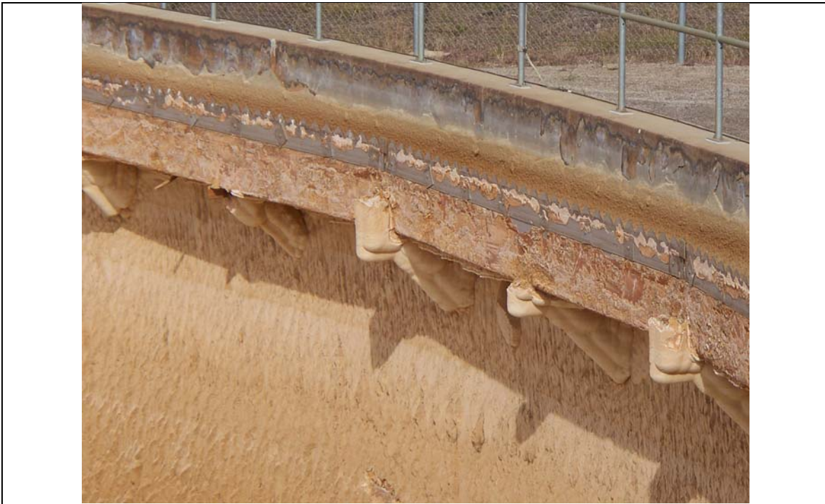
Photo 6. Scale build-up along lip of clarifier overflow.
