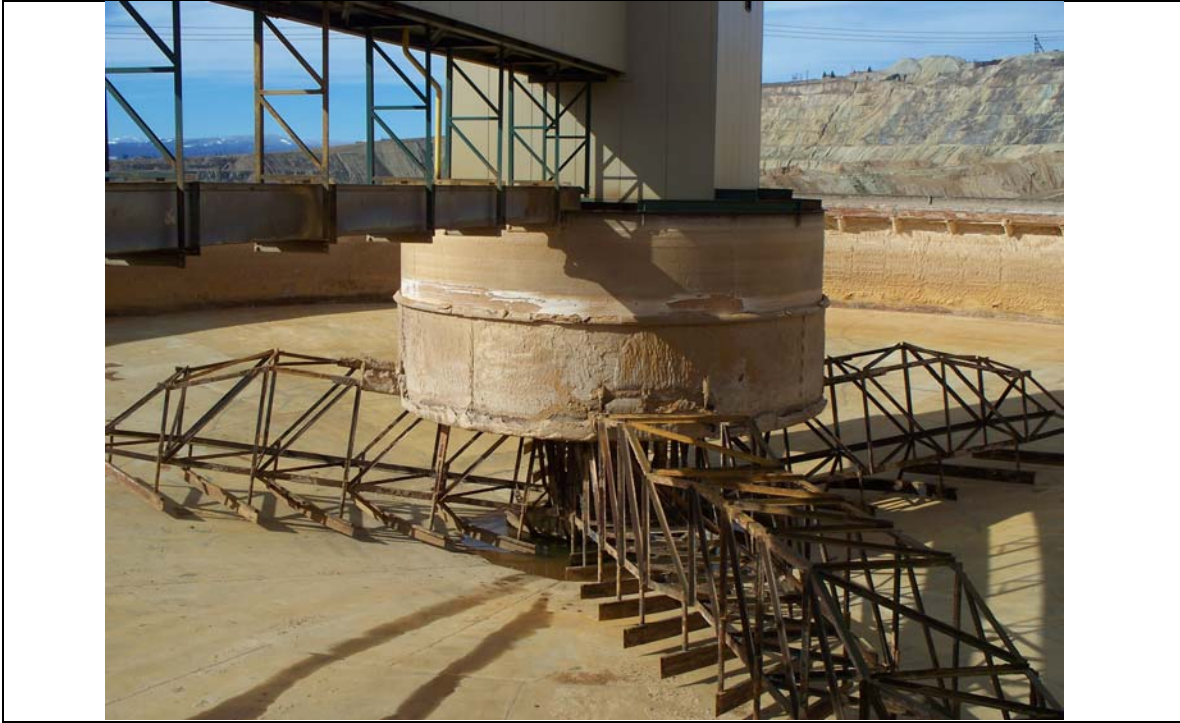
Photo 5. Clarifier with rakes visible (drained for maintenance).
