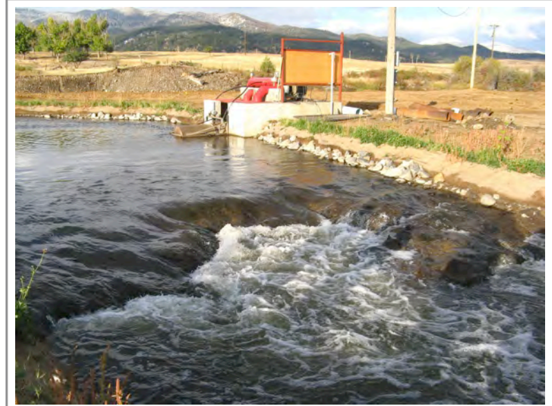
Photo 132: Upper section of Subarea 4—close-up of headcut downstream of pumping station (latitude 46.04443, longitude -112.79708 [WGS 84])
