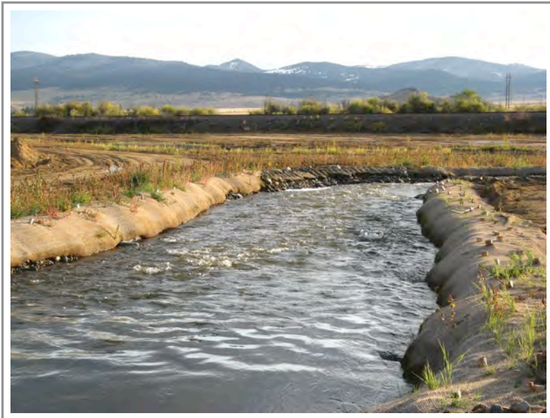
Photo 111: Upper section of Subarea 4—engineered riffle section in reconstructed Silver Bow Creek
