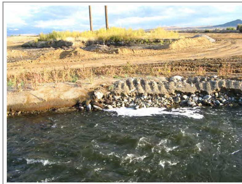
Photo 116: Upper section of Subarea 4—tight curve of newly engineered stream channel showing slight erosion
