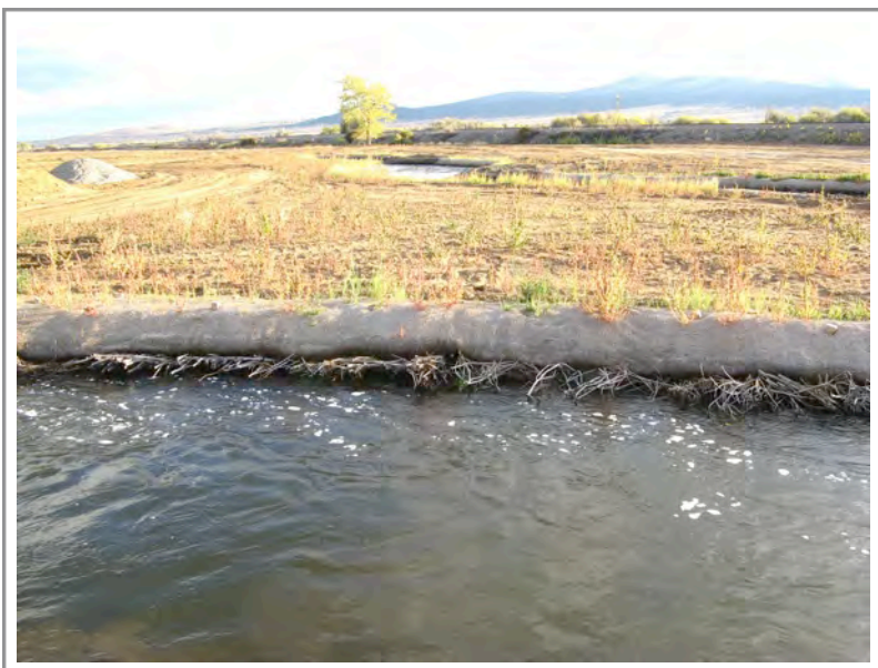
Photo 119: Upper section of Subarea 4—willow stakes protruding from the lower portion of the soil lift
