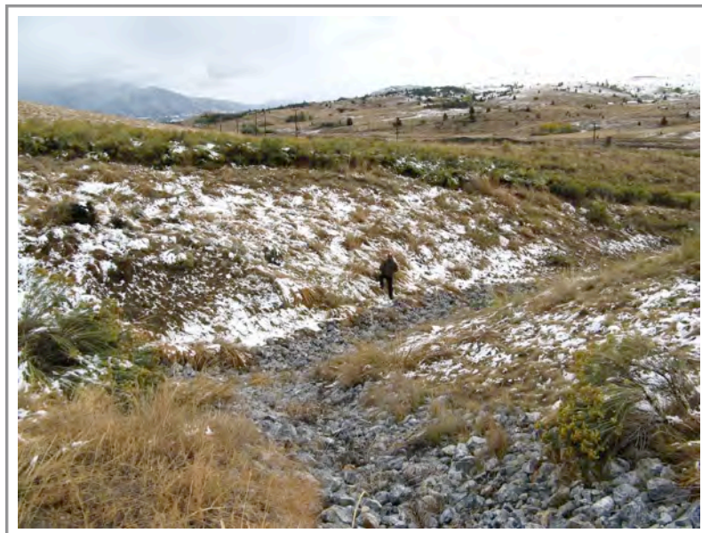
Photo 157: MWRR—rock-lined ditch along the top draining into the ditch upstream of the east pond
