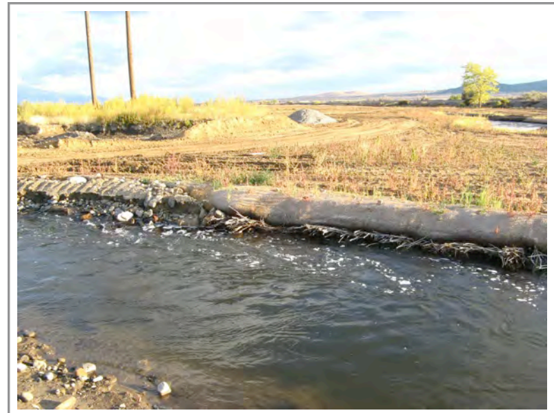
Photo 120: Upper section of Subarea 4—willow stakes protruding from the lower portion of the soil lift
