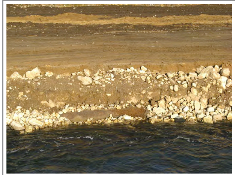
Photo 130: Upper section of Subarea 4—erosion of streambank downstream of pumping station
