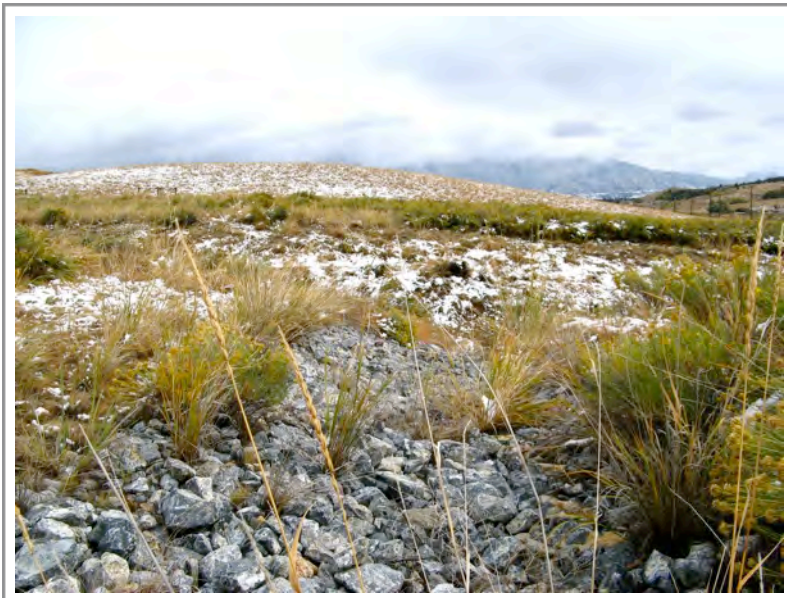
Photo 150: MWRR—rock-lined drainage ditch along the northeast portion (top) of the repository
