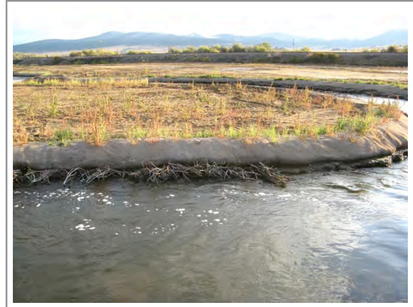
Photo 118: Upper section of Subarea 4—willow stakes protruding from the lower portion of the soil lift
