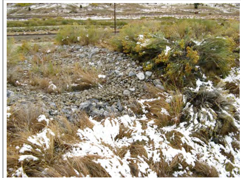
Photo 143: MWRR—west pond rock-lined emergency spillway
