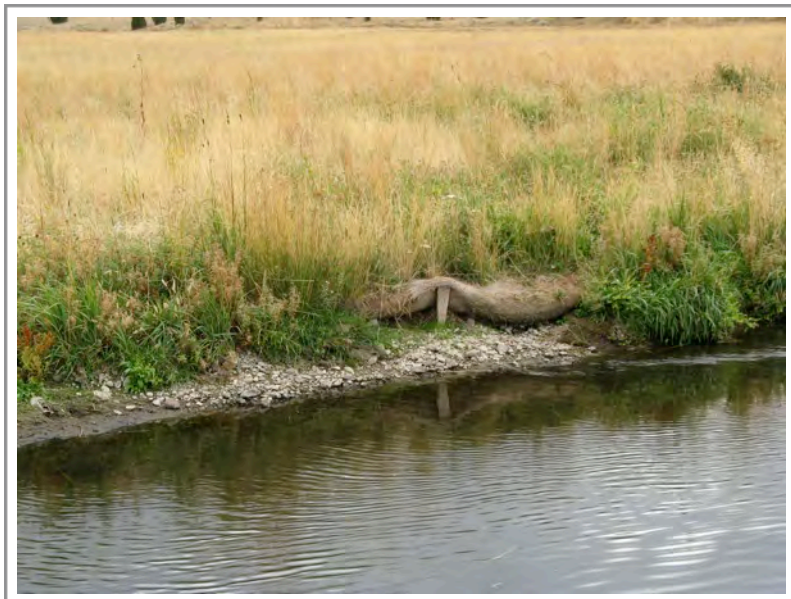
Photo 44: Middle section of Subarea 2—exposed soil lift adjacent on Silver Bow Creek streambank
