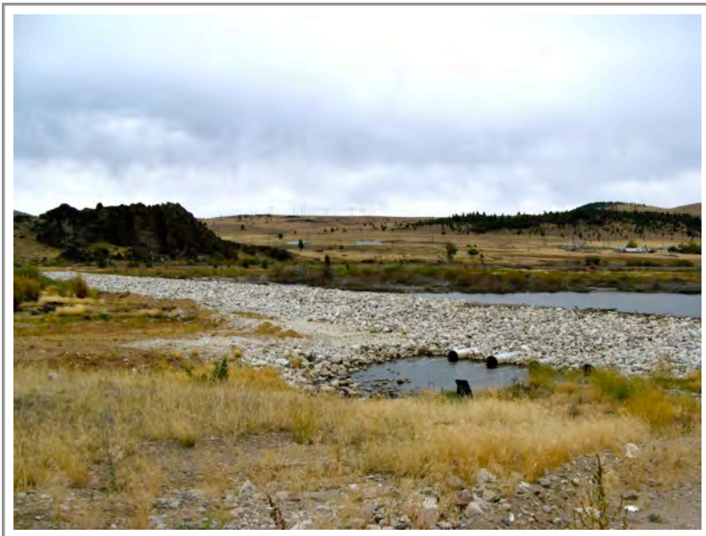
Photo 96: Lower section of Subarea 3—temporary sediment retention dam showing outlet culverts
