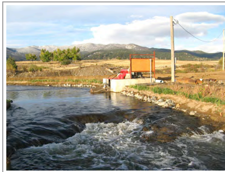
Photo 124: Upper section of Subarea 4—headcut moving upstream towards the newly installed irrigation pumping station
