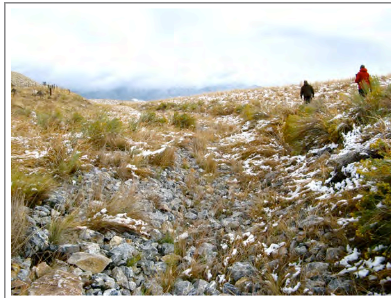
Photo 149: MWRR—rock-lined drainage ditch along the north end (top) of the repository
