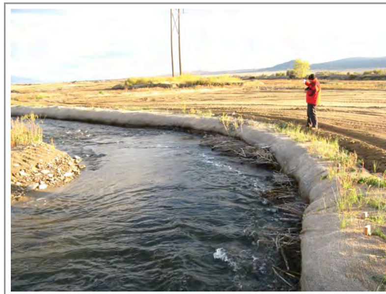
Photo 108: Upper section of Subarea 4—overview of both sides of reconstructed streambanks
