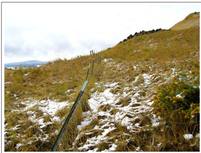
Photo 154: MWRR—downed fence along the northeast section of the repository
