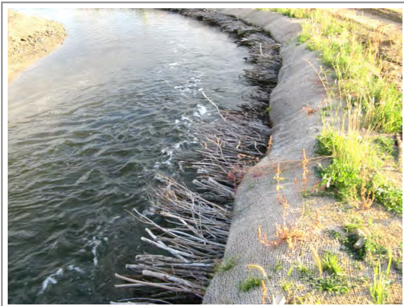
Photo 123: Upper section of Subarea 4—close-up of willow stakes protruding from the lower portion of the soil lift on the outside of a curve
