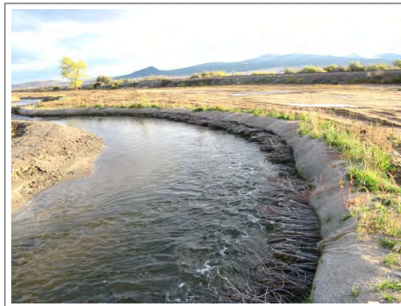
Photo 122: Upper section of Subarea 4—long curving streambank showing willow stakes protruding from the lower portion of the soil lift
