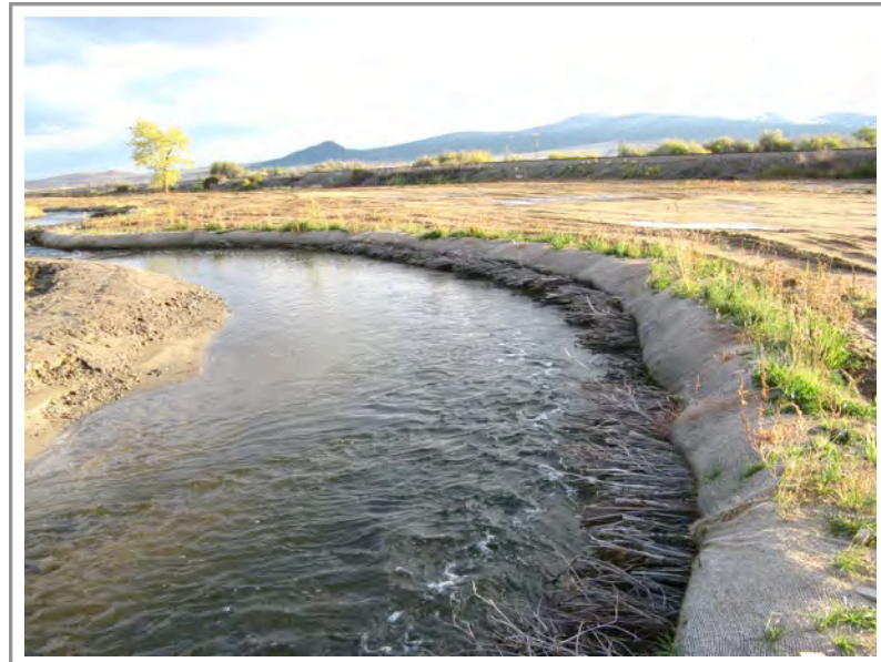
Photo 122: Upper section of Subarea 4—long curving streambank showing willow stakes protruding from the lower portion of the soil lift
