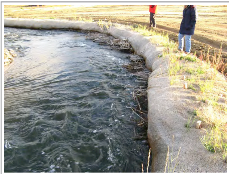
Photo 107: Upper section of Subarea 4—willow stakes at water's edge on outside curve
