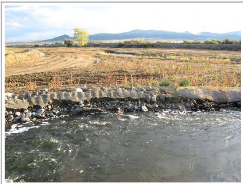
Photo 117: Upper section of Subarea 4—tight curve of newly engineered stream channel showing slight erosion
