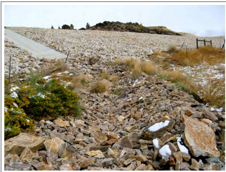
Photo 148: MWRR—rock-lined drainage ditch along the north end (top) of the repository
