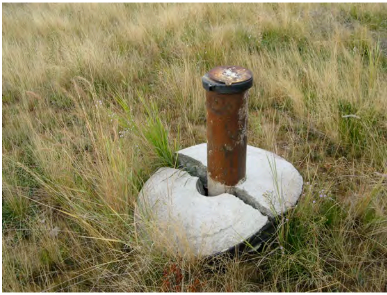
Photo 72: Ramsay Flats section of Subarea 2—unlocked well (G 135) with broken base at latitude 46.00032, longitude -112.68661 (WGS 84)
