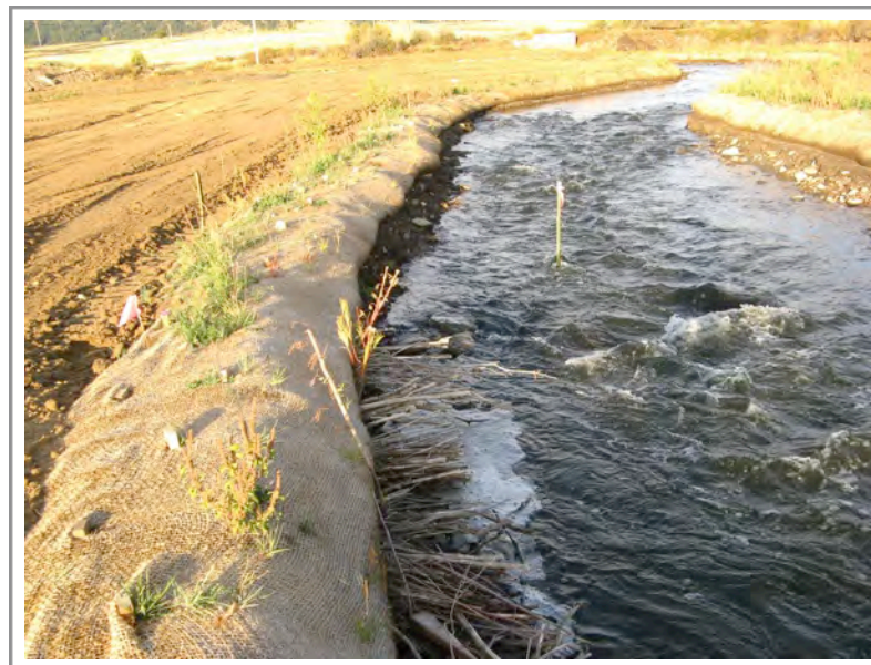
Photo 106: Upper section of Subarea 4—willow stakes installed below soil lift
