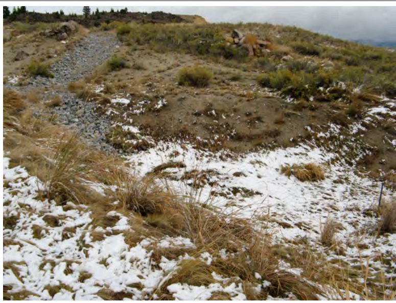
Photo 140: MWRR—view of west pond showing rock-lined drainage ditch
