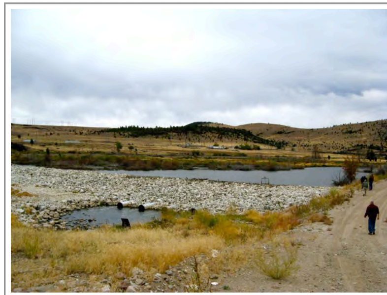
Photo 95: Lower section of Subarea 3—temporary sediment retention dam showing outlet culverts
