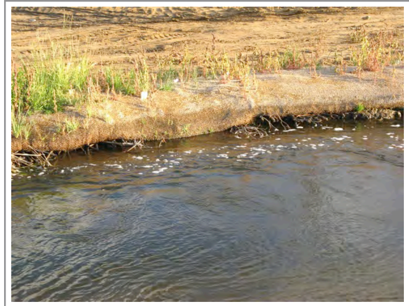
Photo 110: Upper section of Subarea 4—photo showing some gaps below a soil lift on a newly constructed streambanks
