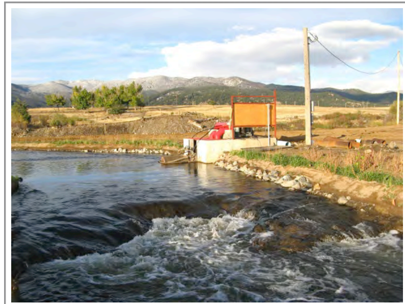
Photo 124: Upper section of Subarea 4—headcut moving upstream towards the newly installed irrigation pumping station
