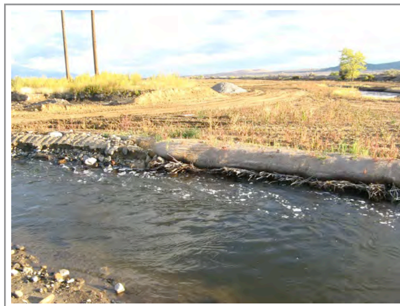
Photo 120: Upper section of Subarea 4—willow stakes protruding from the lower portion of the soil lift
