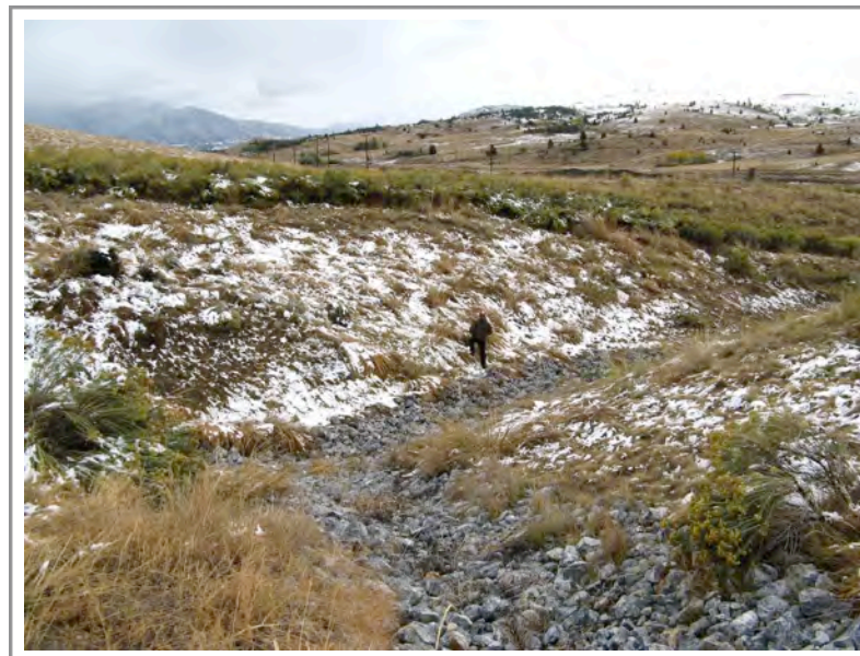
Photo 157: MWRR—rock-lined ditch along the top draining into the ditch upstream of the east pond
