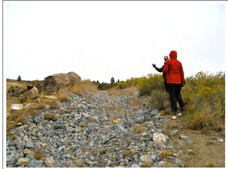
Photo 145: MWRR—rock-lined drainage ditch along north end of repository
