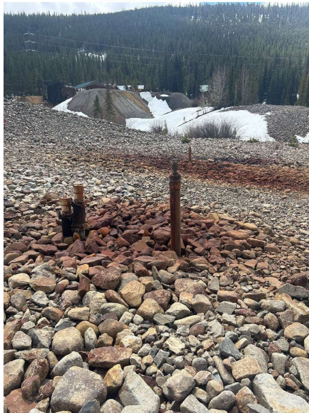
New injection well in foreground and old injection well and mining structure in background
