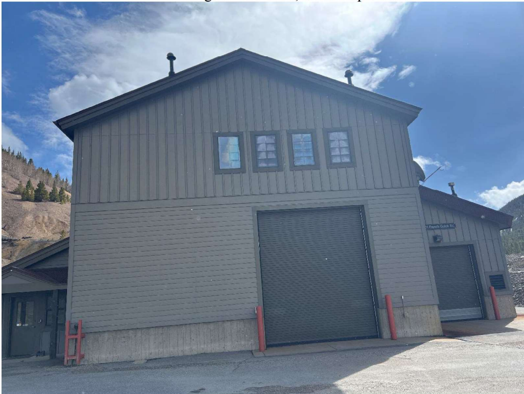
The WTP building
