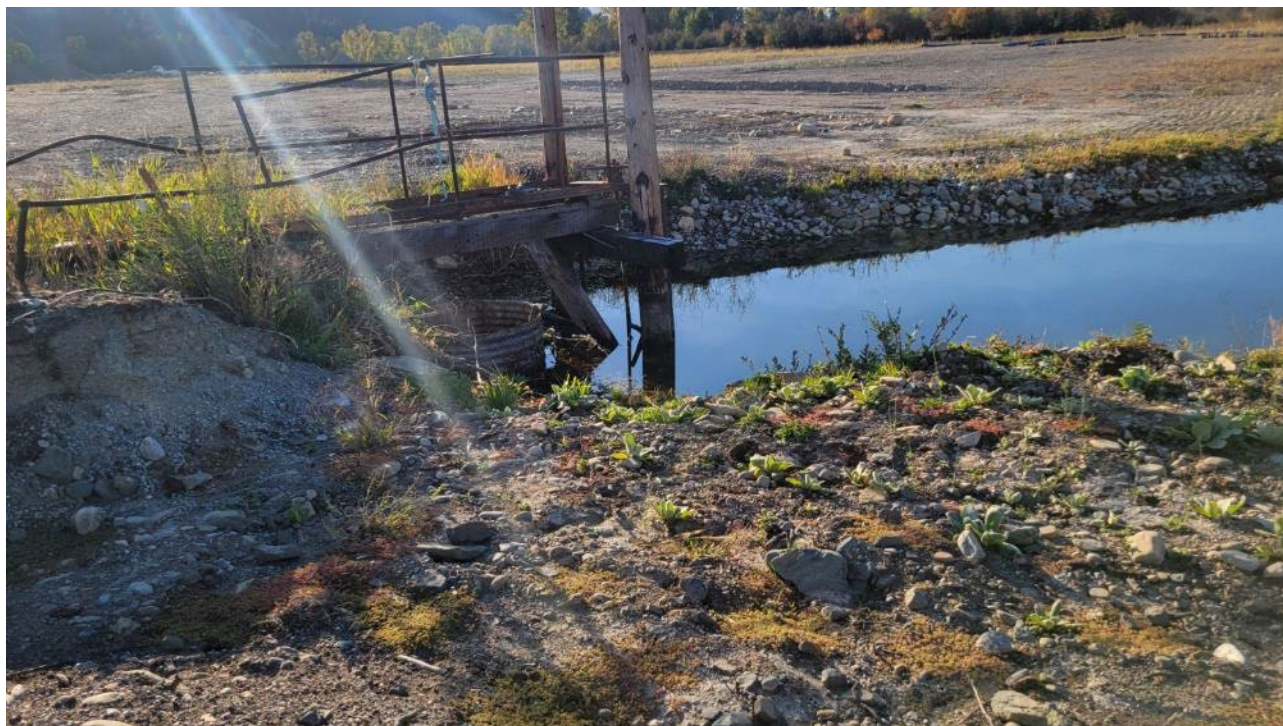
Photograph 14: Outlet of fire pond. Note that water level is below outlet elevation.
