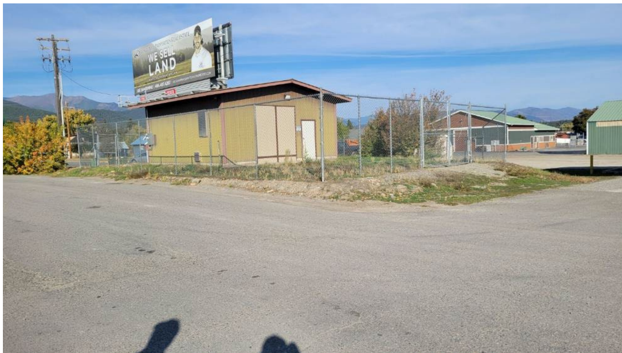
Photograph 27: Old well building converted to record storage.
