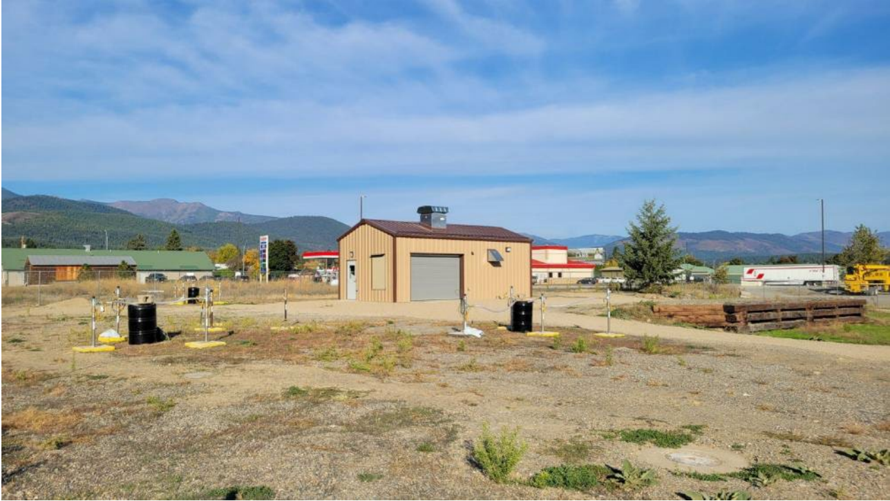
Photograph 23: Area 2 ISB nested monitoring wells.
