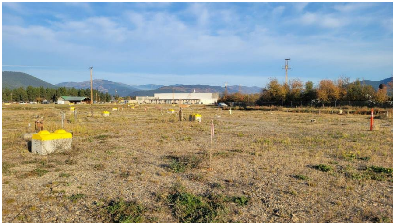
Photograph 18: Area 1 ISB area with Stakes showing new ISB wells to be installed.
