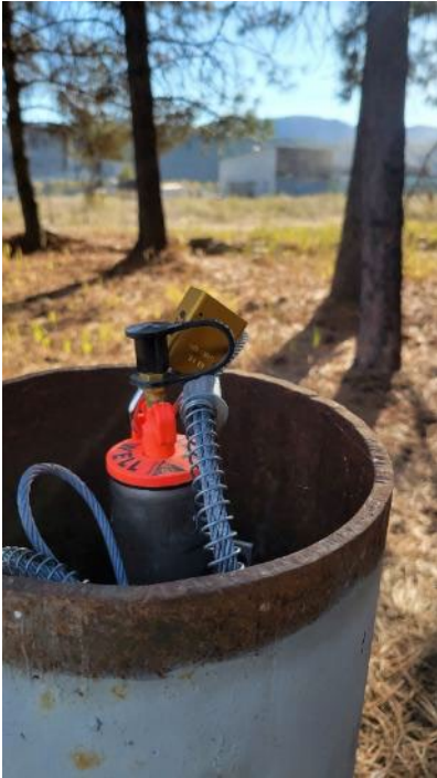
Photograph 24: Area 2 ISB monitoring well with air vent attachment.
