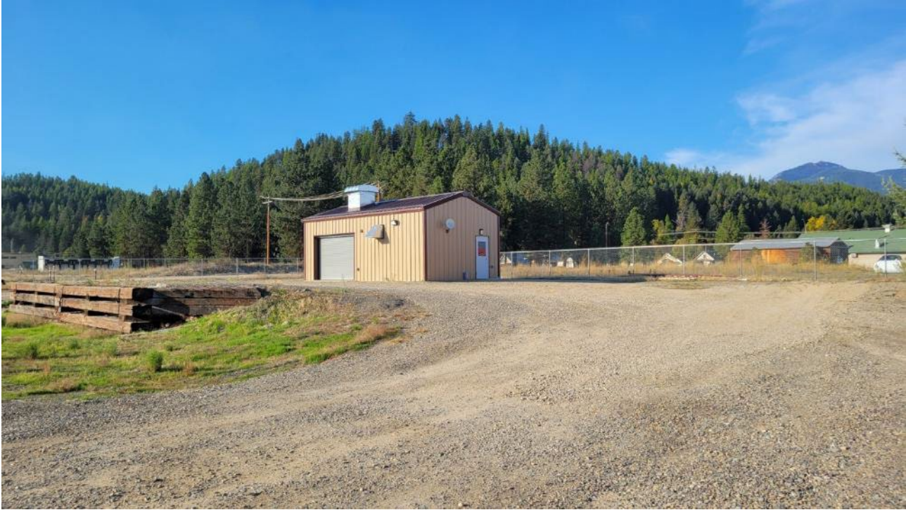
Photograph 21: Area 2 ISB building.
