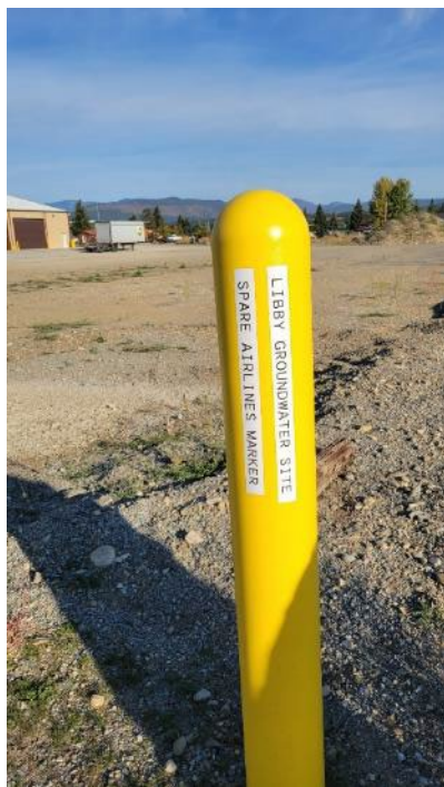
Photograph 19: Area 2 ISB bollard for buried airlines.
