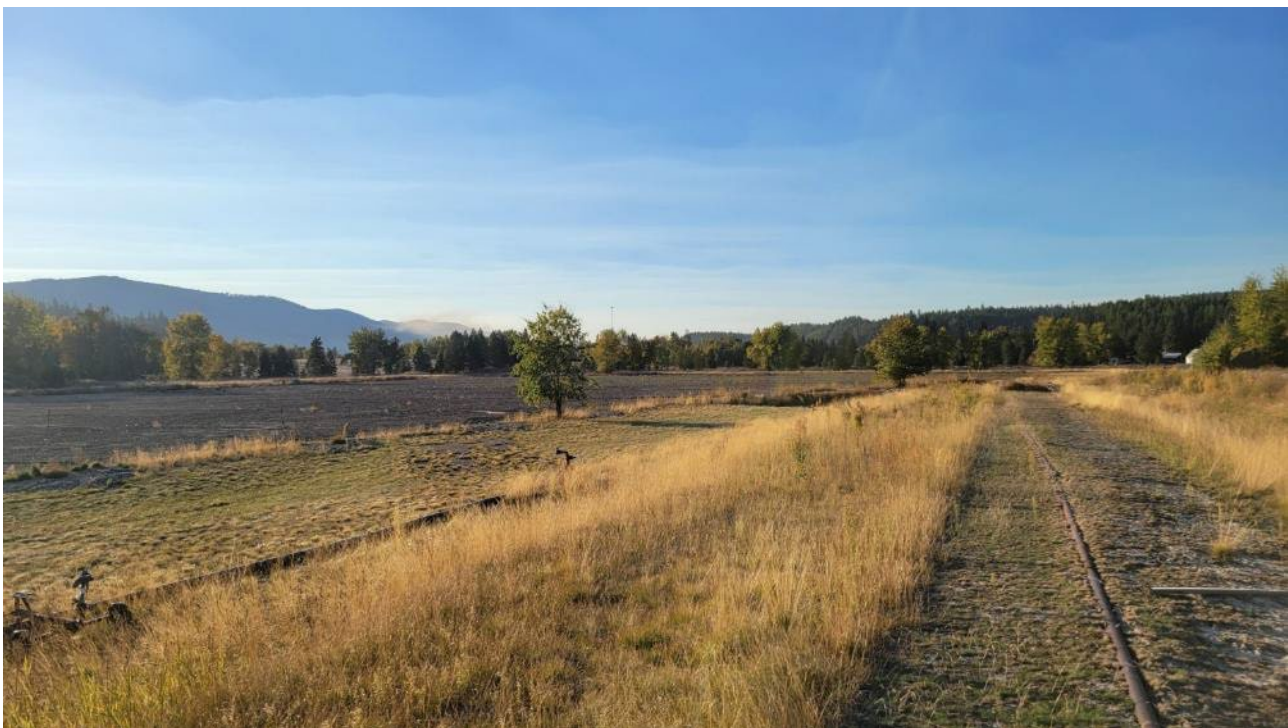
Photograph 13: LTU (piping (on right) and Expanded Landfarm (ELF) on the left
