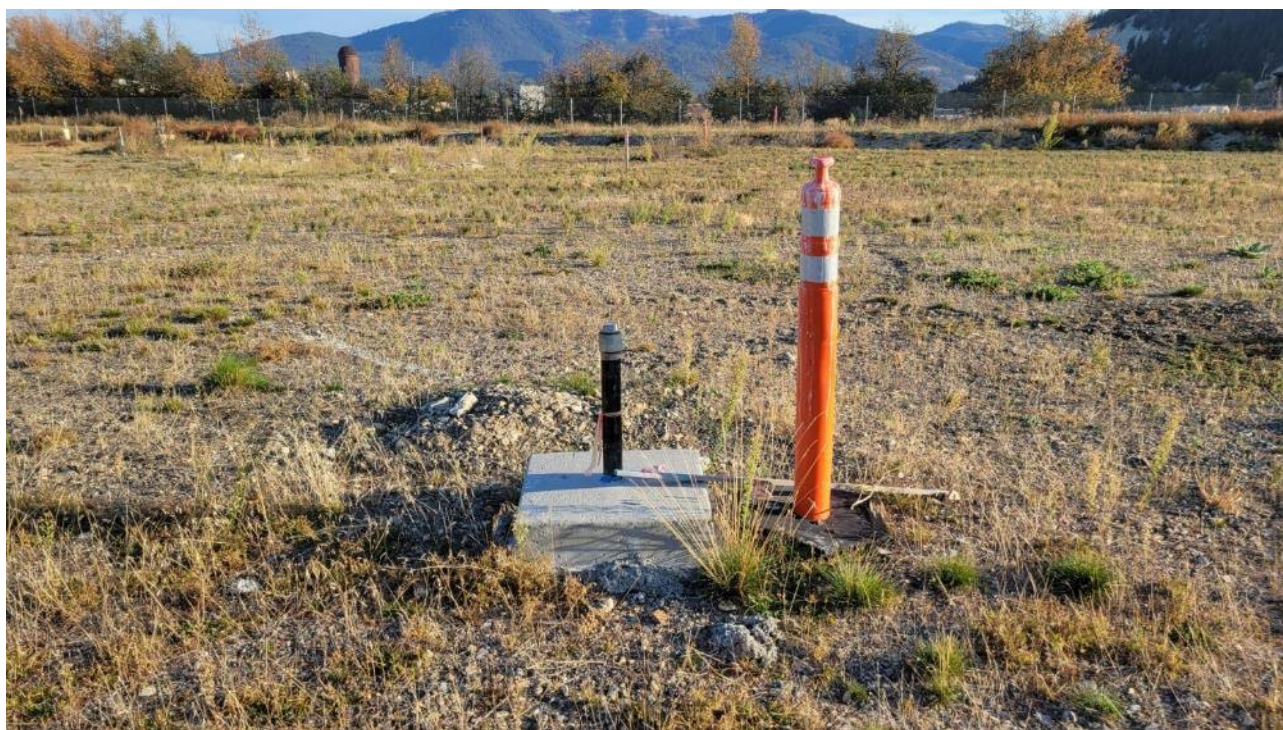
Photograph 17: Area 1 ISB associated well
