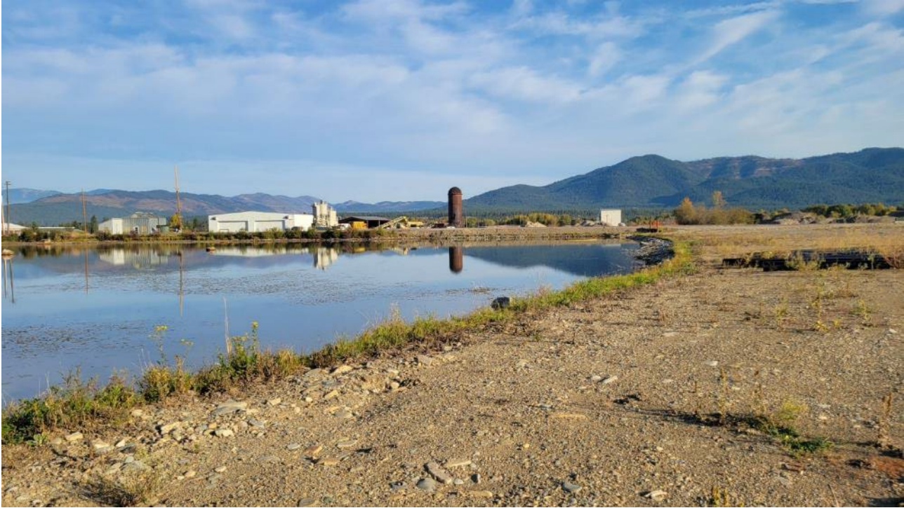
Photograph 15: Southeast corner of fire pond, looking north. Note east bank is graded and de-vegetated.
