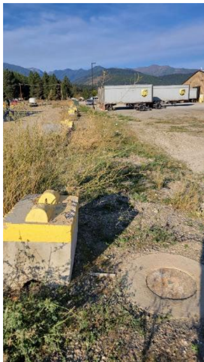
Photograph 20: Area 2 ISB biosparging well curtain line, looking west.
