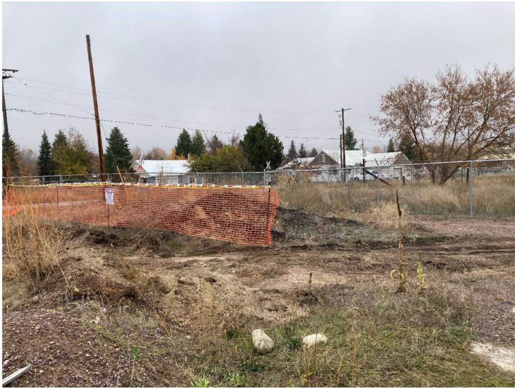
Fencing and signage at OU4 construction project
