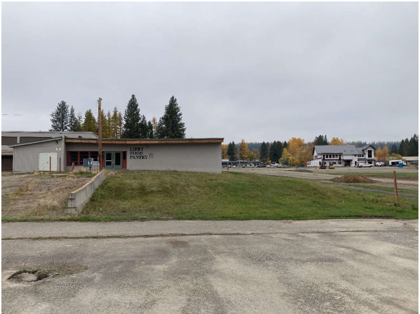
OU4 property scheduled to be demolished and abated as part of redevelopment project
