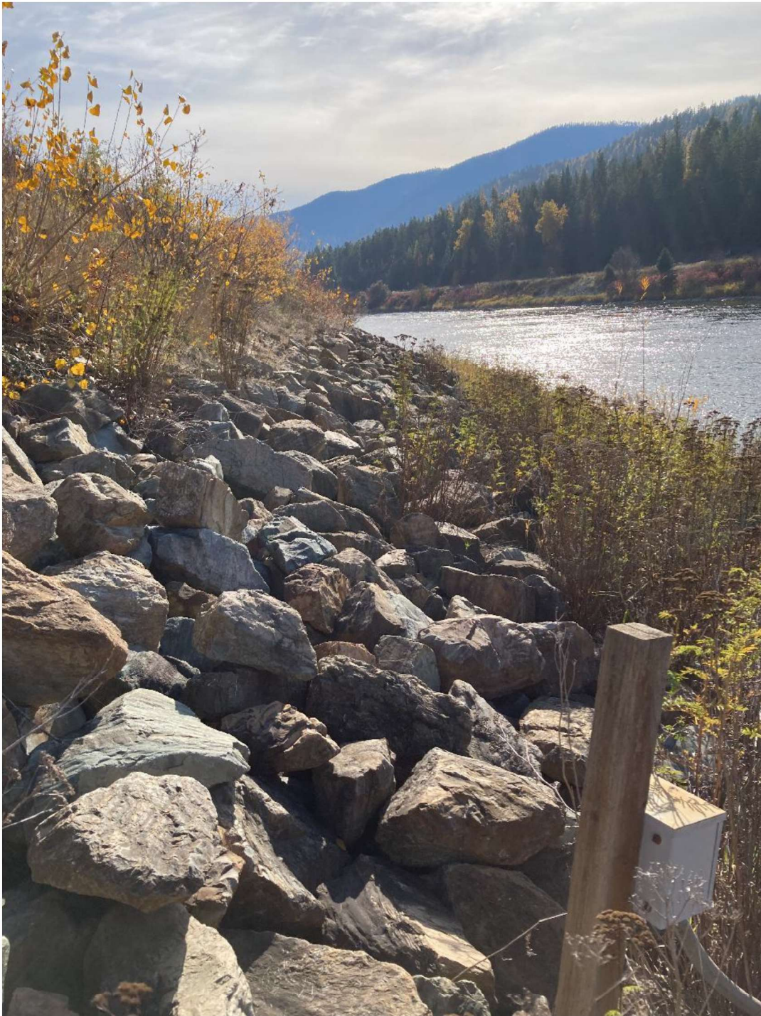
OU2 rip rap along river
