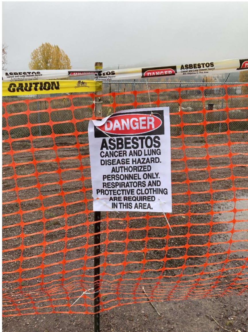
Fencing and signage at OU4 construction project
