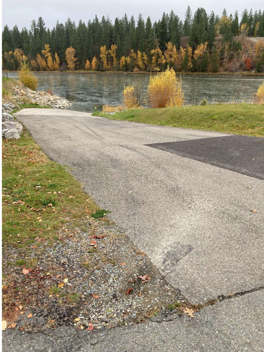
OU1 public boat ramp at Riverfront Park. Minor cover disturbance from users cutting through grass.
