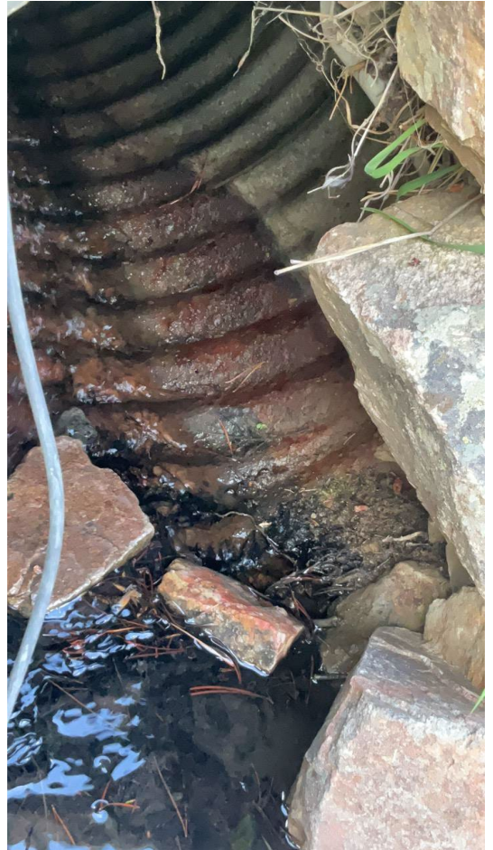
Photo # 110 07-087- AD1 Downstream
