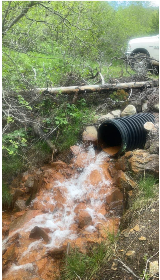
Photo # 98 CSC-117A Upstream
