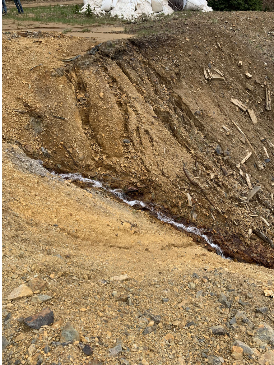
Figure 5: Photograph taken on June 21, 2023, from just below the Silver Dyke Adit looking downslope at the eroded gully.
