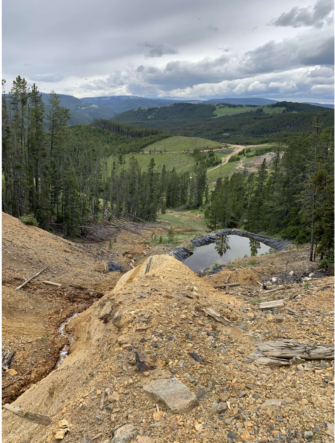
Figure 6: Photographs from June 21, 2023, of Silver Dyke Adit drainage cutting through waste rock below the Adit.
