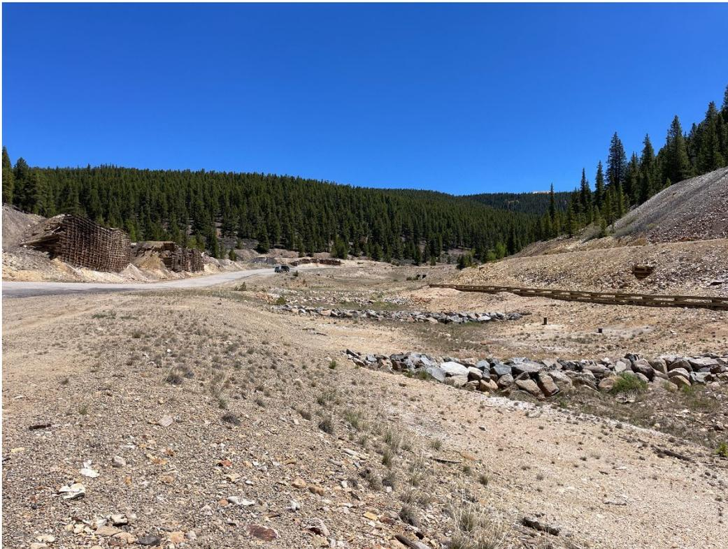
OU4 – View from Helen Waste pile showing cribbing along road and drainage controls
