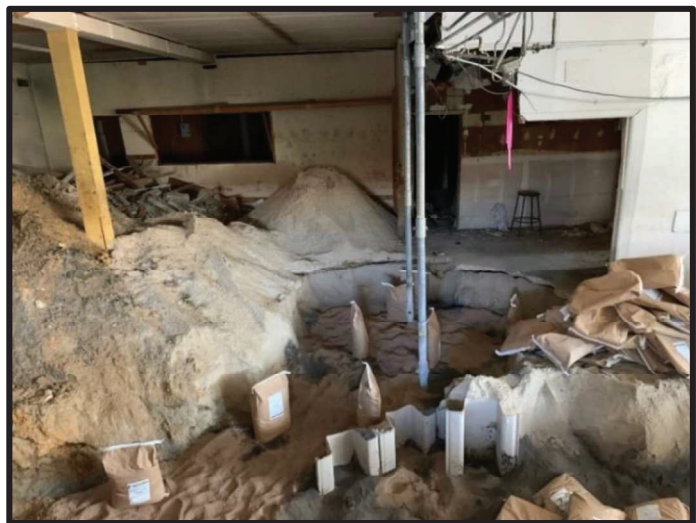
Figure 1: Provect-IR® Applied to Excavation
