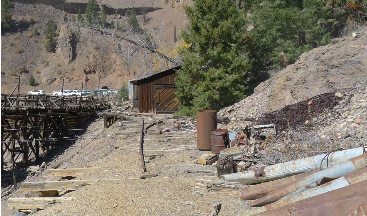
Photo No. 23: South side of generator building/locomotive shed (Resource 6) with mine rail line remnant (Resource 3) in foreground. Camera facing northwest.
