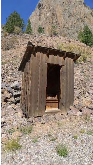
Photo No. 31: Privy (resource 11), looking west.
