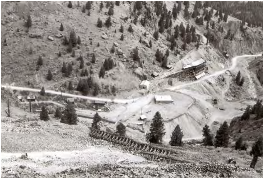
Historic Photo 13. Commodore surface plant, showing south waste rock dump and locomotive charging shed on top, 1999; camera facing southeast. Photo by Eric Twitty from Mining the Amethyst Vein , 105.
