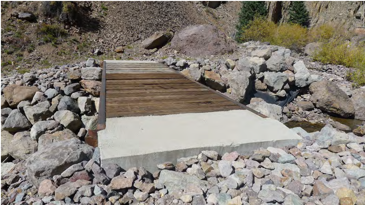
Photo No. 34: Bridge crossing West Willow Creek (Resource 14). Camera facing west.
