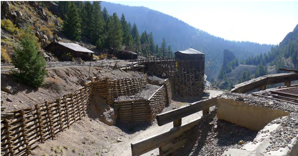
Photo No. 2: View of southeast portion of Commodore surface plant, with county road and waste rock dump cribbing walls in foreground. Commodore ore sorting house and generator/locomotive sheds beyond. Camera facing southeast.
