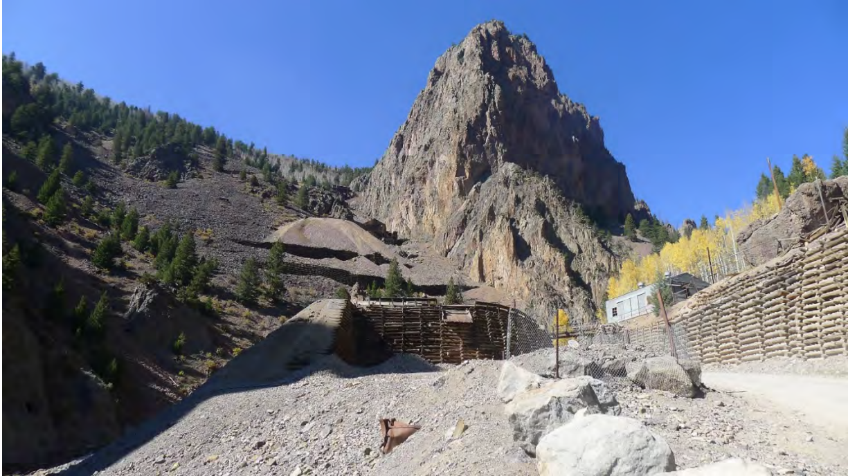
Photo No. 1: Overview of Bachelor-Commodore Mine Complex site, with bedrock pinnacle of Bachelor Mountain at center. Lower and Upper Bachelor tunnel surface plants visible on mountain slope. Commodore Mine waste rock dump and cribbing walls in foreground. Camera facing northwest.
