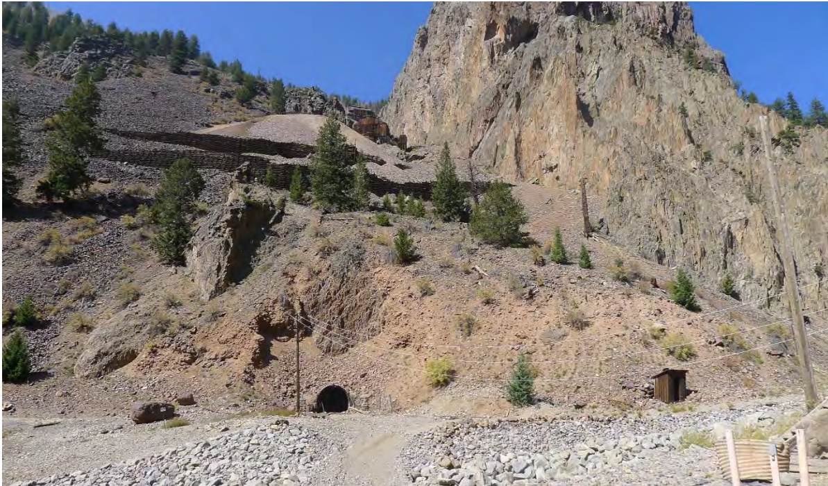
Photo No. 3: View of Commodore tunnel portal and Lower Bachelor waste rock dump and ore sorting house beyond up mountain side, with rockwork lining of West Willow Creek in foreground. Camera facing northwest.
