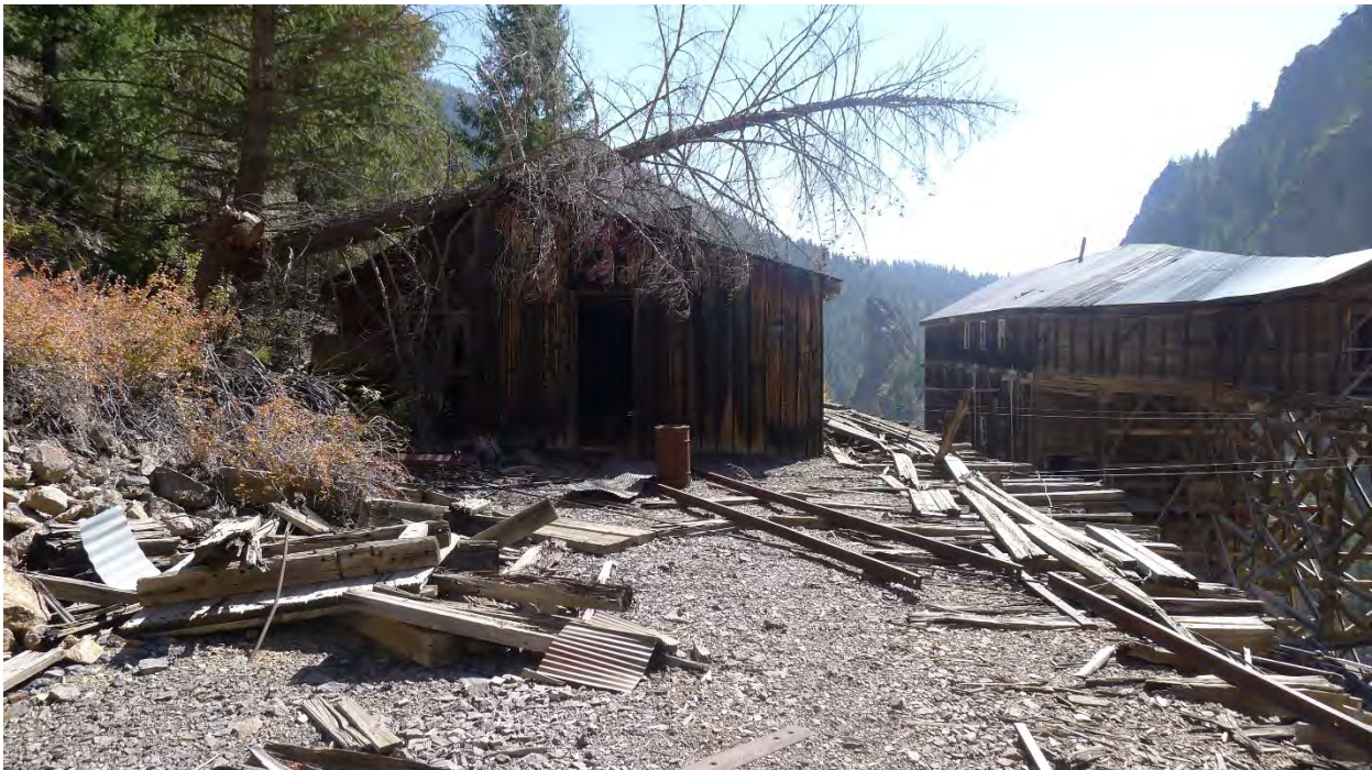
Photo No. 22: North side of generator building/locomotive shed (Resource 6). Camera facing southeast.
