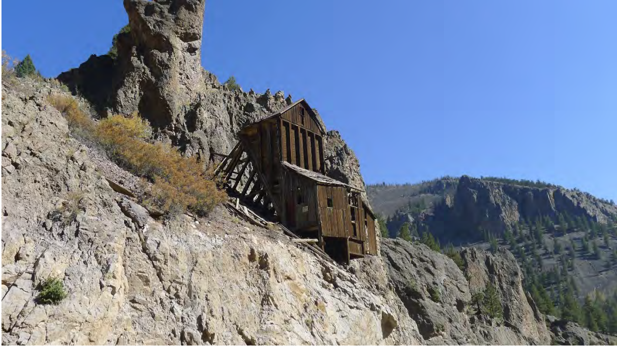
Photo No. 11: West and north sides of ore sorting house (Resource 2). Camera facing east.
