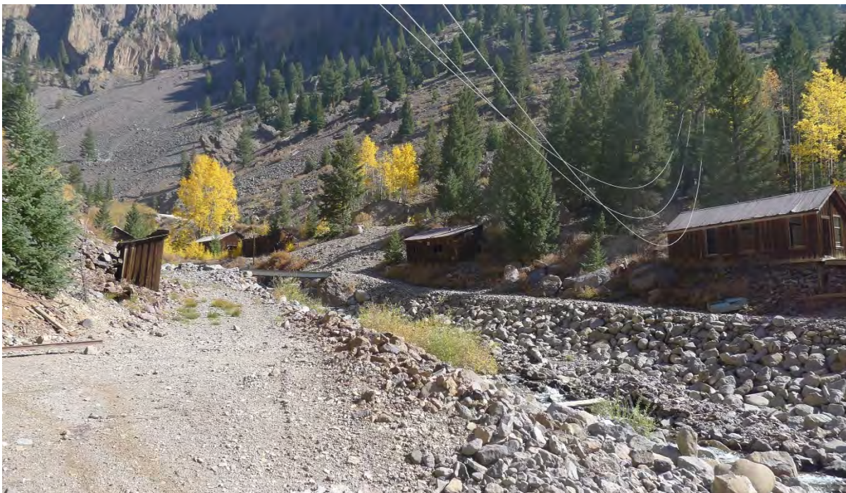
Photo No. 4: View of northern section of Commodore Tunnel No. 5 surface plant; office, compressor house, bridge, shop and compressor house (Resources 13-17) from right to left on opposite side of creek bed. Camera facing north.
