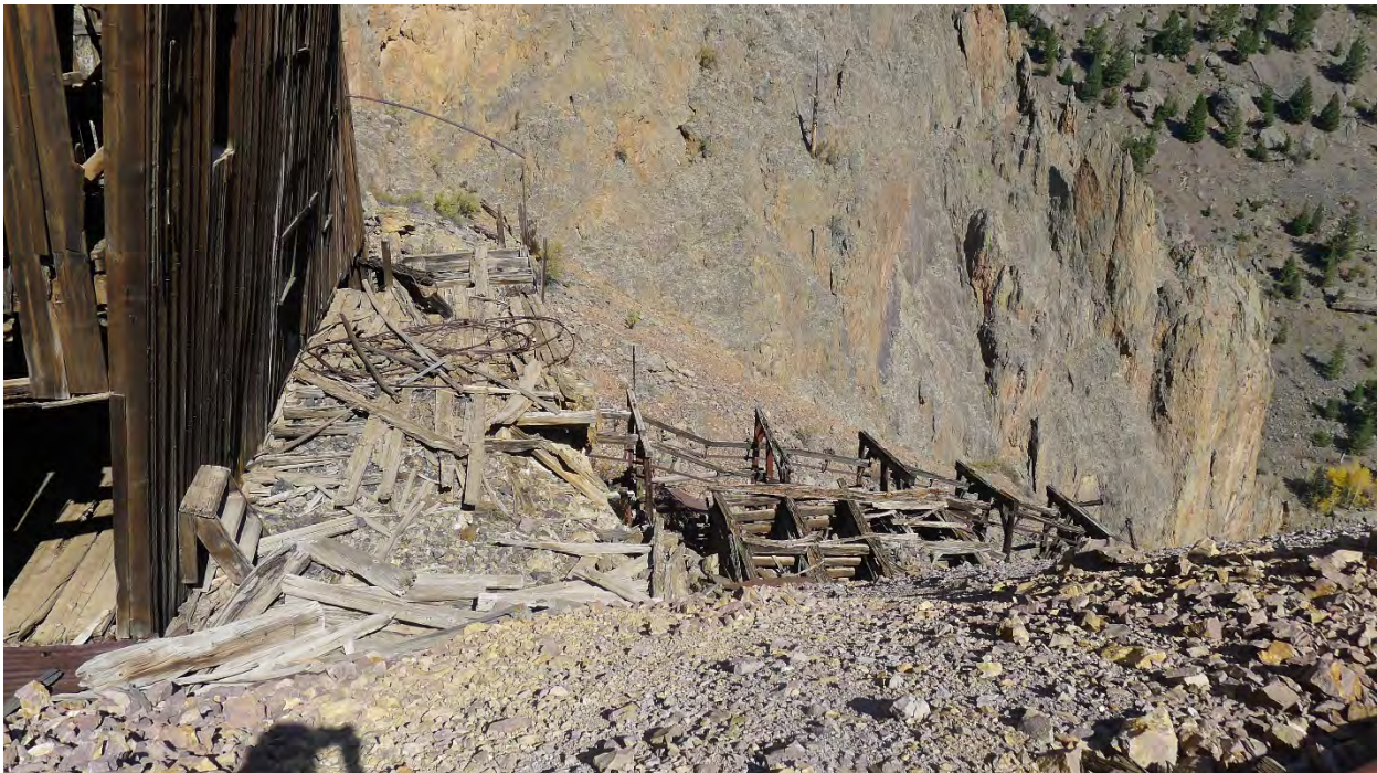
Photo No. 58: Aerial tramway framework at east side of ore sorting house and aerial tramway terminal. Camera facing north.
