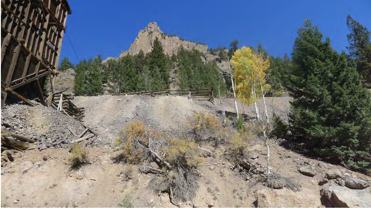
Photo No. 15: View from road looking up toward south end of southeast waste rock dump (Site Feature 1) on mountainside. Camera facing northeast.
