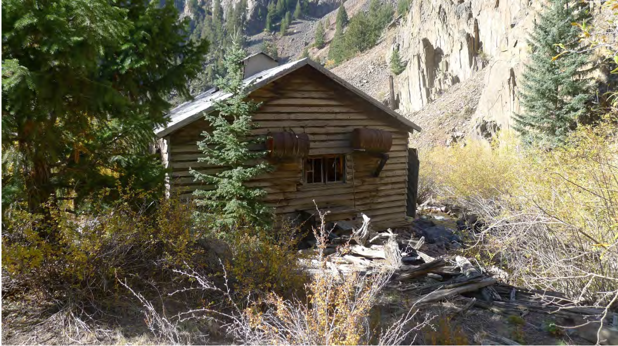
Photo No. 43: North side of compressor house. Camera facing south.
