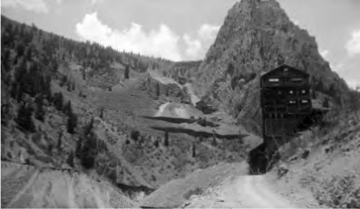
Historic Photo 5. Photograph by Muriel Sibell Wolle, circa 1955, showing Lower and Upper Bachelor waste rock dumps and surface plants on mountainside, with 1940 Commodore Ore Sorting House in right foreground. Photo courtesy of Denver Public Library Special Collections, call number X-5152.
