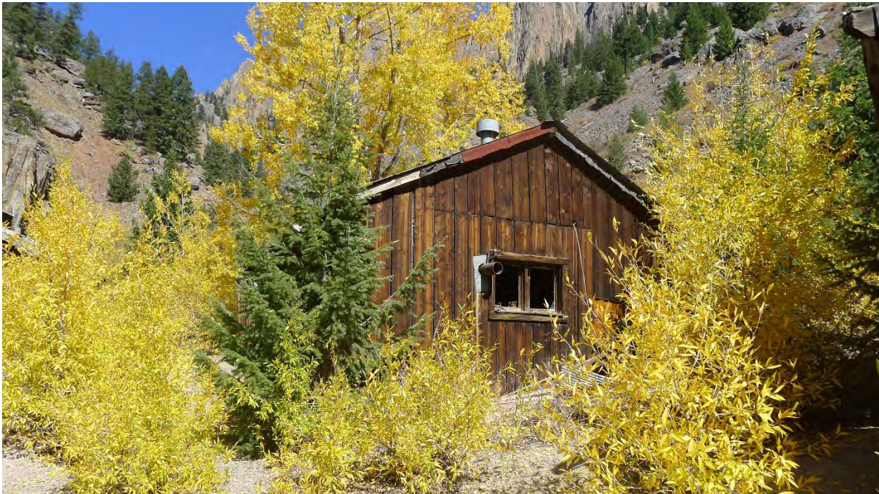
Photo No. 36: South side of compressor house (Resource 17). Camera facing north.
