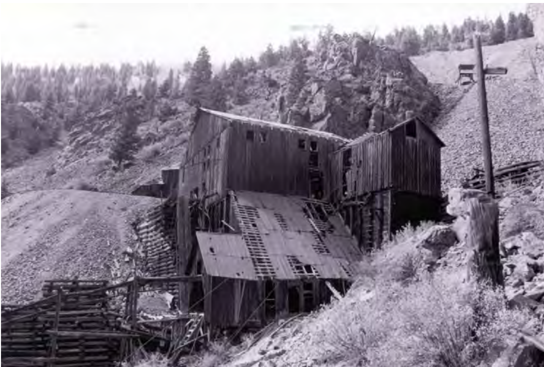
Historic Photo 11. Lower Bachelor Ore Sorting House with Aerial Tramway Terminal, 1999; camera facing southwest. Photo by Eric Twitty from Mining the Amethyst Vein , 79.
