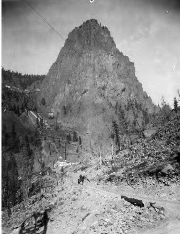
Historic Photo 1. Circa 1895 photo showing wagon road (now County Road 503) passing through West Willow Creek canyon, with surface plants of the Commodore No. 5, Lower and Upper Bachelor tunnels in distance. Powerhouse and other buildings at Commodore plant removed prior to 1930s. Photo courtesy of Denver Public Library Special Collections, call number X-61954.
