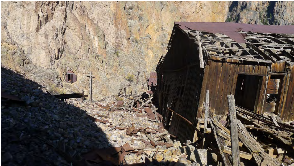
Photo No. 60: West side of ore sorting house and aerial tramway terminal with debris and artifacts on adjacent waste rock. Note cables of aerial tramway to Upper Bachelor are still suspended. Explosives magazine (Resource 30) in distance at left in bedrock face. Camera facing north.
