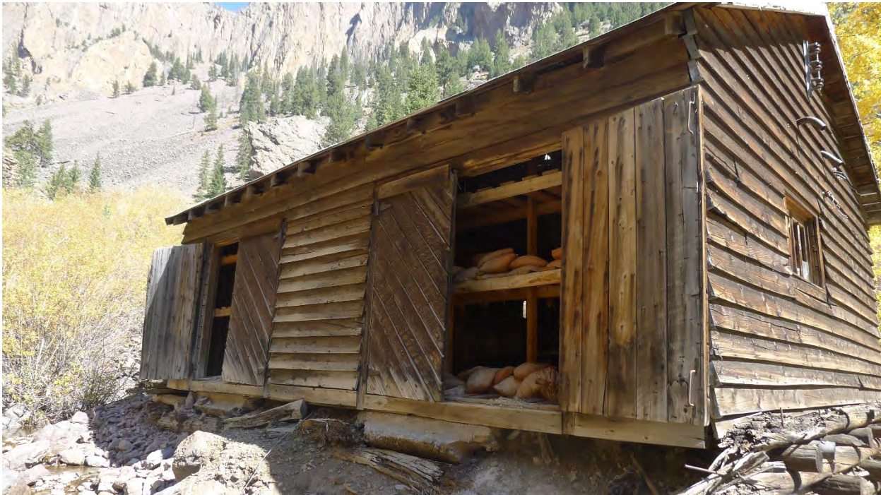
Photo No. 42: West side of compressor house. Camera facing northeast.
