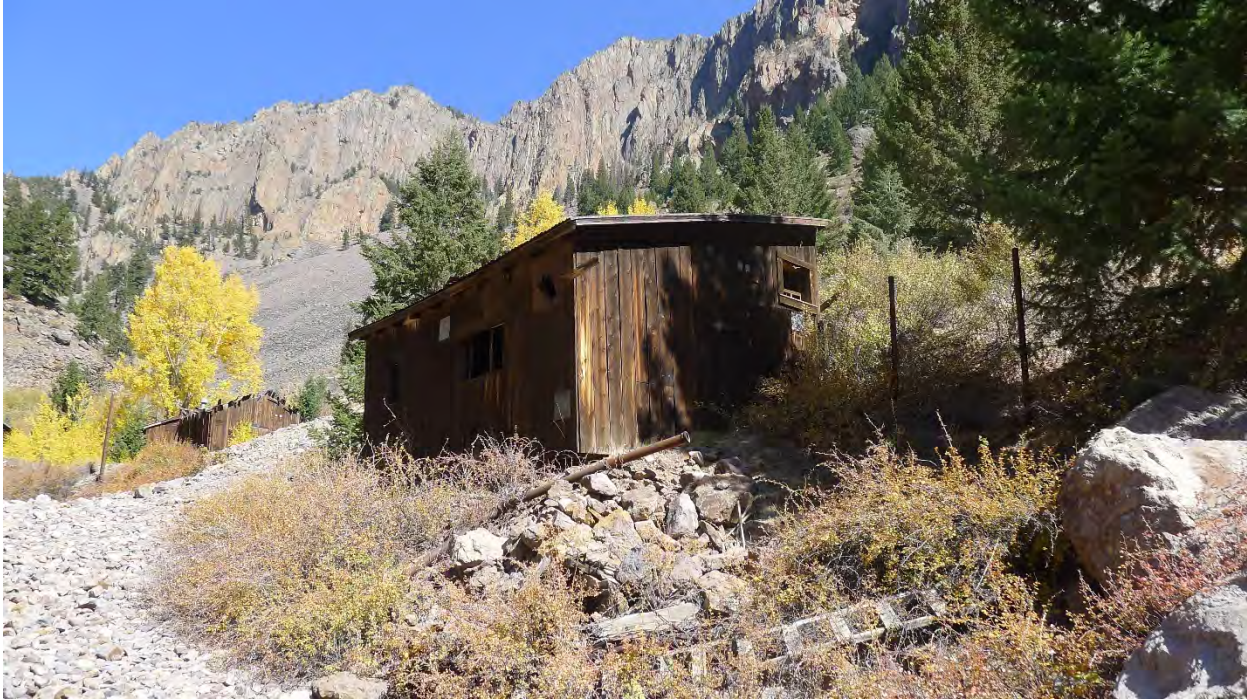
Photo No. 33: South and west sides of compressor house (Resource 13). Camera facing north.
