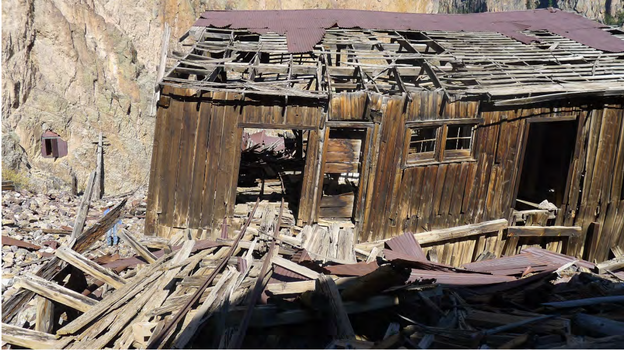
Photo No. 59: Detail of south side of ore sorting house and aerial tramway terminal with view to interior along ore cart rail. Explosives magazine (Resource 30) in distance at left in bedrock face. Camera facing north.
