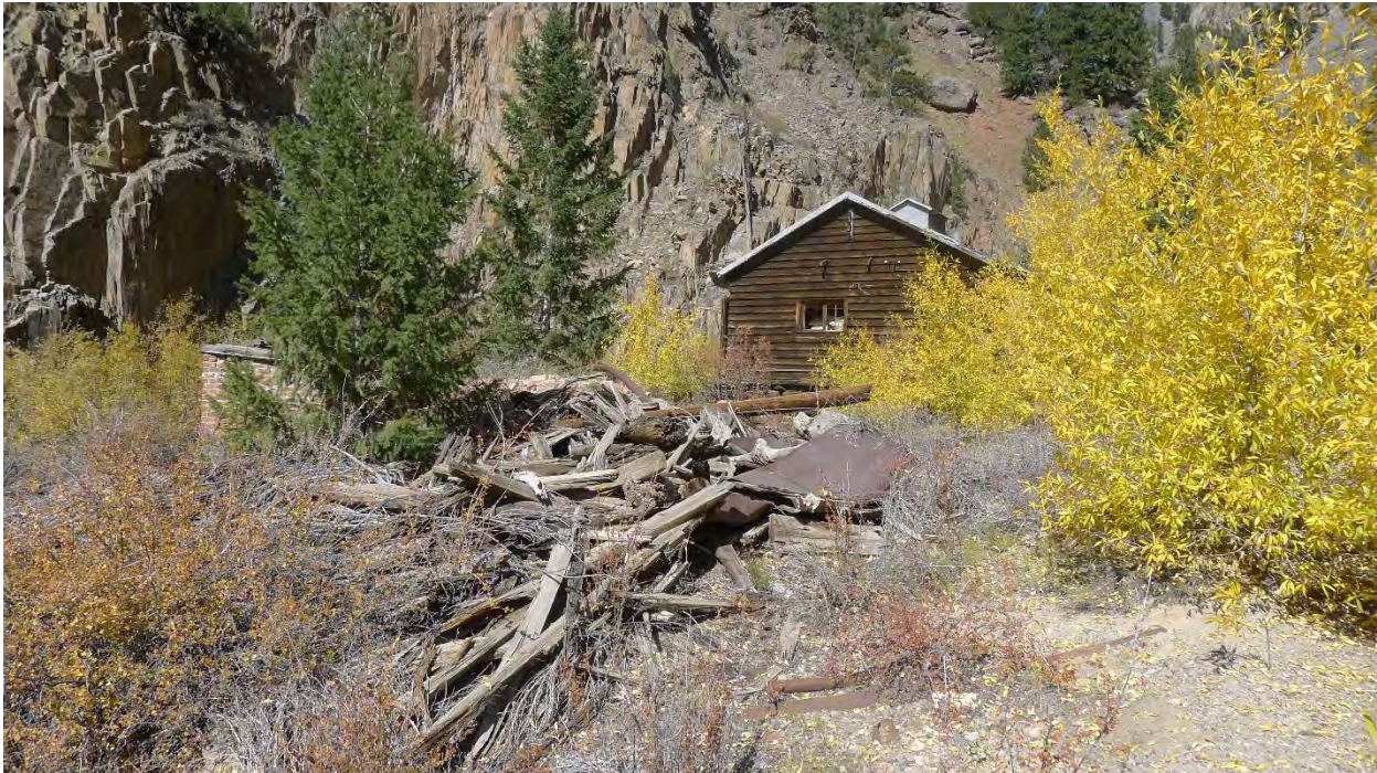
Photo No. 38: View of powerhouse ruins (Site Feature 3) with debris on top and boiler setting remnant to left. Compressor house (Resource 19) beyond. Camera facing north.
