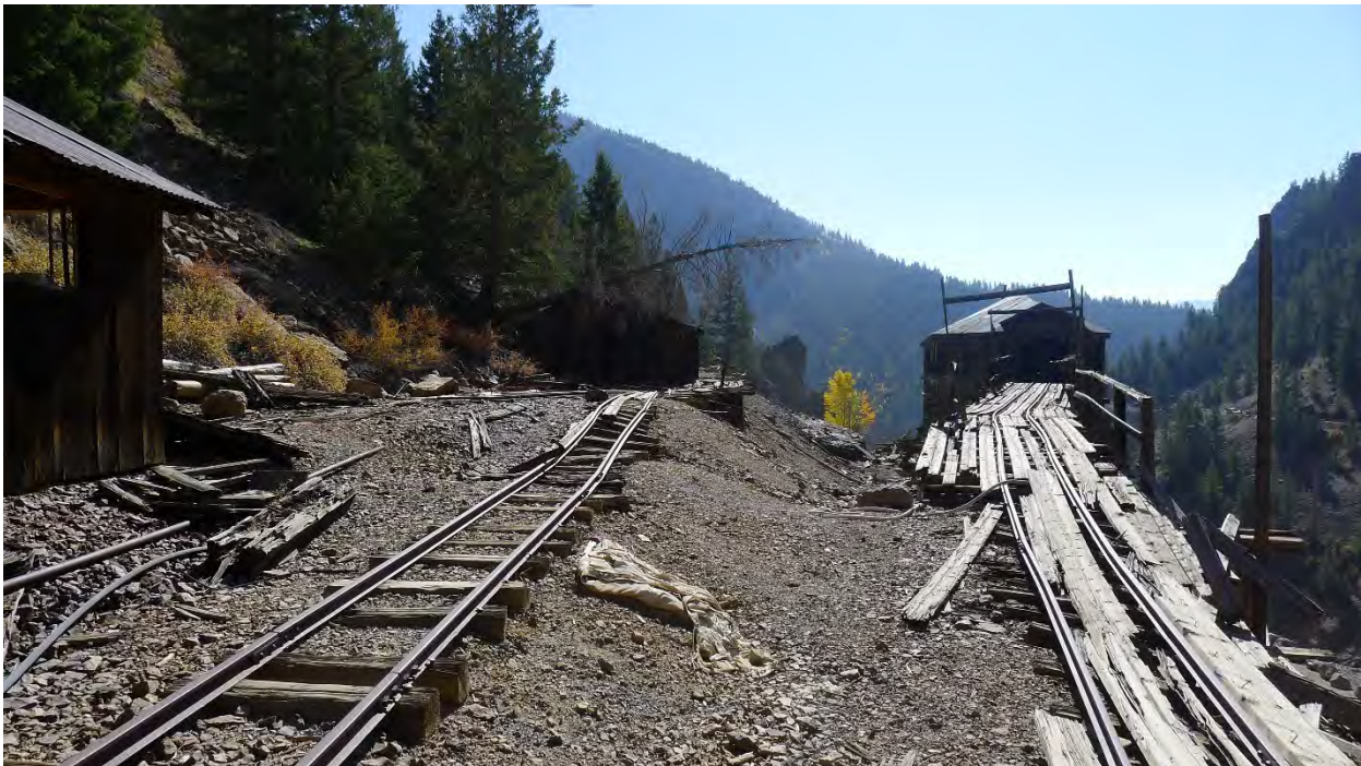
Photo No. 14: View southeast toward Commodore ore sorting house (Resource 4) at right and two generator buildings/locomotive sheds (Resources 5-6) at left.
