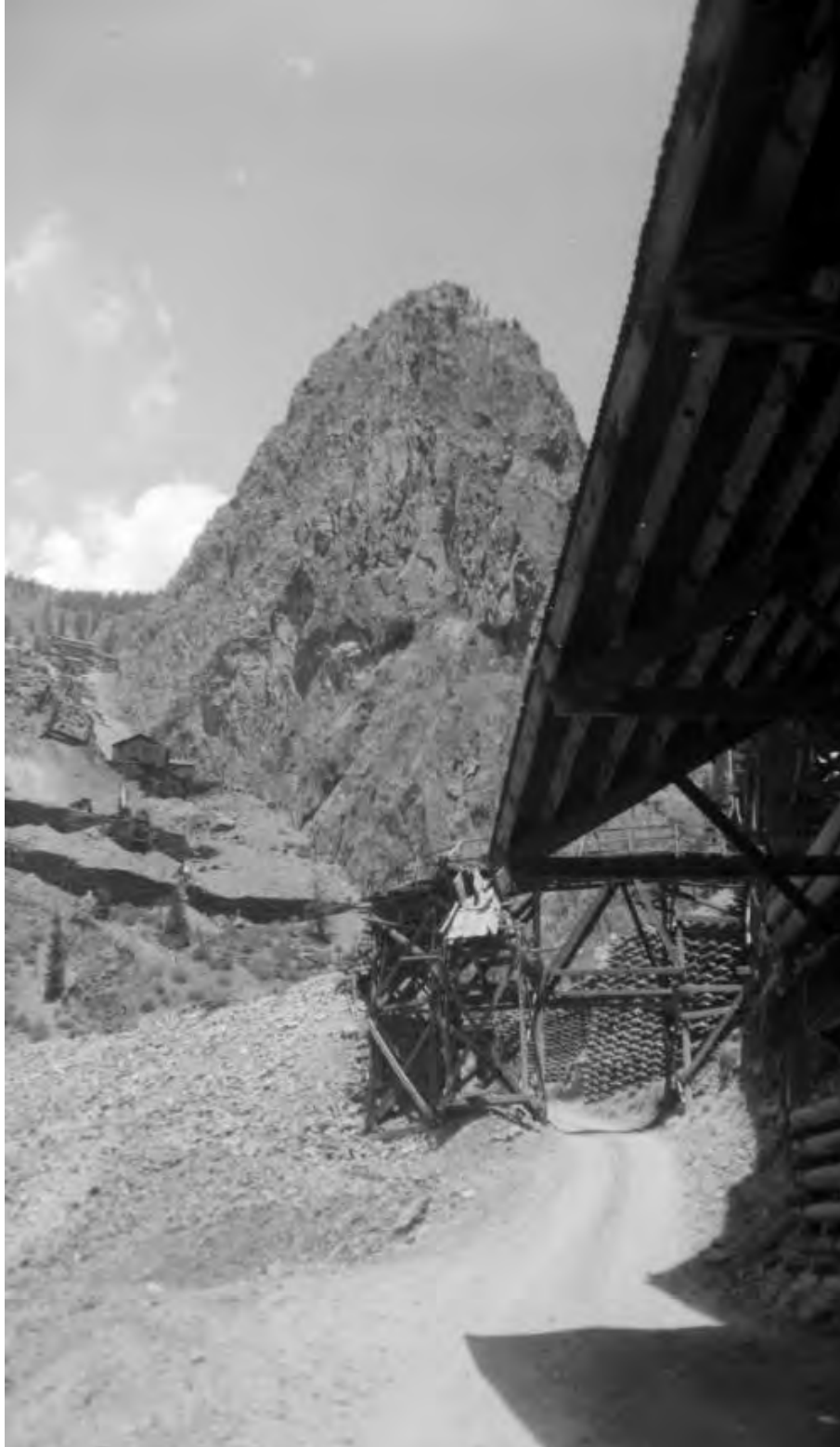
Historic Photo 9. Photograph by Muriel Sibell Wolle, circa 1955, view northwest toward trestle carrying mine rail spur over road from tunnel portal to ore sorting house (in foreground). Photo courtesy of Denver Public Library Special Collections, call number X-5153.
