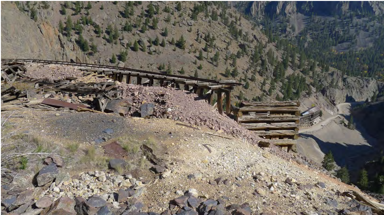
Photo No. 52: Privy pit cribbing (Resource 26) with mine rail line remnant (Resource 27) at left. Camera facing southeast.
