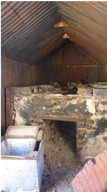
Photo No. 50: Interior of dynamite thaw house (Resource 24), with thaw box on floor. Camera facing southwest.
