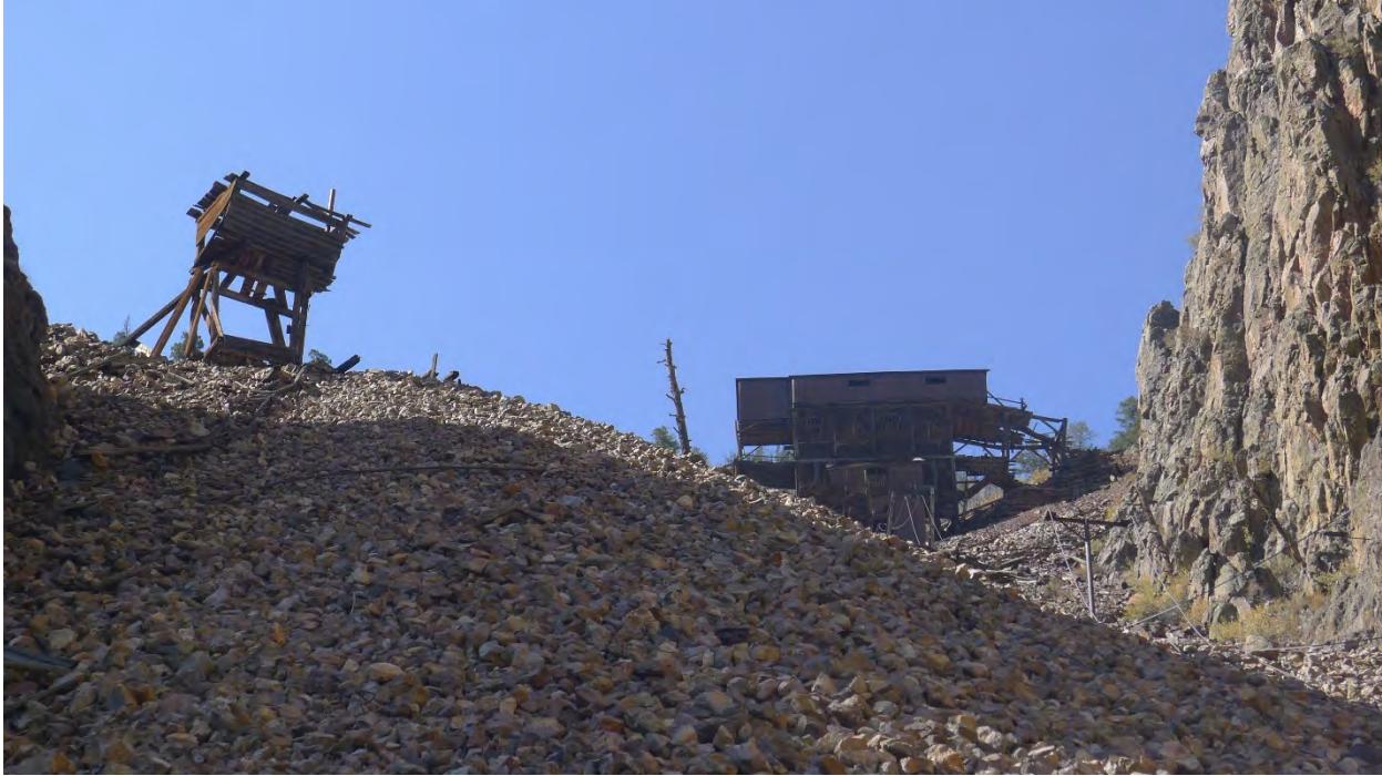
Photo No. 67: Detail of ore bin (Resource 32) at left and Upper Bachelor ore sorting house and aerial tram terminal (Resource 39) beyond at right. Camera facing west.
