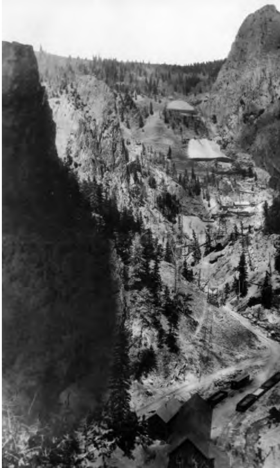
Historic Photo 3. Circa 1920 view of southeast flank of Bachelor Mountain with Commodore and Lower and Upper Bachelor surface plants ascending up mountainside. Aerial tramways bring loads of ore to railroad terminus in foreground. Photo courtesy of Denver Public Library Special Collections, call number X-61954.
