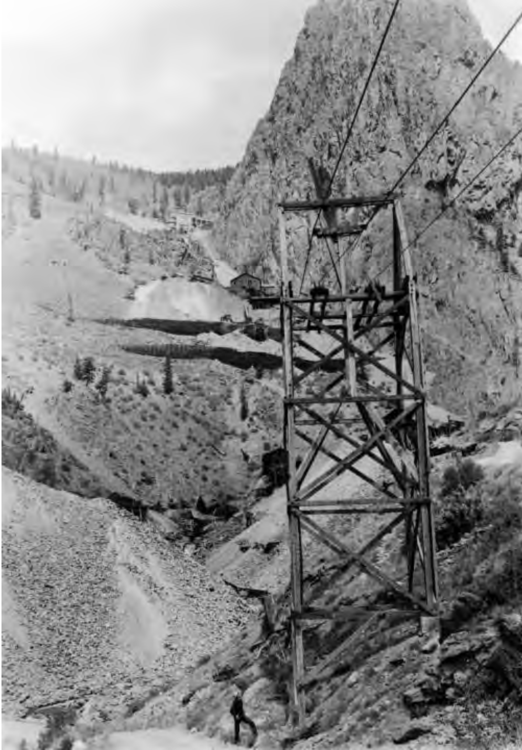
Historic Photo 4. Photograph showing aerial tramway tower in foreground of West Willow Creek and Bachelor Mine surface plants on mountainside. The 1942 photograph is by Theodore Fisher. Photo courtesy of Denver Public Library Special Collections, call number X-61937.
