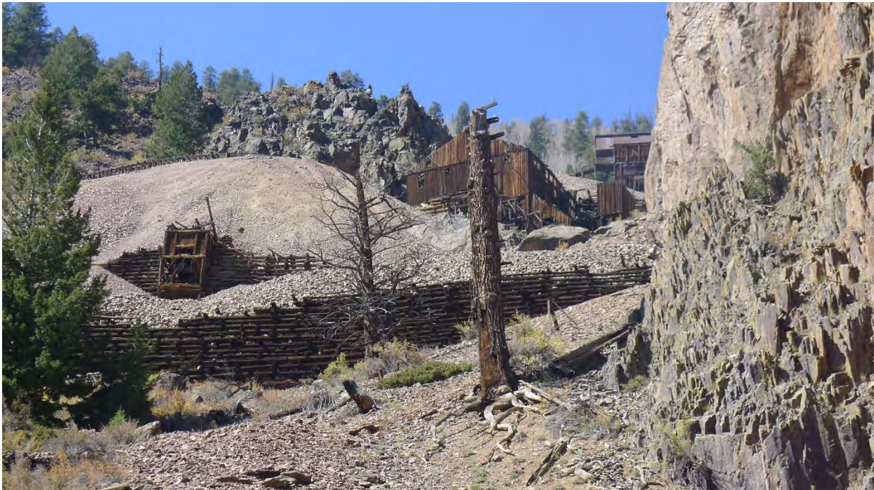
Photo No. 44: Close-up of Lower Bachelor waste rock dump with lower cribbing wall (Site Feature 4) in foreground and ore bin and aerial tram terminal (Resource 20) at left at upper cribbing wall. Lower Bachelor ore sorting house and aerial tram terminal (Resource 29) beyond near bedrock outcrop, and Upper Bachelor ore sorting house (Resource 39) in distance at right. Camera facing west.
