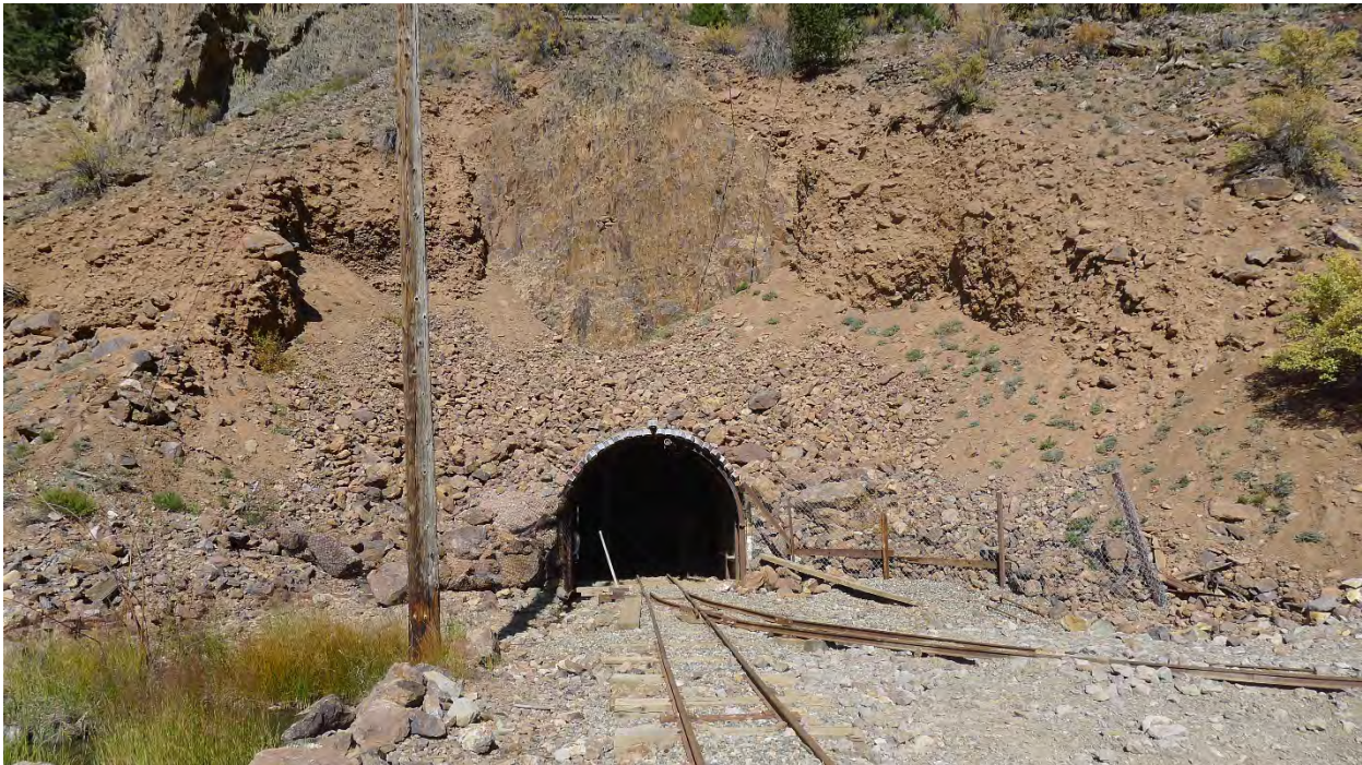
Photo No. 30: Commodore Tunnel Portal (Resource 10). Camera facing west.
