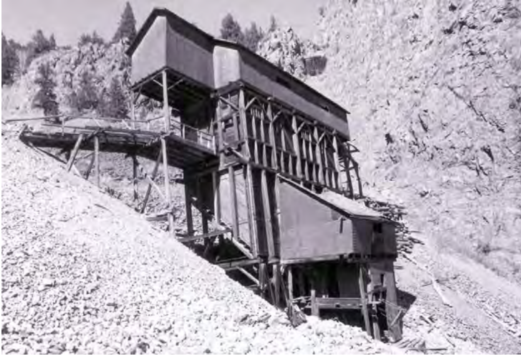
Historic Photo 12. Upper Bachelor Ore Sorting House, 1999; camera facing north. Photo by Eric Twitty from Mining the Amethyst Vein , 87.
