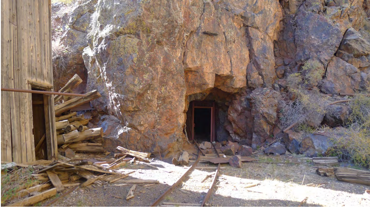
Photo No. 65: Lower Bachelor Tunnel Portal (Resource 31) in bedrock outcrop. Camera facing west.
