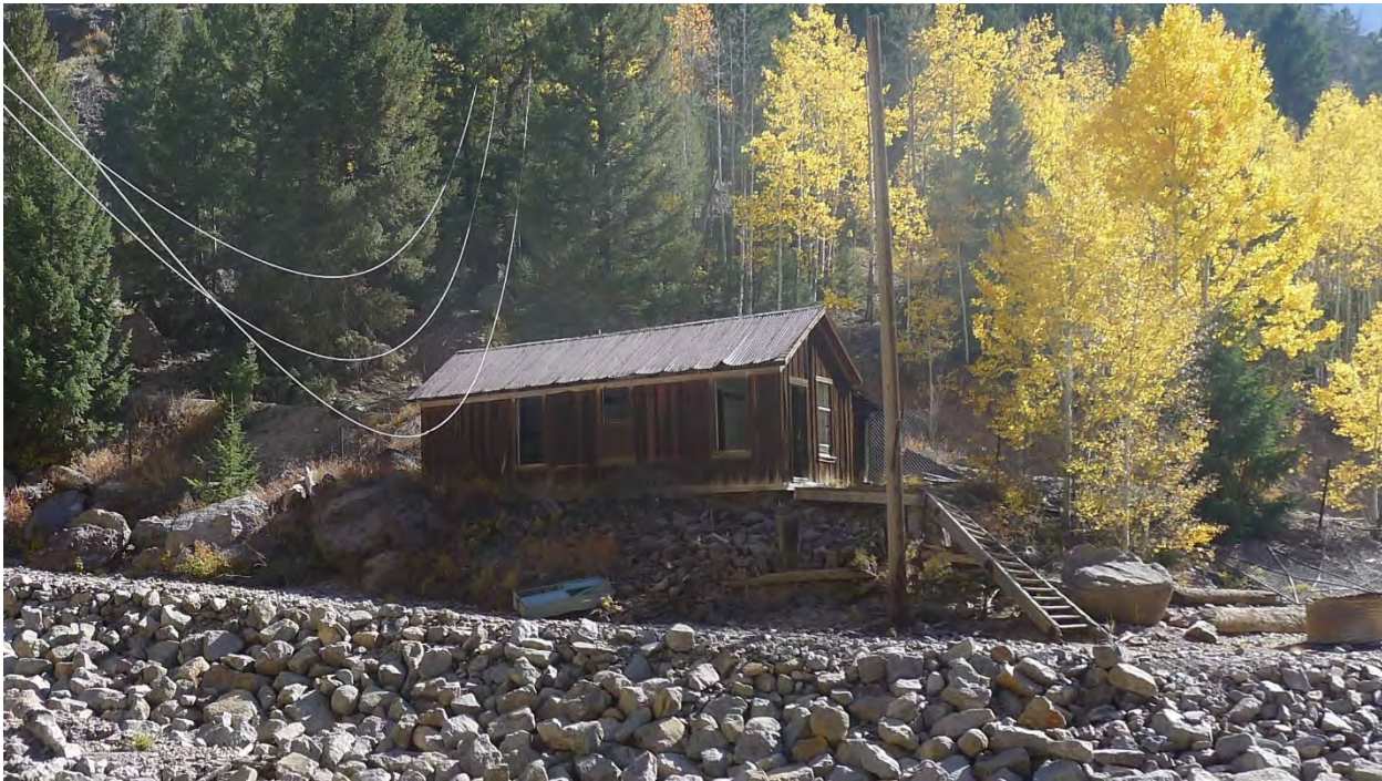
Photo No. 32: West and south sides of office (Resource 12). Camera facing east.
