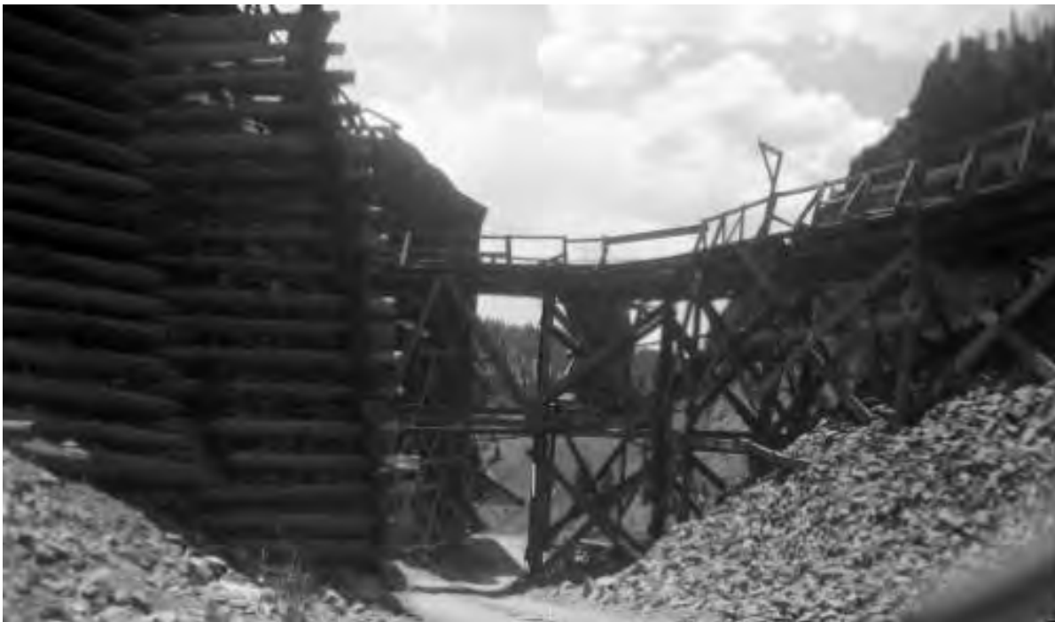
Historic Photo 8. Photograph by Muriel Sibell Wolle, circa 1955, view south toward trestle carrying mine rail spur over road from tunnel portal to ore sorting house; rail line no longer extant. Photo courtesy of Denver Public Library Special Collections, call number X-5151.
