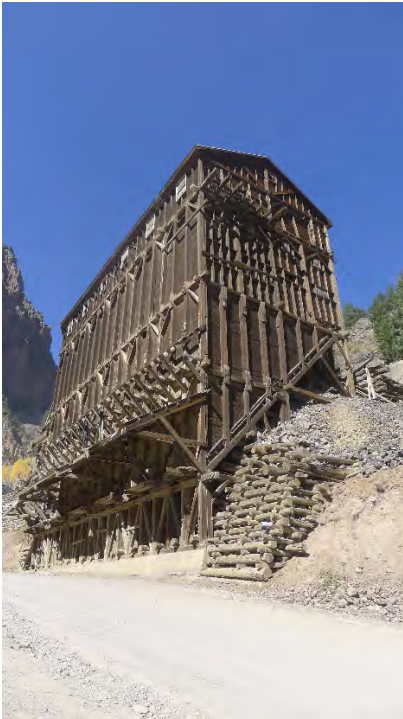
Photo No. 17: Commodore ore sorting house, south and west sides. Camera facing north.
