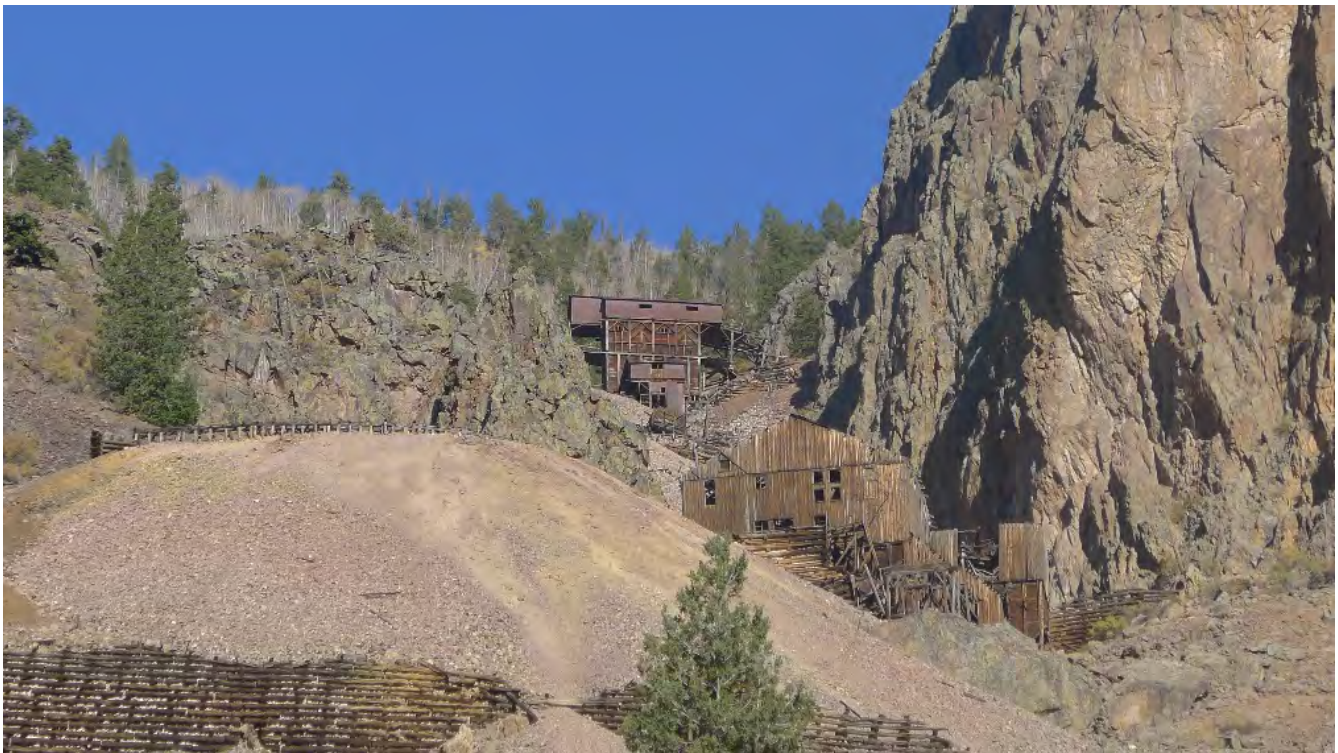
View of the cribbing and Lower and Upper Ore Sorting House and Aerial Tramway
