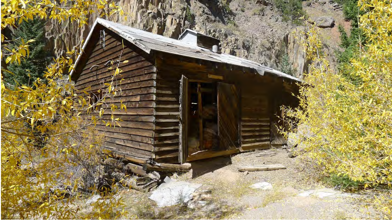
Photo No. 41: South and east sides of compressor house (Resource 19). Camera facing northwest.
