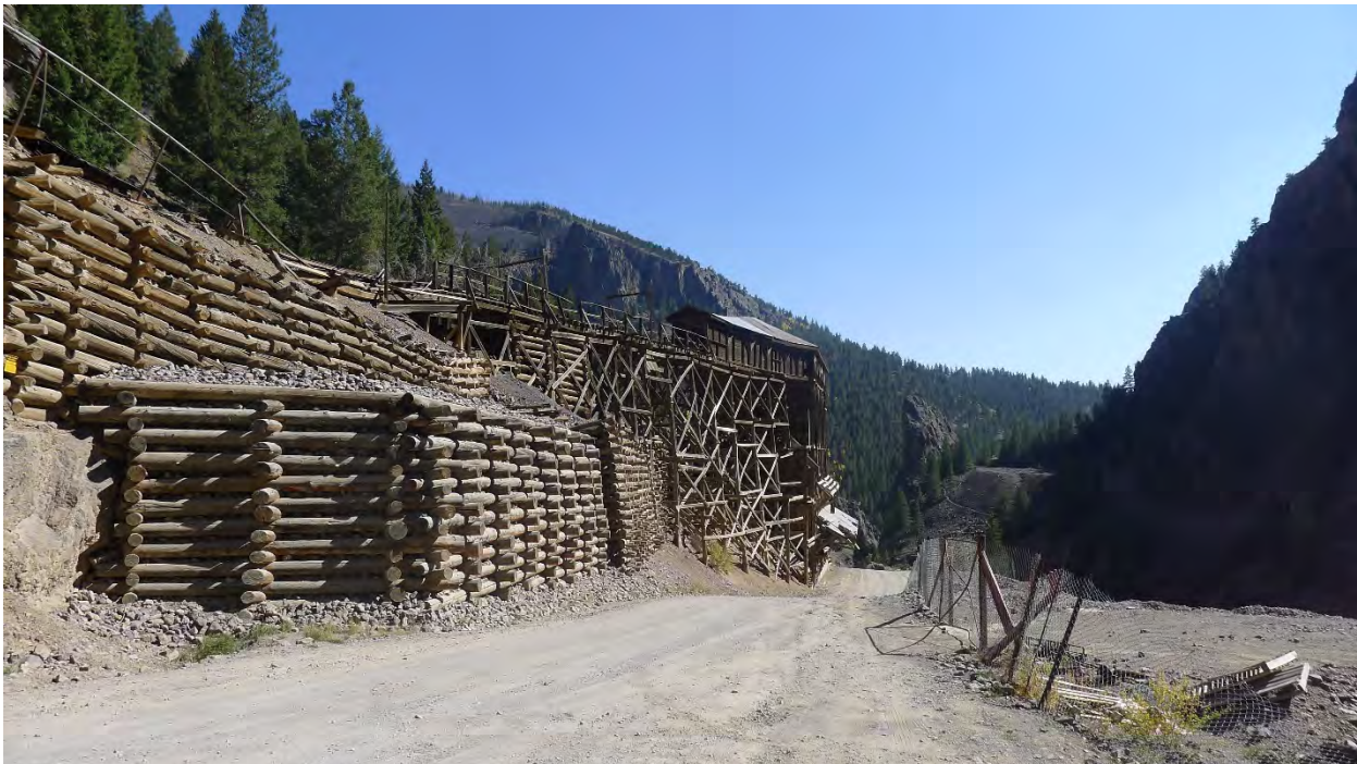
Photo No. 16: View of cribbing walls of southeast waste rock dump (Site Feature 1) with road in foreground and ore sorting house with trestle (Resource 4) in distance. Camera facing southeast.
