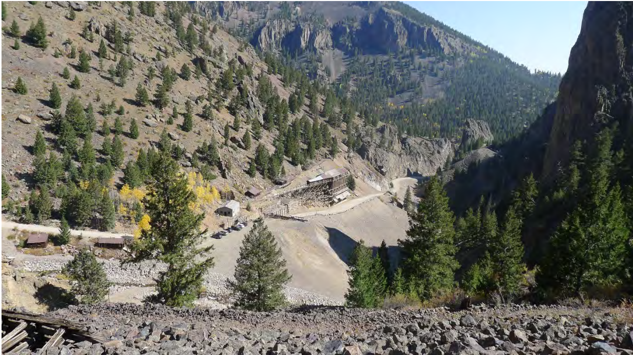
Photo No. 9: View of southeast section of Commodore surface plant from side of Bachelor Mountain; note recontoured waste rock dump at parking area and along road. Camera facing southeast.
