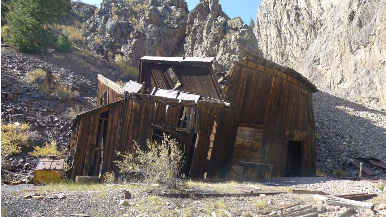
Photo No. 55: East side of shop (Resource 28). Camera facing west.
