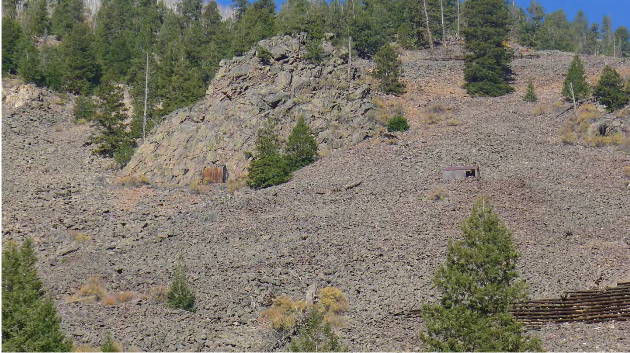
Photo No. 47: View of explosives magazine (Resource 22, at left) and dynamite thaw house (Resource 24) on scree slope. Camera facing west.
