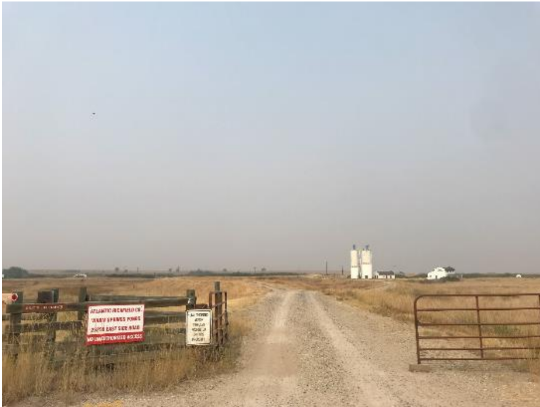
Entrance to lime treatment facility
