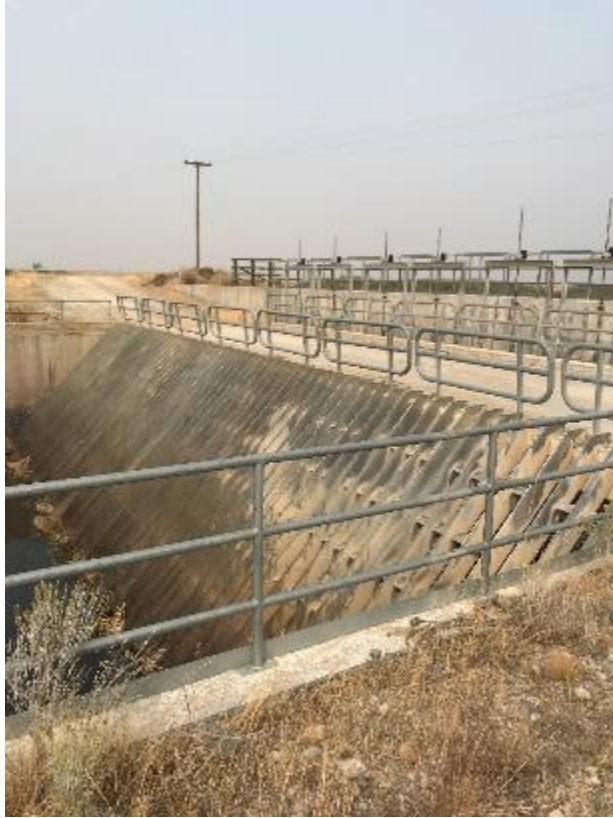
Pond 3 inlet structure
