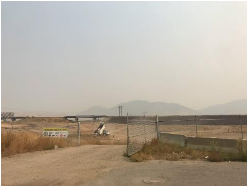
Parrot Tailings removal area
