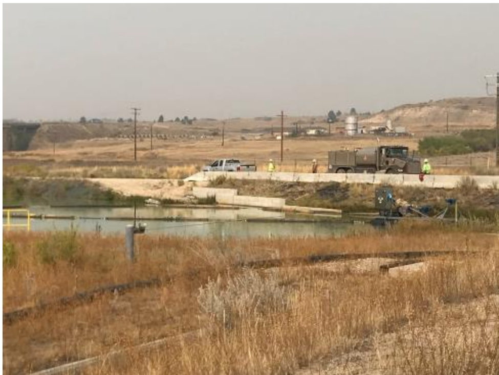
Dredging operation at Butte Treatment Lagoons
