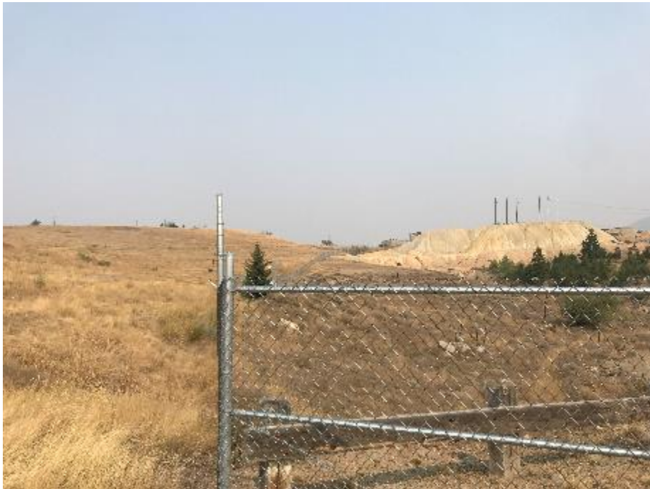
Green Mountain Catch Basin
