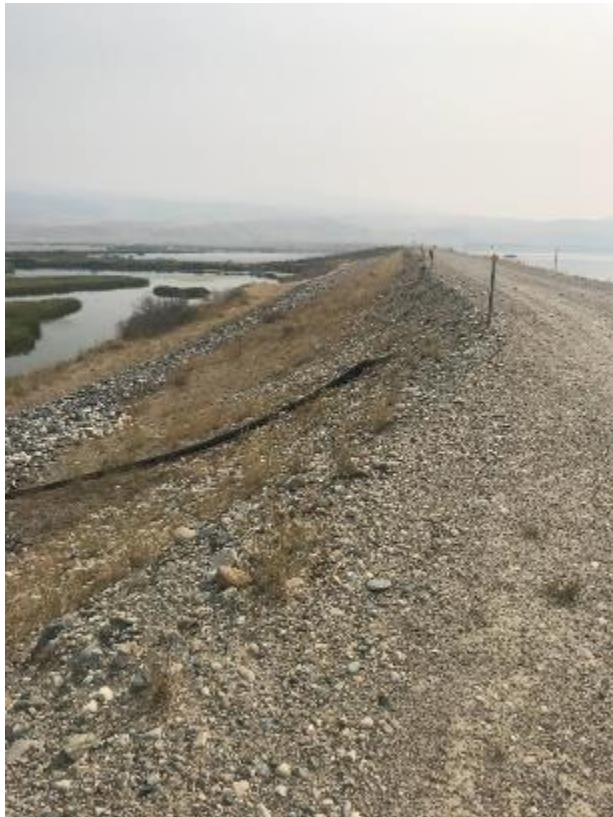
Berm from Pond 3 to Pond 2
