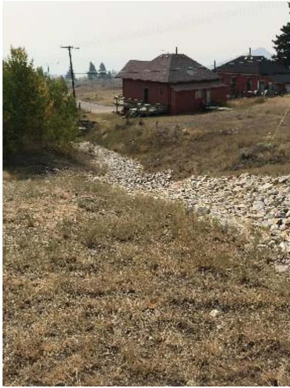
BRES site with stormwater management features, Alice diversion ditch
