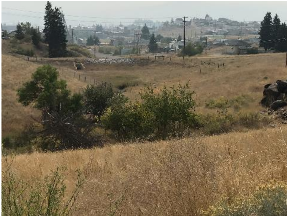
BRES site with stormwater management features, Buffalo South
