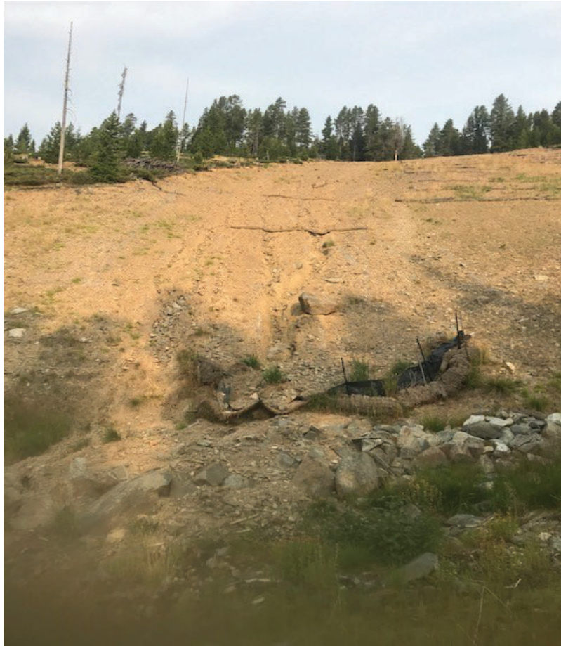
Figure 2: Surface impoundment contaminated with mine waste shows no vegetation establishment and is severely eroded into No Name Creek.
