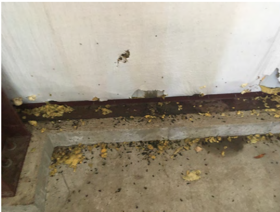
Treatment chemical remaining in the Groundwater Recovery System building after decommissioning of the WTP. Chemicals will be mixed with kitty litter to solidify and chemicals will be disposed in the local landfill.
