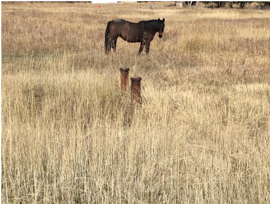
Monitoring wells 27A and B which are the furthest downgradient wells with detectable concentrations of PCP
