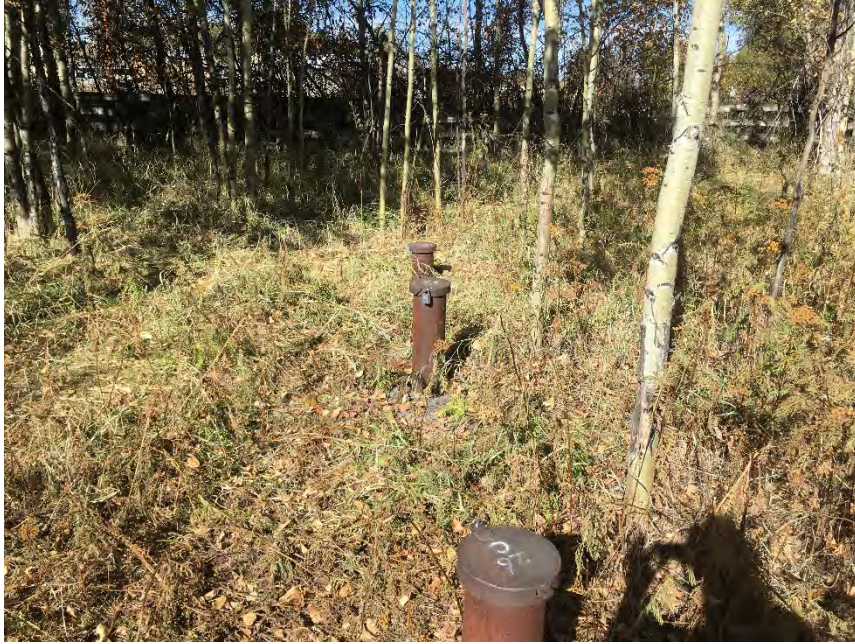
Monitoring wells 26A, B and C. No issues identified during the inspection.
