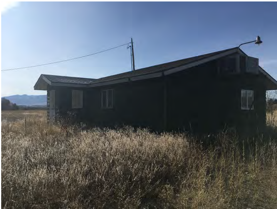
The Green administrative building. A trespasser broke into this building and turned up the heat. Electricity was turned off as a result of the trespasser and the building is going to be relocated to an adjacent property pending permit approval from the City of Bozeman.
