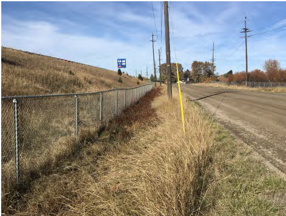
Bohart lane ditch looking west. Community member noticed a black ooze in Spring 2019 during unusually high groundwater levels. Soil samples were collected in October 2019 and analyzed for pentachlorophenol and total extractable hydrocarbons. Samples results are below screening levels for industrial use.
