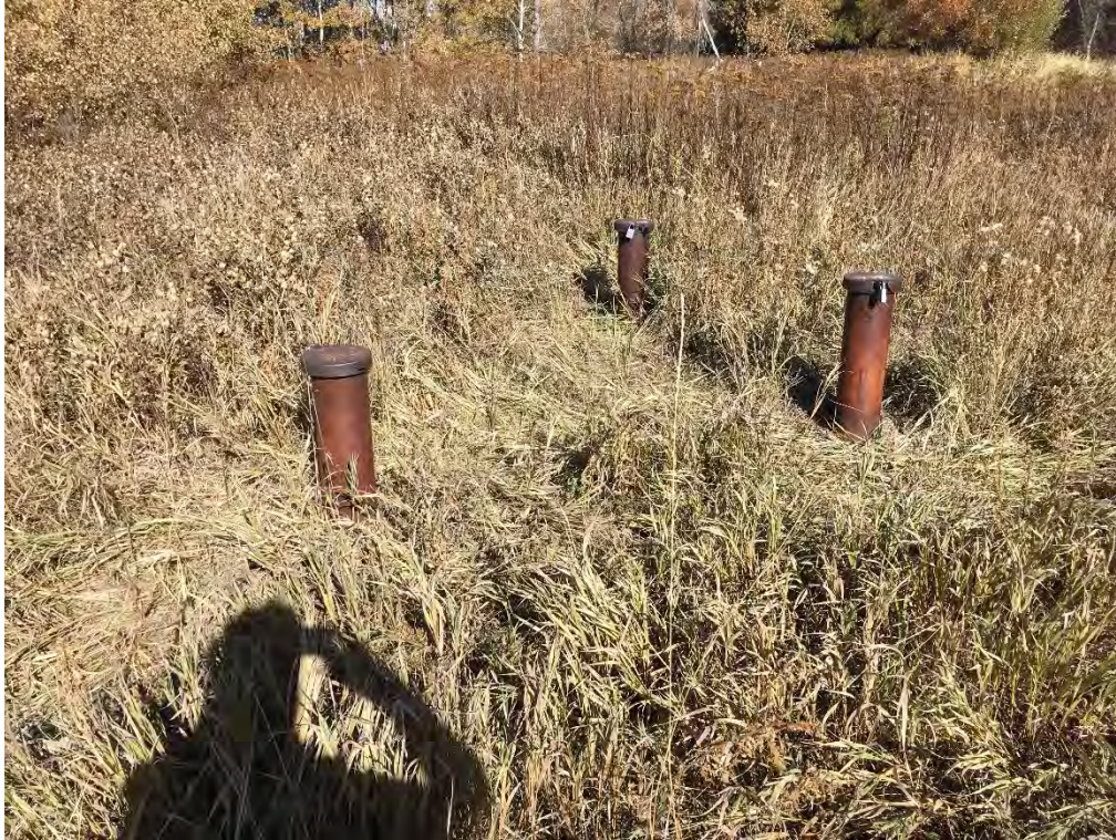
Wells 24A, B and C. No issues identified during the site inspection.
