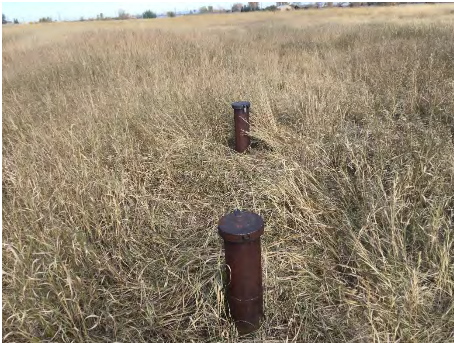
Wells 19A & B. No issues identified during the inspection.
