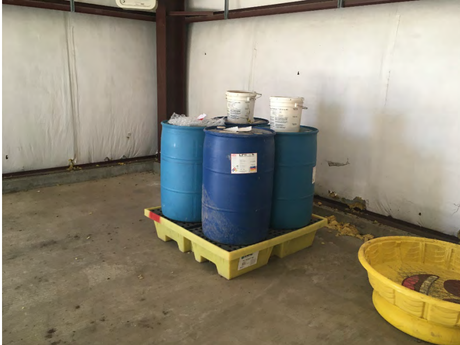
Treatment chemical remaining in the Groundwater Recovery System building after decommissioning of the WTP. Chemicals will be mixed with kitty litter to solidify and chemicals will be disposed in the local landfill.
