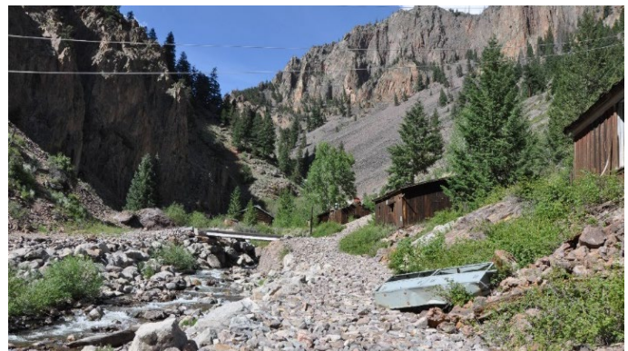
Cluster of buildings along West Willow Creek.
