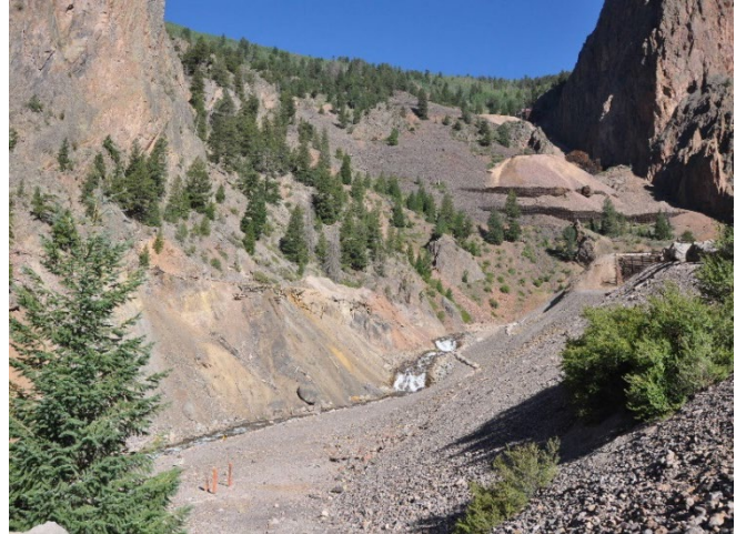
West Willow Creek downstream from Nelson Tunnel and Commodore Waste Rock Pile.
