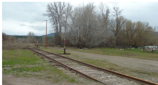
Rail to service businesses at the site.
