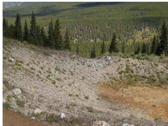
Retention pond at upper part of OU6 Evans Gulch Area (water line shows pond level is low even during spring runoff; pond capacity is much greater than the water line)
