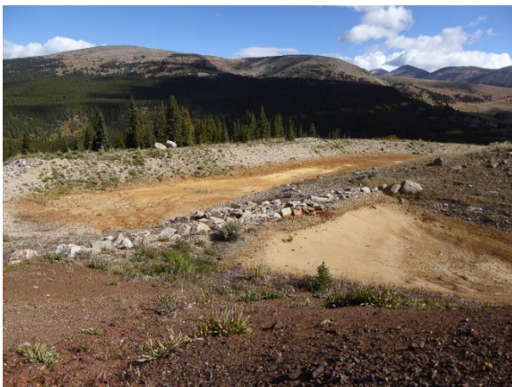
Retention pond at upper part of OU6 Evans Gulch Area (water line shows pond level is low even during spring runoff; pond capacity is much greater than the water line)
