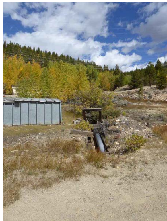
Outflow under road where new flow from OU6 goes through OU4 to California Gulch
