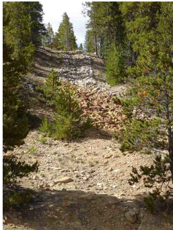
OU6 – reinforced Mikado Pond drainage ditch
