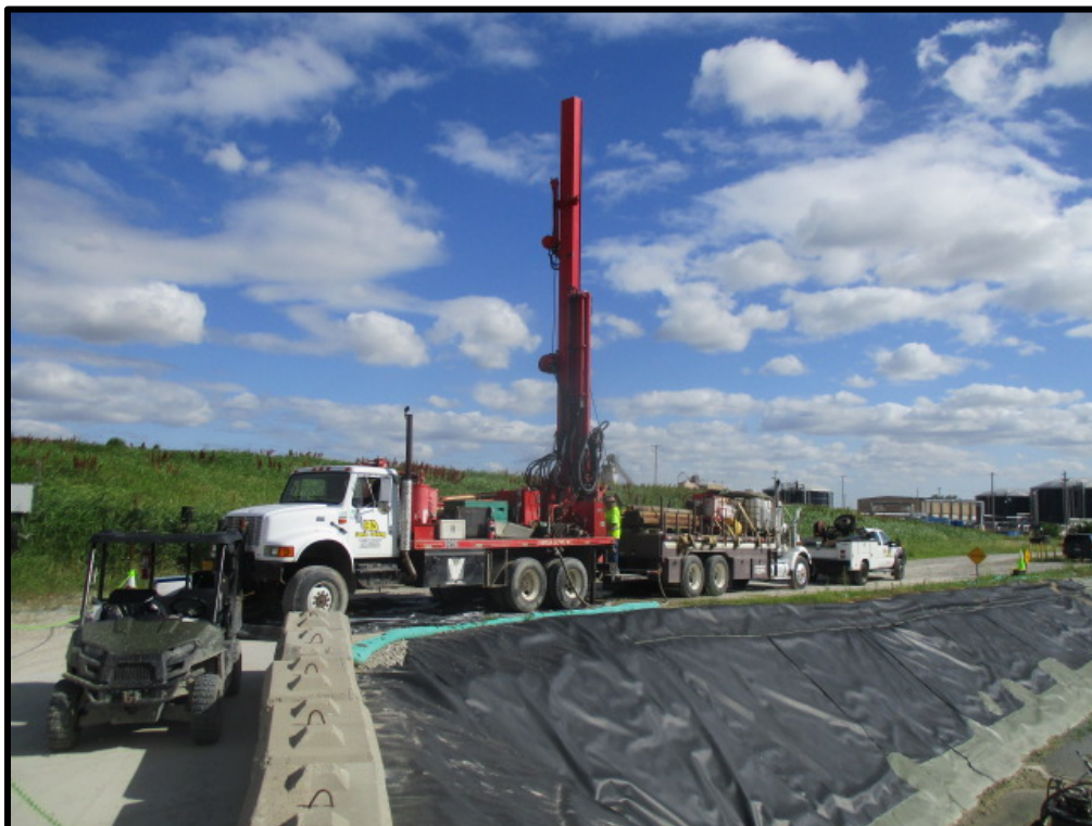
PHOTOGRAPH NO. 2 Borings were located as far east as possible, without impacting existing site infrastructure.
