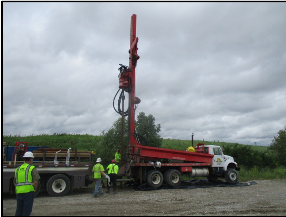
PHOTOGRAPH NO. 1 Sonic drill rig performing waste separation borings.
