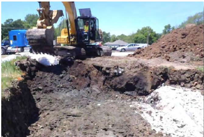
Excavation of site soils.
