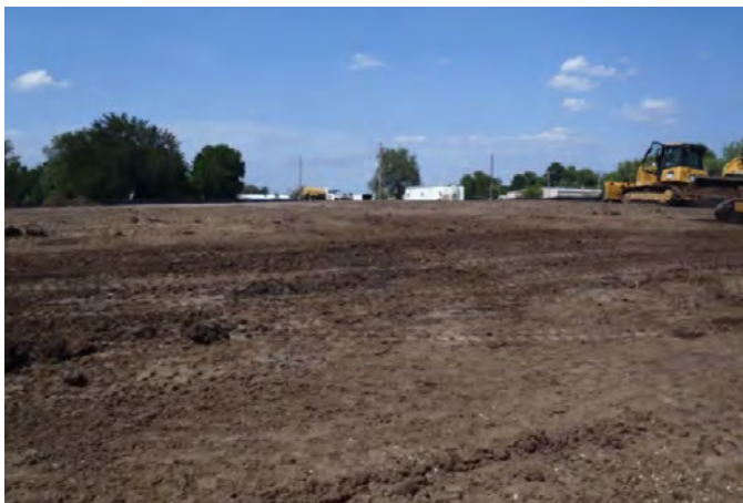
Final top soil grading.
