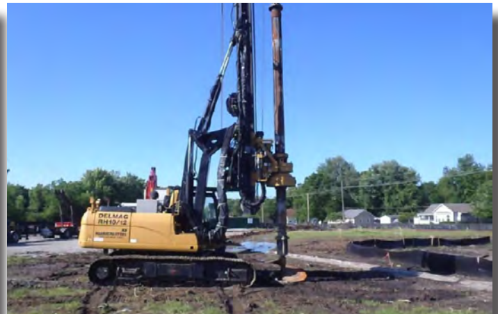
Equipment making large-diameter borings for monitoring.
